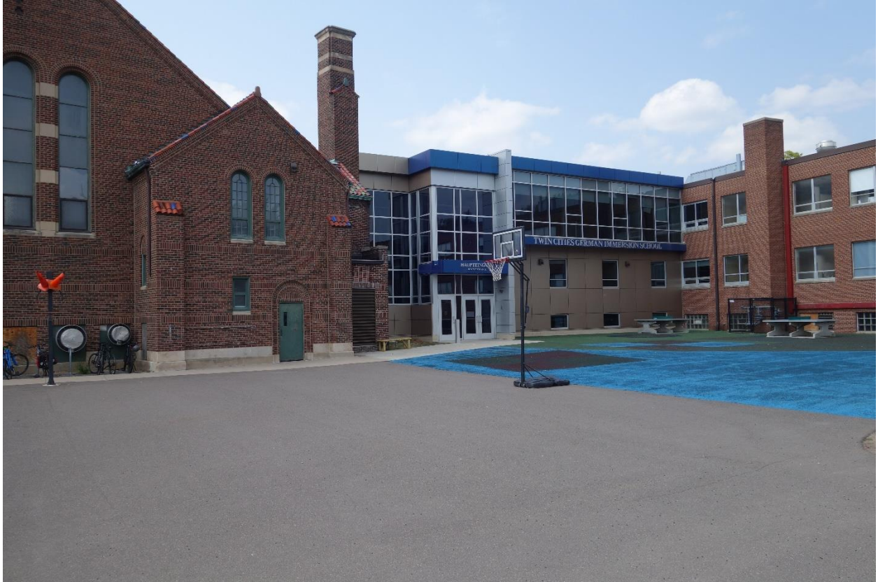
Figure 10. St. Andrew's Church at the left, the school building at the right, and the addition that connects the buildings in the center. Photo Rolf Anderson
