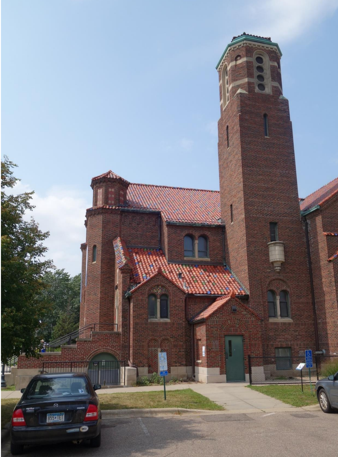
Figure 6. South portion of the east elevation. Photo Rolf Anderson
