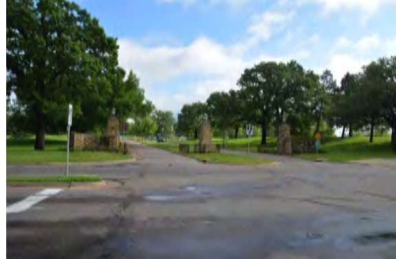
Figure 34. Wheelock Parkway facing Phalen Drive gates, facing east.
