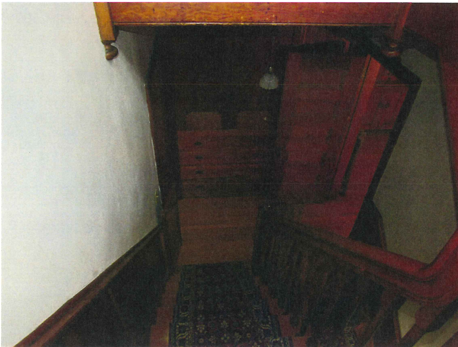
Stair Case from third floor
