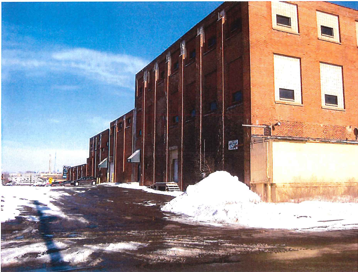
Looking north/northeast along Montgomery, subject site is the entire building and parking on right
