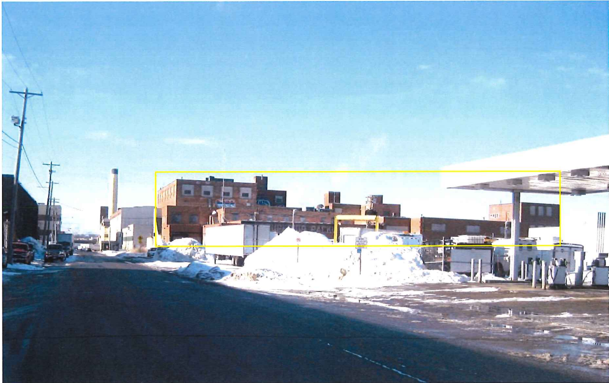
Looking west/northwest along Wabash, subject site is the brick building in yellow outline
