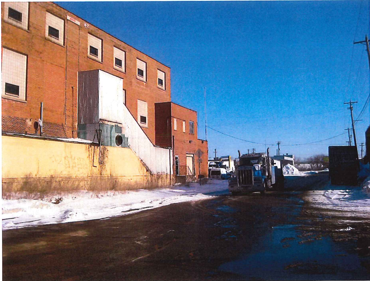
Looking east along Wabash, subject site on the left
