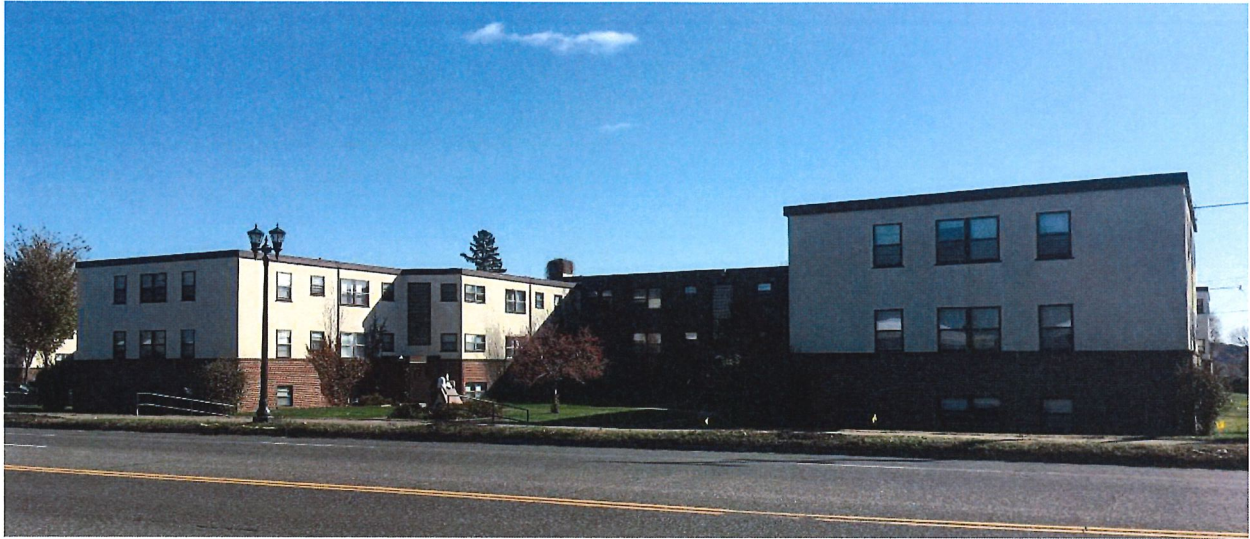
East of 2525 West 7th Street - Sibley Manor Apartments
