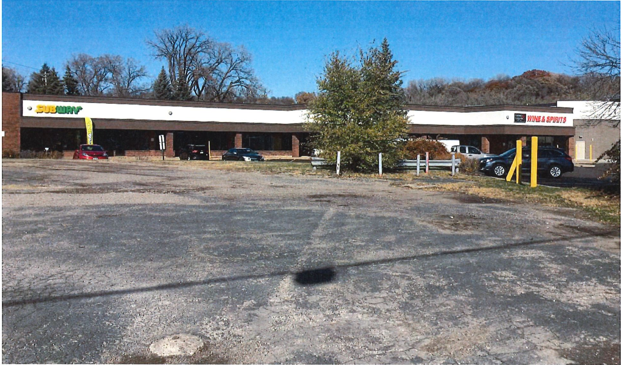
North end of 2525 West 7th Street and Sibley Plaza
