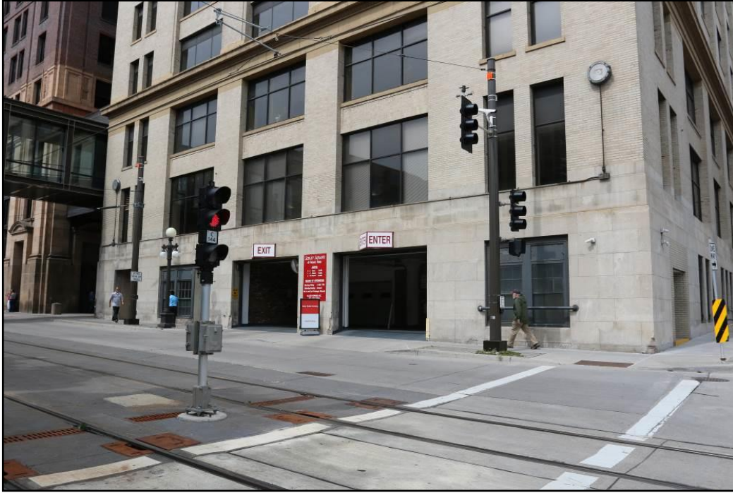
Pre-rehabilitation signage at the garage entrance overlooking East Fourth Street
