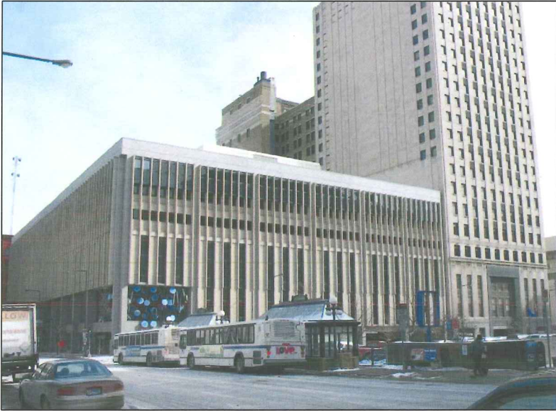
14. First Bank Addition, 332 Minnesota Street, left: 2008
