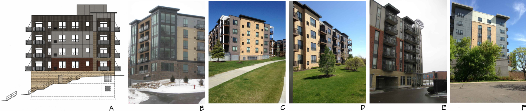
EXTERIOR FACADE IMAGERY
