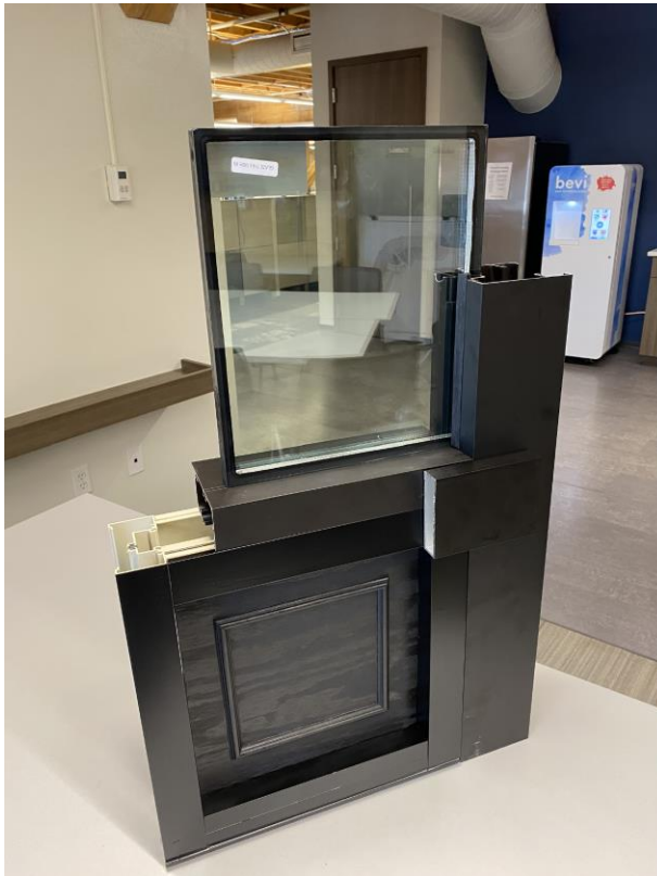
Figs. 10 & 11. Proposed mock-up of storefront. Entire system will be aluminum. Proposed section detail.
