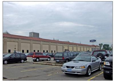
Window openings on the north facade of the main assembly building have been enclosed with concrete block.
