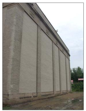
The window openings on the west facade of the steam plant were enclosed following flooding in the 1950s.
