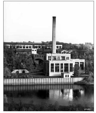
An enclosed bridge connected the steam plant to an underground conveyor that carried coal from the east side of the assembly plant. The tunnel entrance and barge dock are also shown in this 1936 photograph. (Minnesota Historical Society)
