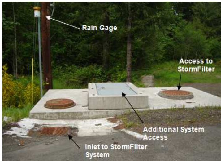
Figure 7. External view of the StormFilter system at Lolo Pass Road.
