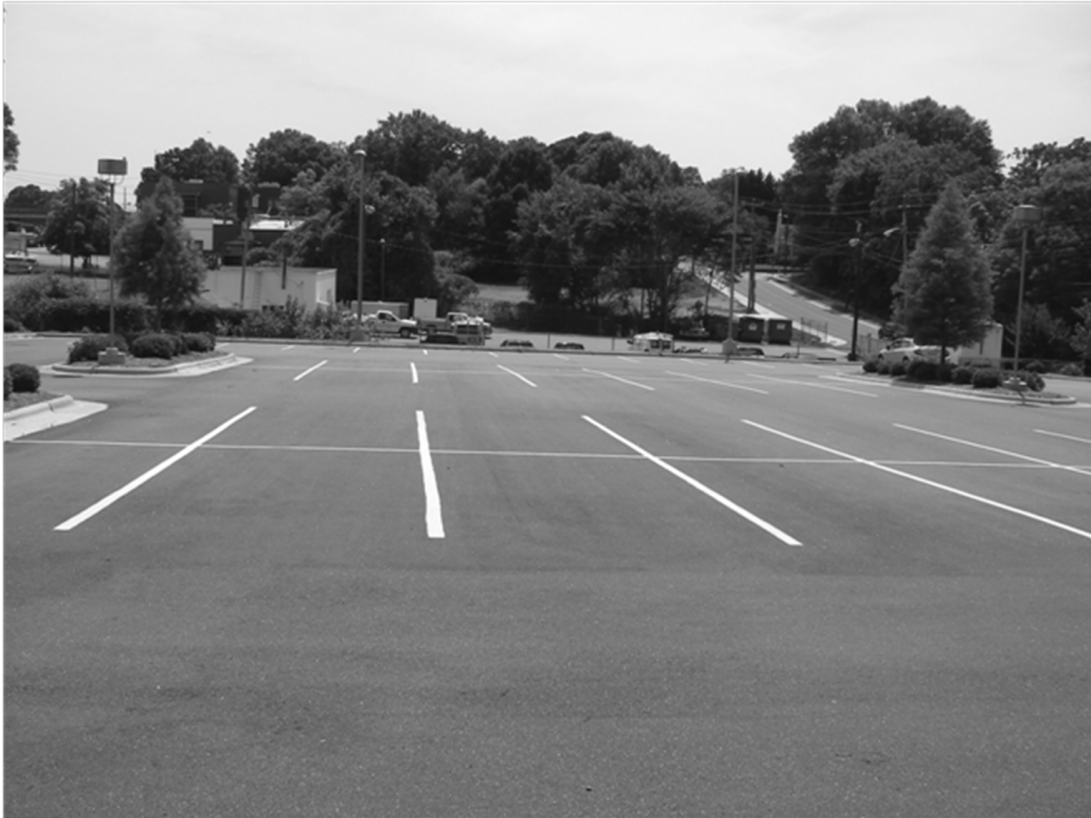
Figure 2. View of finished parking lot at the Mitchell Community College testing site.
