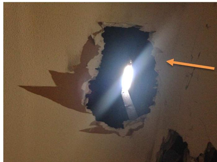
**Picture 6 – Hole Through Ceiling and Roof**
