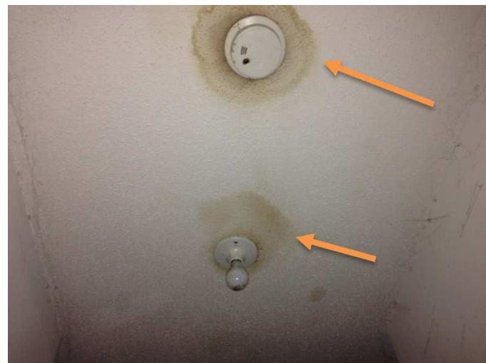
**Picture 4 – Water Damage at 2<sup>nd</sup> Floor Ceiling**
