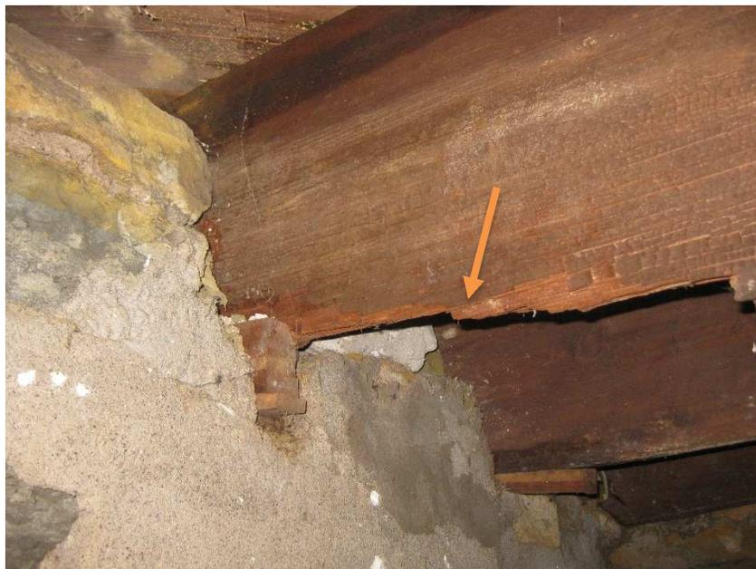
**Picture 8 – Damaged Floor Joist**
