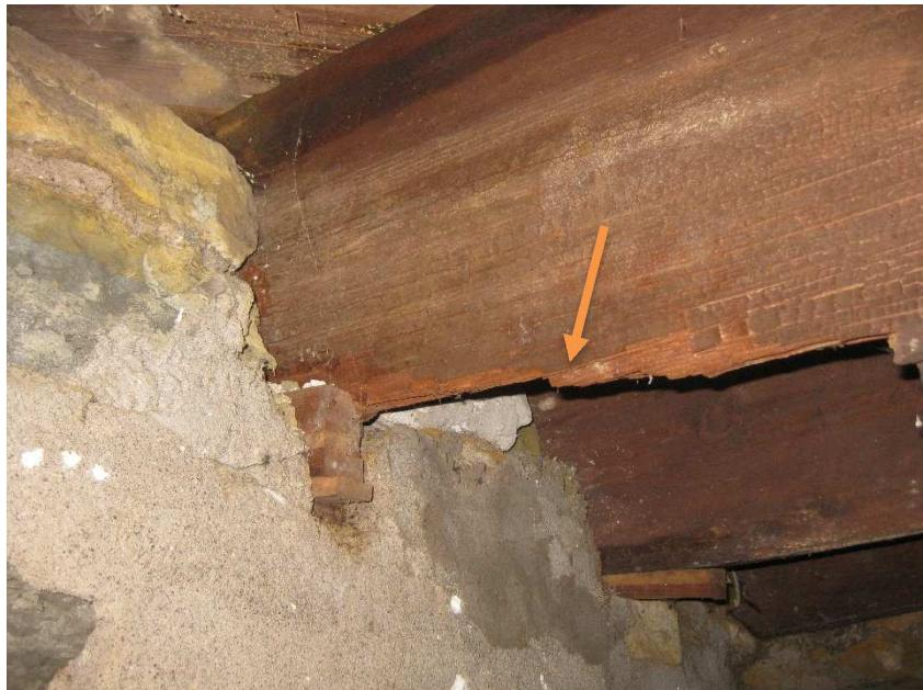
**Picture 8 – Damaged Floor Joist**
