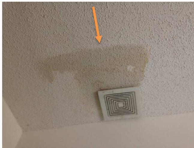
**Picture 5 – Water Damage at 2<sup>nd</sup> Floor Ceiling**
