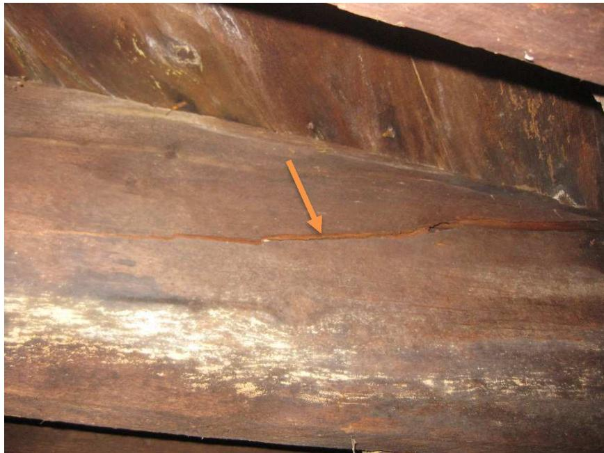
**Picture 7 – Crack in Floor Joist**
