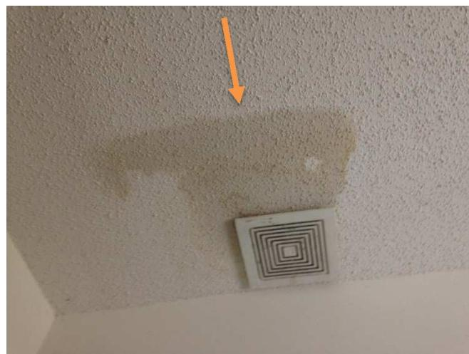
**Picture 5 – Water Damage at 2<sup>nd</sup> Floor Ceiling**
