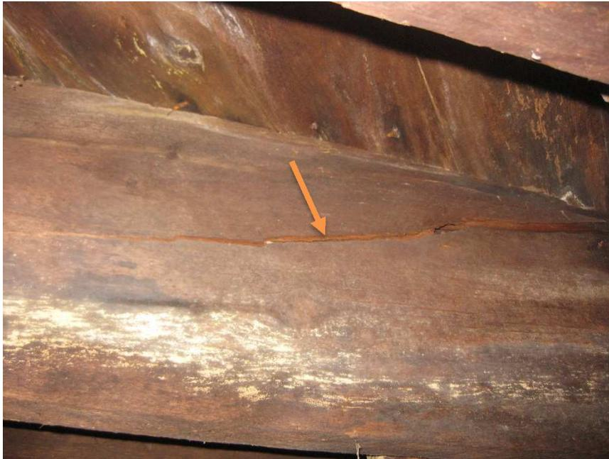
**Picture 7 – Crack in Floor Joist**
