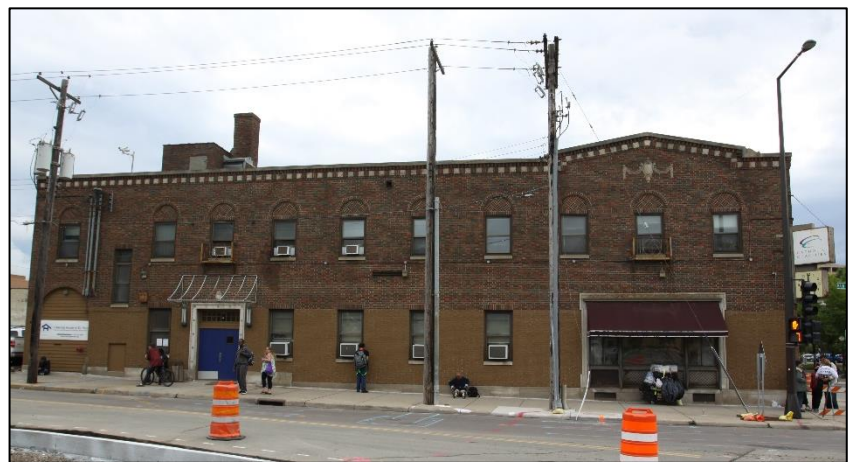
The west wall, looking east
