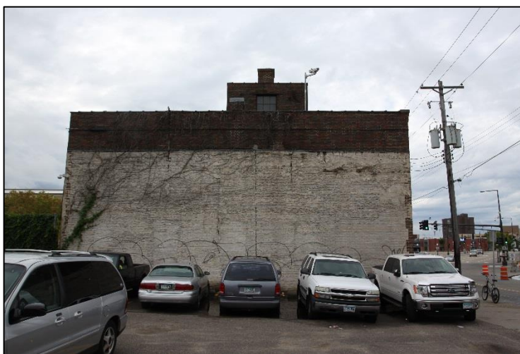
The north wall, looking south; the painted section was originally concealed by an adjacent building
