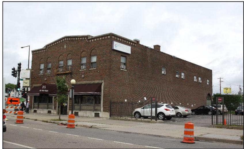
The south (left) and east (walls), looking northwest
