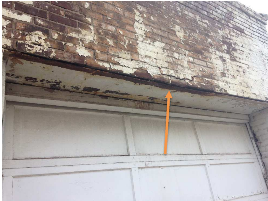
Picture 5 – Deflecting Lintel at Northwest Wall
