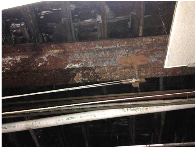
Picture 3 – Rusting Steel Beam
