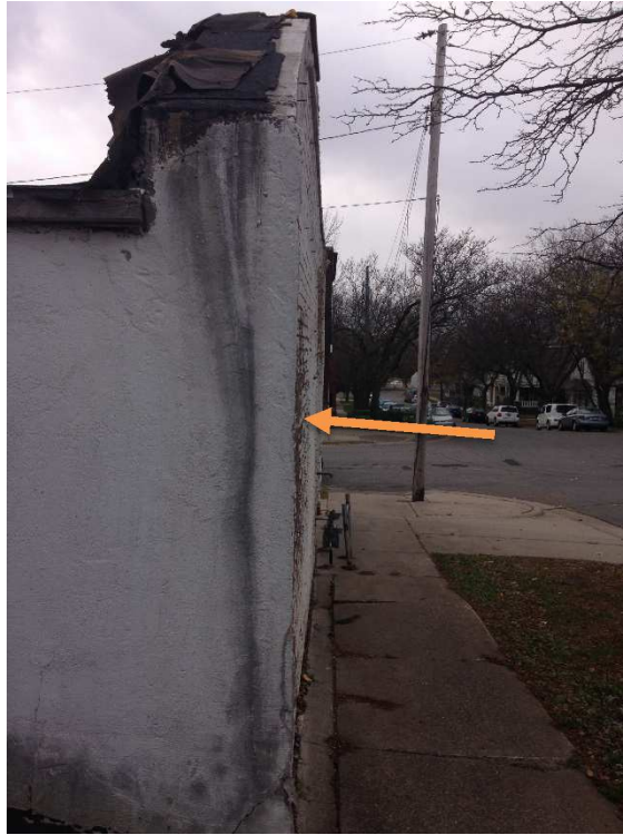
Picture 7 – Northeast Wall
