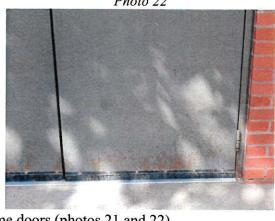
Corrosion was observed on the hollow metal frame doors (photos 21 and 22).
