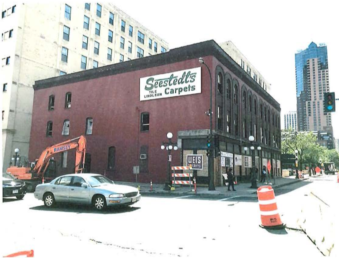
E.01 Looking south from Wall Street at the north and east façades. Photo taken August 2019.
