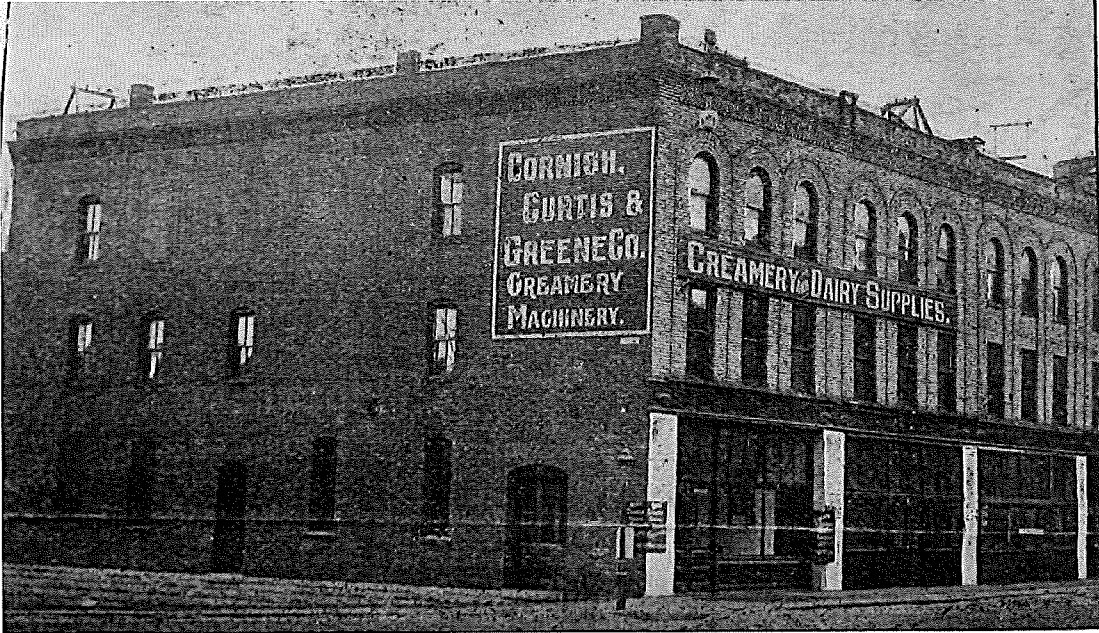
H.01 Looking south from Wall Street at the north and east façades. Photo taken 1898. Photo Courtesy of the Minnesota Historical Society archives ("The Quotation," Vol, 1 No. 39, 1898).
