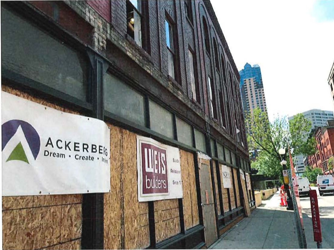
E.03 Looking southwest from East 6th Street at the north façade. Photo taken August 2019.
