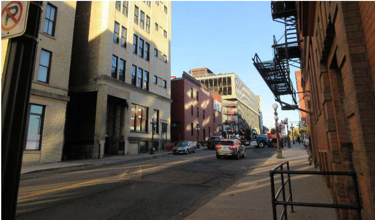
Figure 4: View of the Commission House, looking northwest from the intersection of Wall Street and 5 th Street East. Mock up rooftop addition minimally visible.
