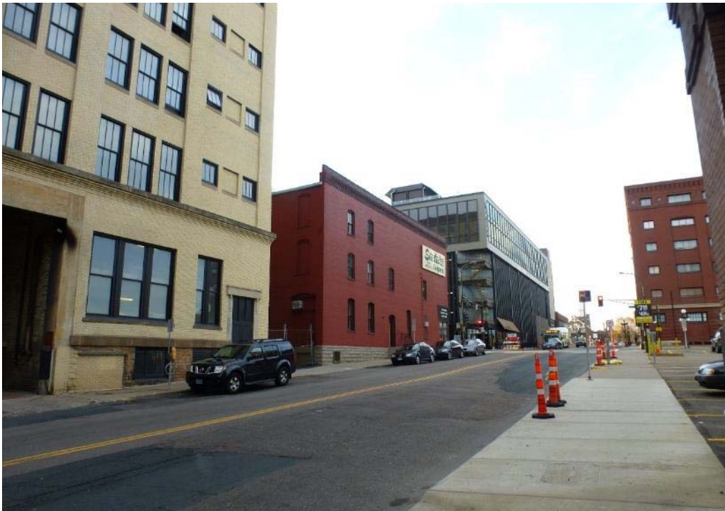
E.04 View of the east elevation, looking north. October 2015.
