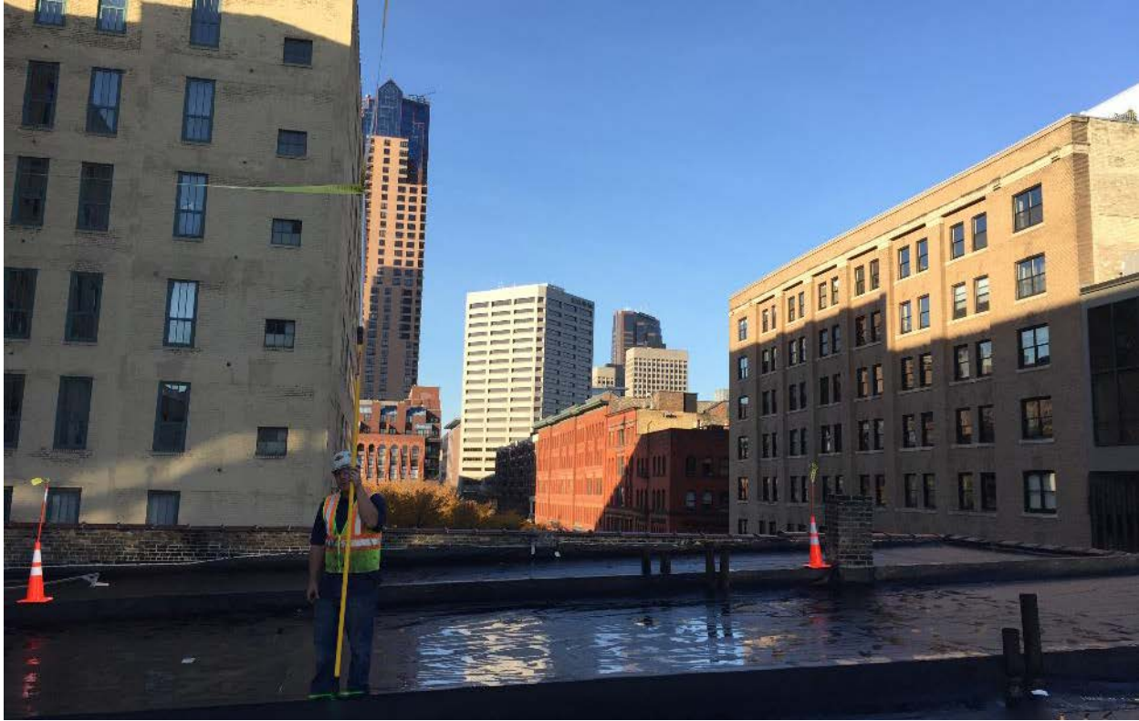
Figure 3: View of rooftop addition mock up, looking west. Photo courtesy of Crowe Construction.
