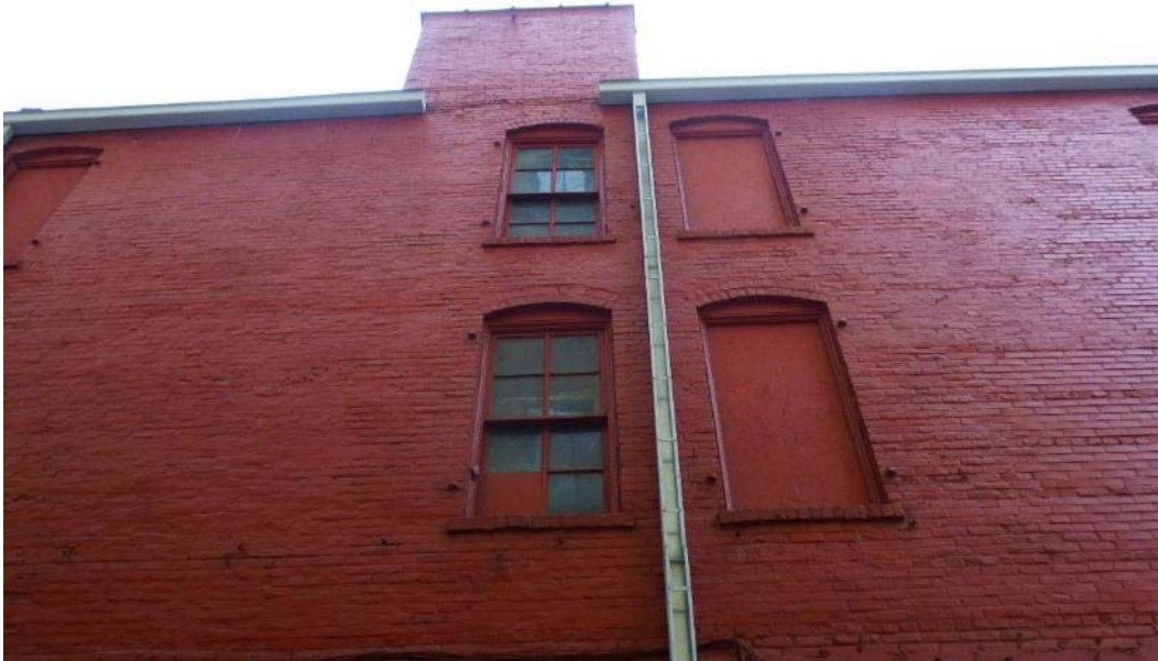
E.13 View of south elevation remaining wood windows and infilled window openings, elevator overrun, and drainage system, looking north. October 2015.
