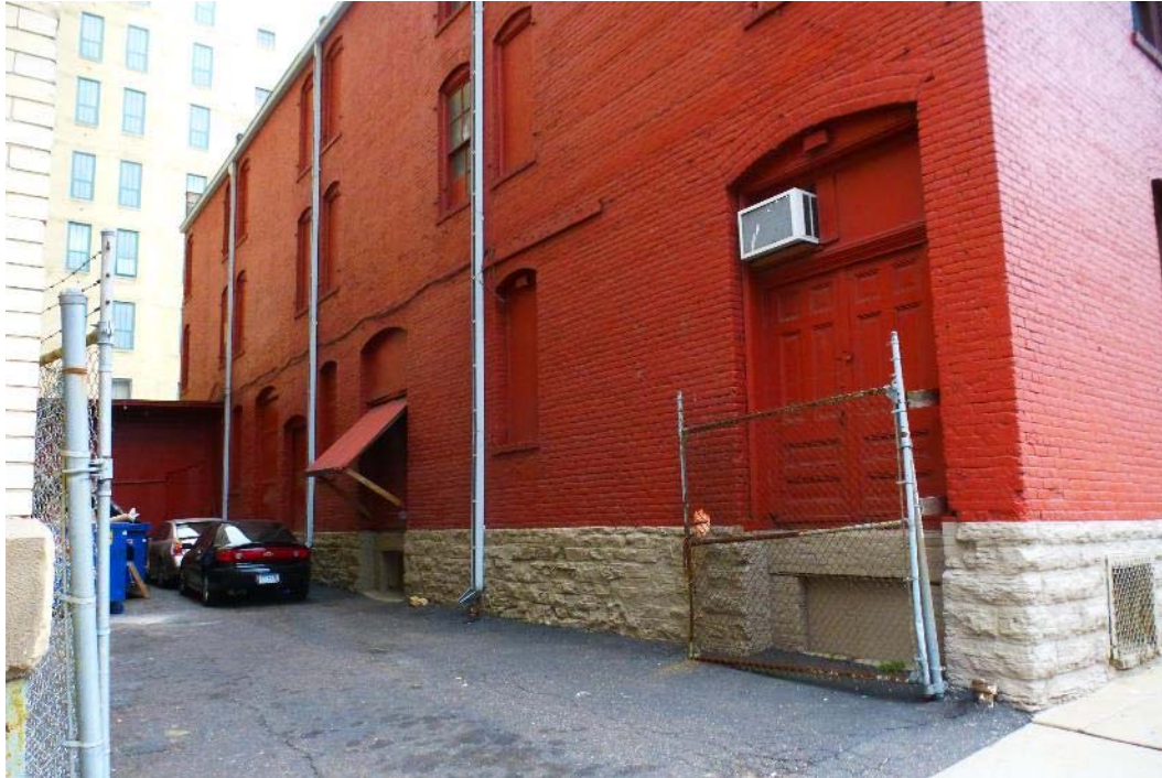
E.07 View of south elevation, looking northwest. Note the limestone foundation, and loading dock with historic wood double leaf panel doors. October 2015.
