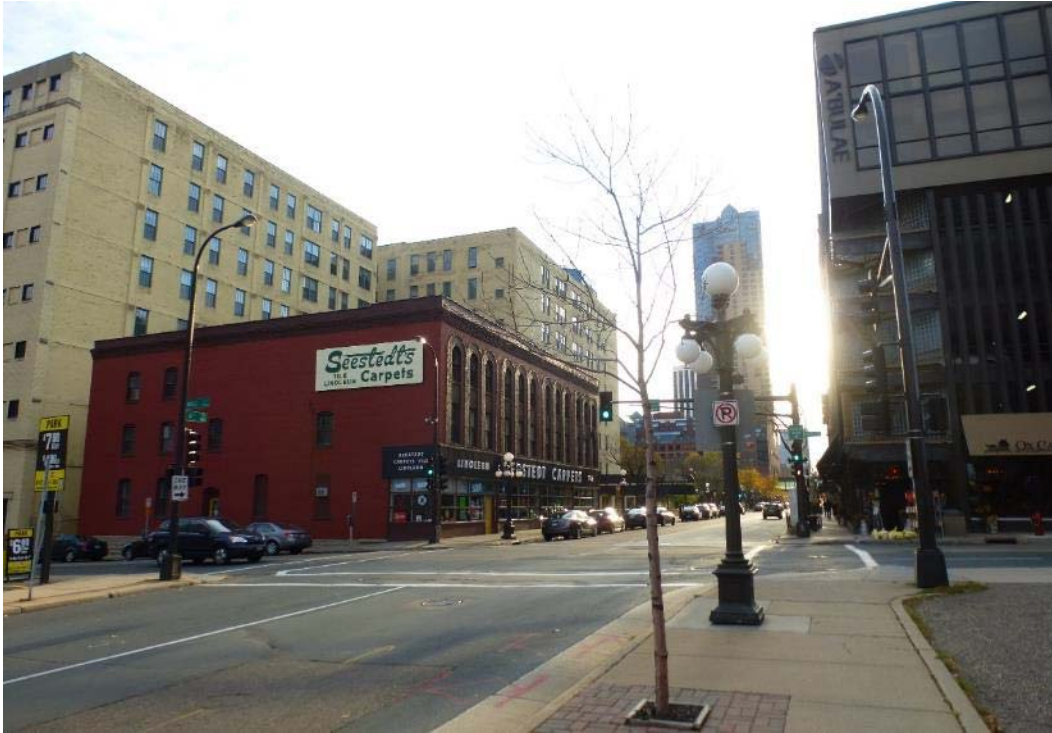
E.03 View of the east and north elevations, looking west. October 2015.
