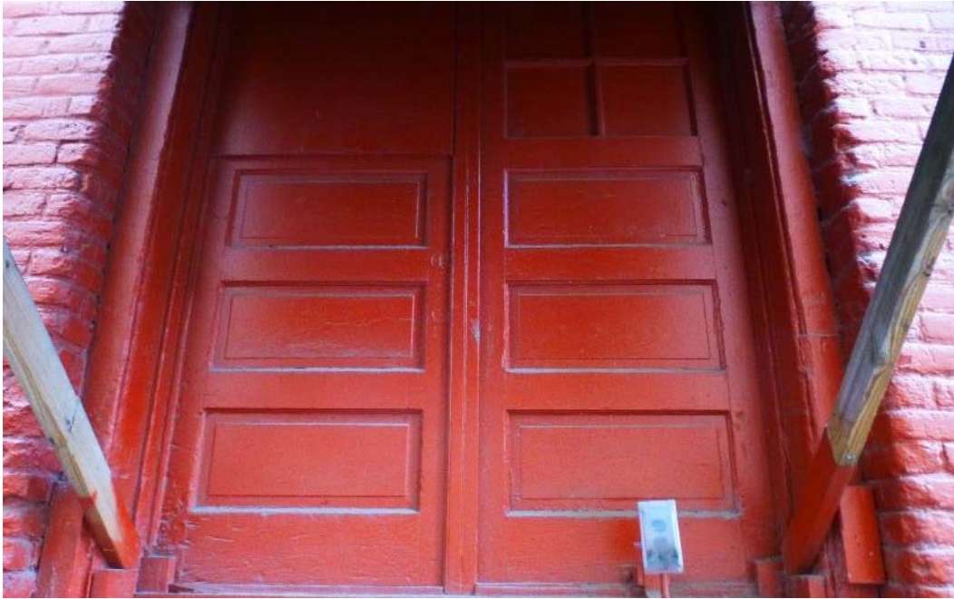
E.11 View of remaining south elevation, historic loading dock doors, looking north. October 2015.
