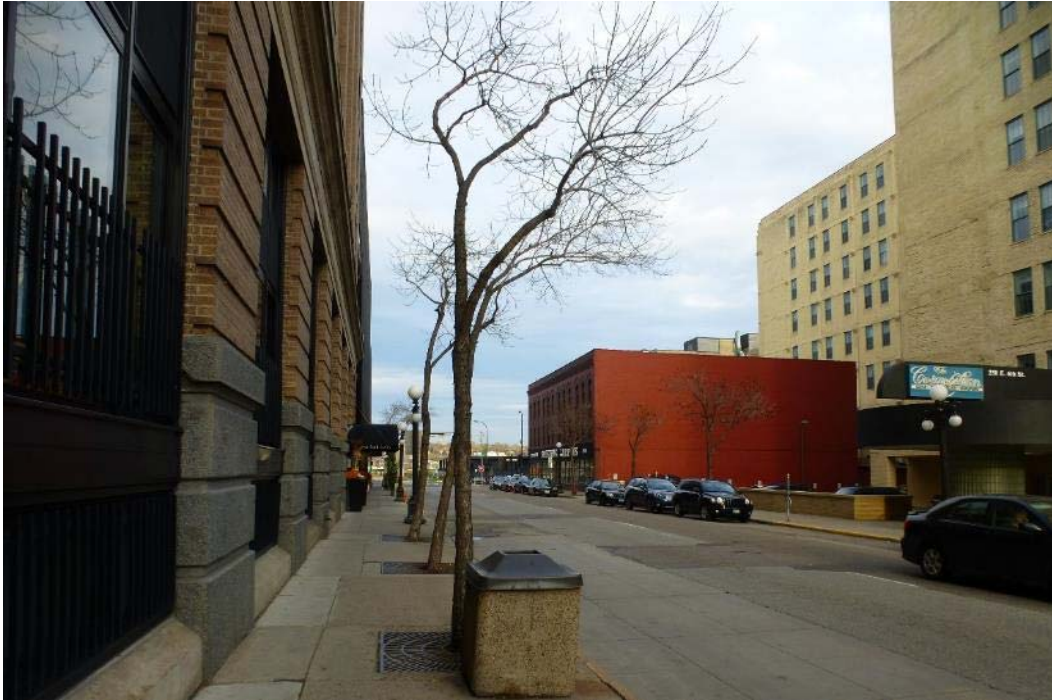
E.01 View of the west 1 elevation, looking east. October 2015.
