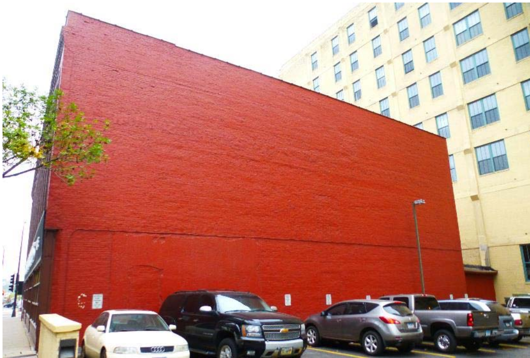
E.08 View of west elevation, looking east. October 2015.
