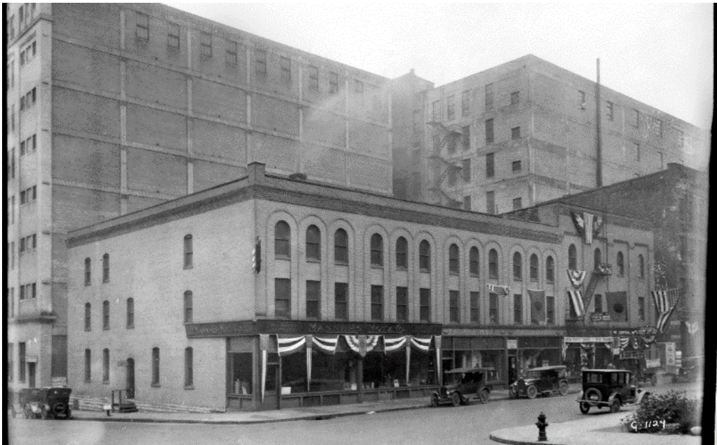
H.02 Manners and Motz Building looking southwest. 1924. Photo Courtesy of the Minnesota Historical Society archives (1542-B).
