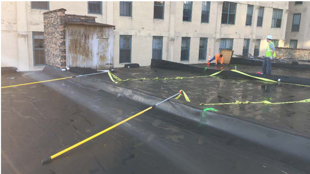
Figure 2: View of roof top addition mock up during its assembly, looking southwest. Photo courtesy of Crowe Construction.
