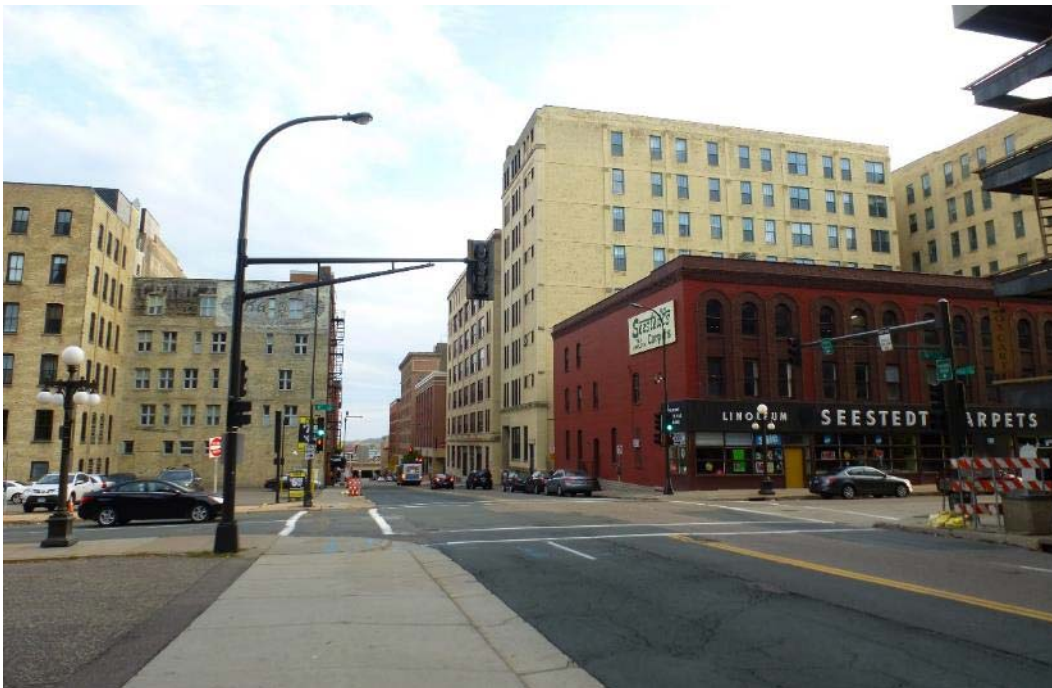
E.02 View of the north corner of the building, looking south. October 2015.
