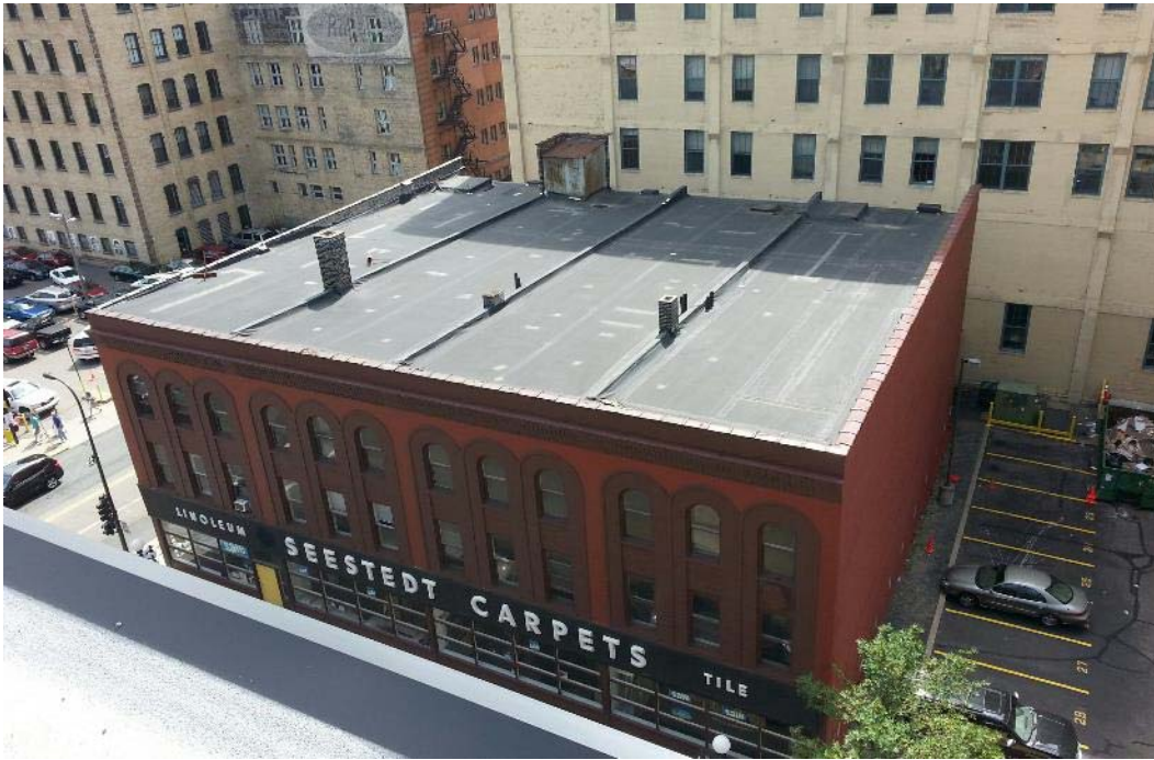
E.15 View of the roof from across the street, looking true east. Summer 2015. Photo courtesy of Global Resource Developers, Inc.
