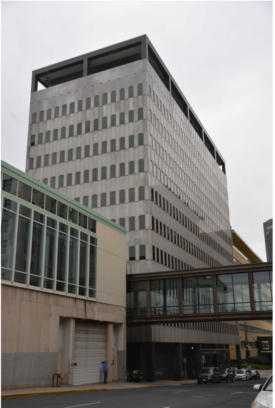
Degree of Honor Protective Association Building_0003 Exterior, South and West elevations, camera facing Northwest.
