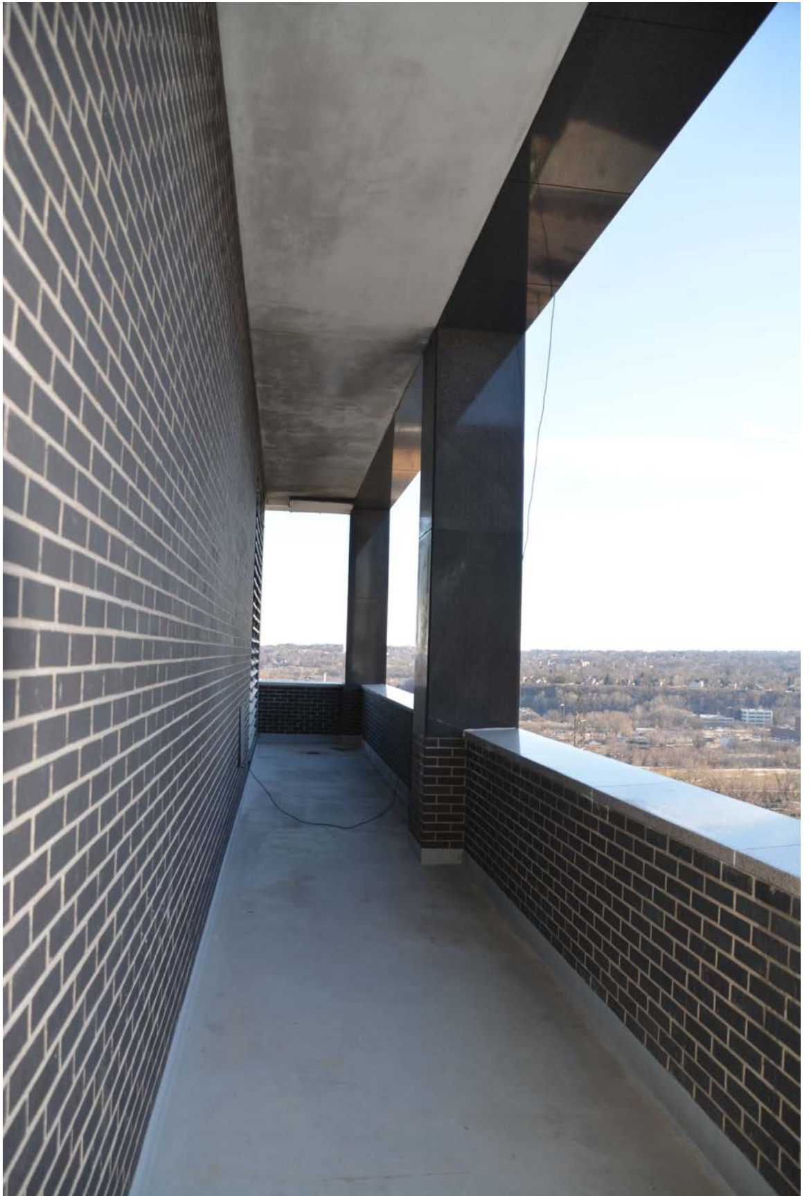
Degree of Honor Protective Association Building_0011 Exterior, Eleventh floor, mechanical floor, camera facing South.
