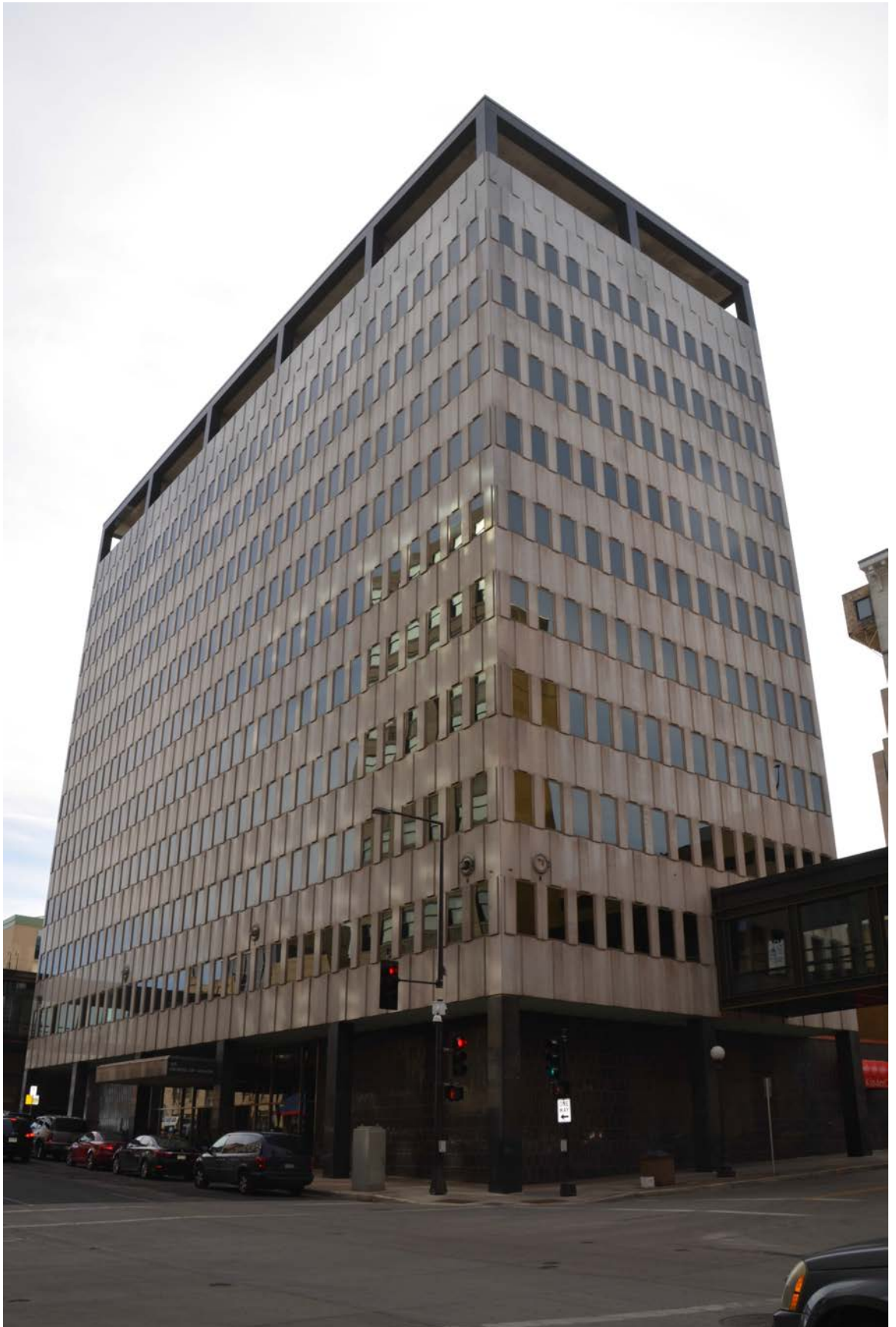
Degree of Honor Protective Association Building_0001 Exterior, North and East elevations, camera facing Southwest.
