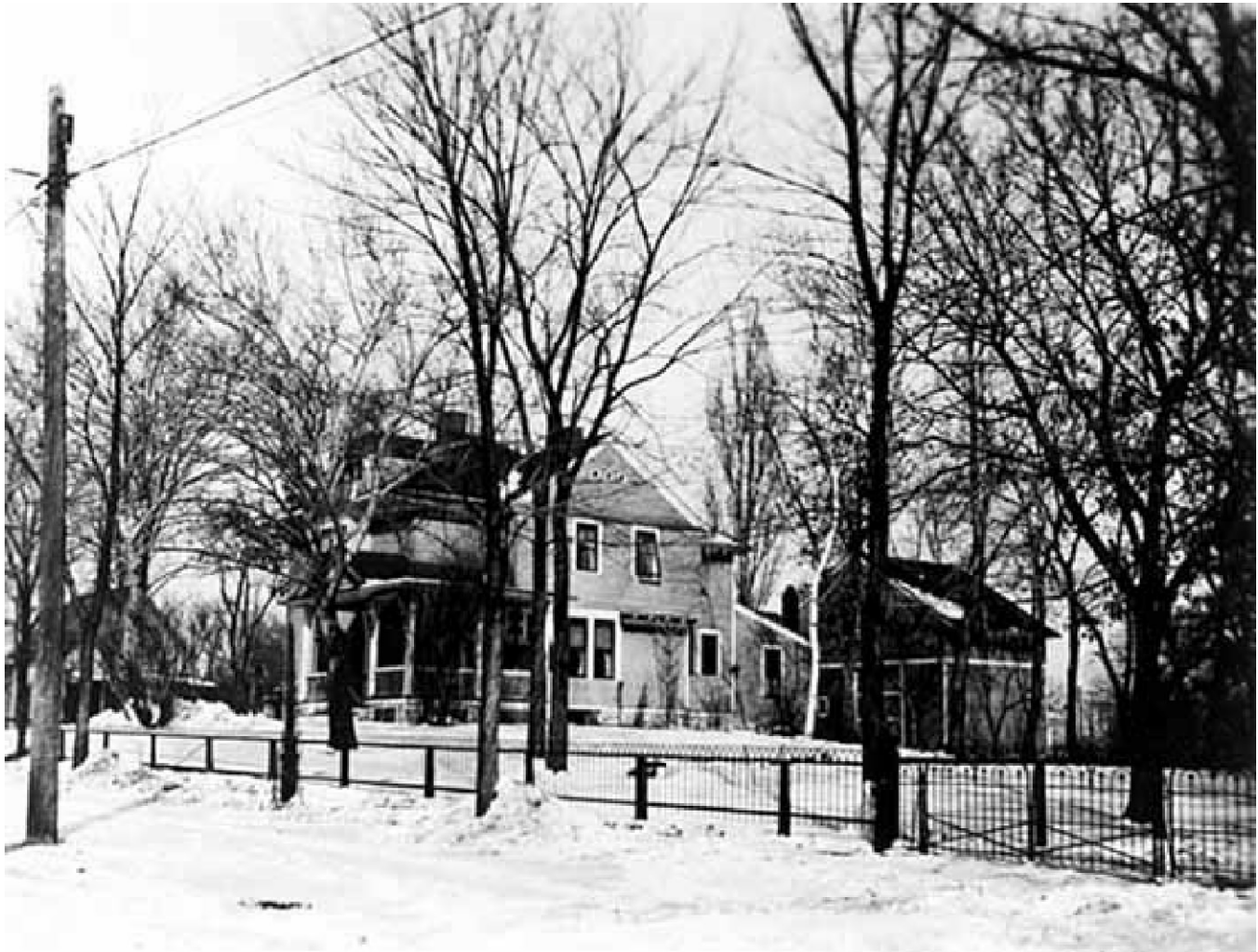
Fig 10. Dwight and Clara Watson House and Barn from the southwest, 1914 source: Mark Thomas
