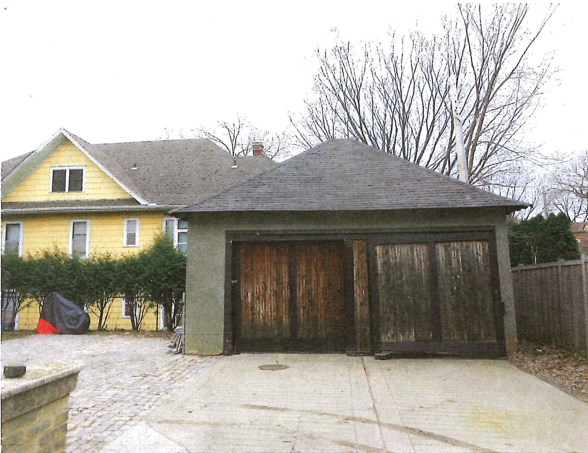
North elevation of existing garage
