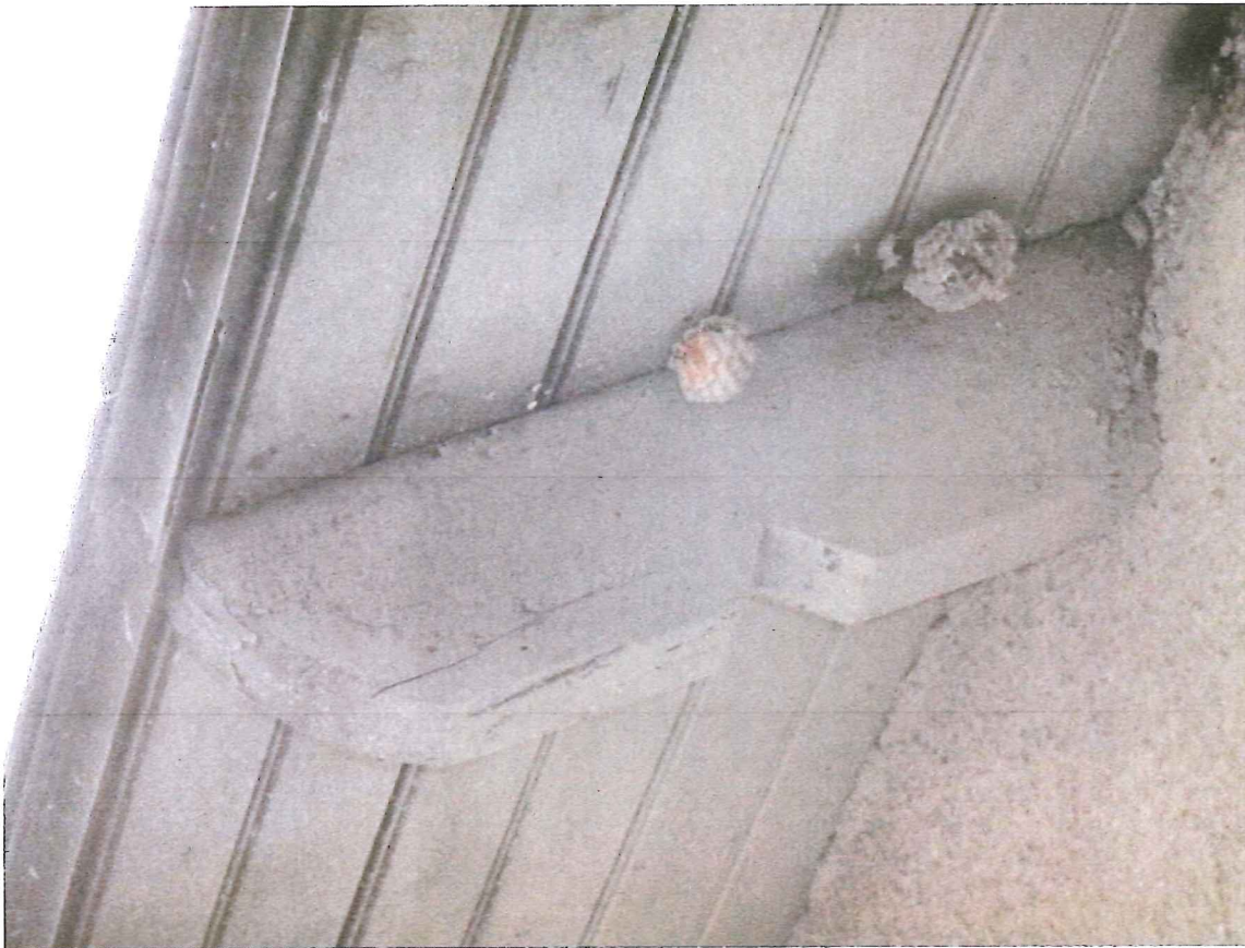
Rafter tails and beaded soffit
