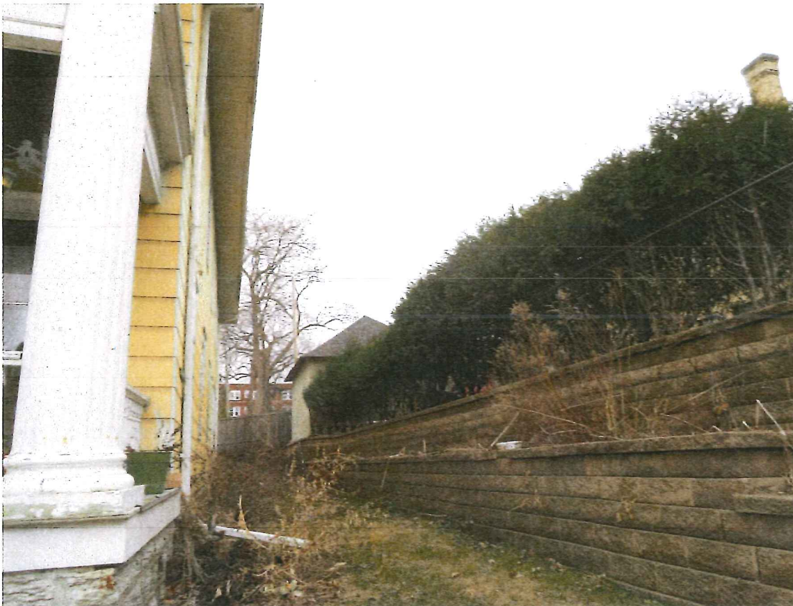
SE corner from sidewalk (Oakland Ave)
