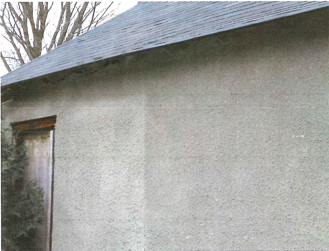
East wall of existing
