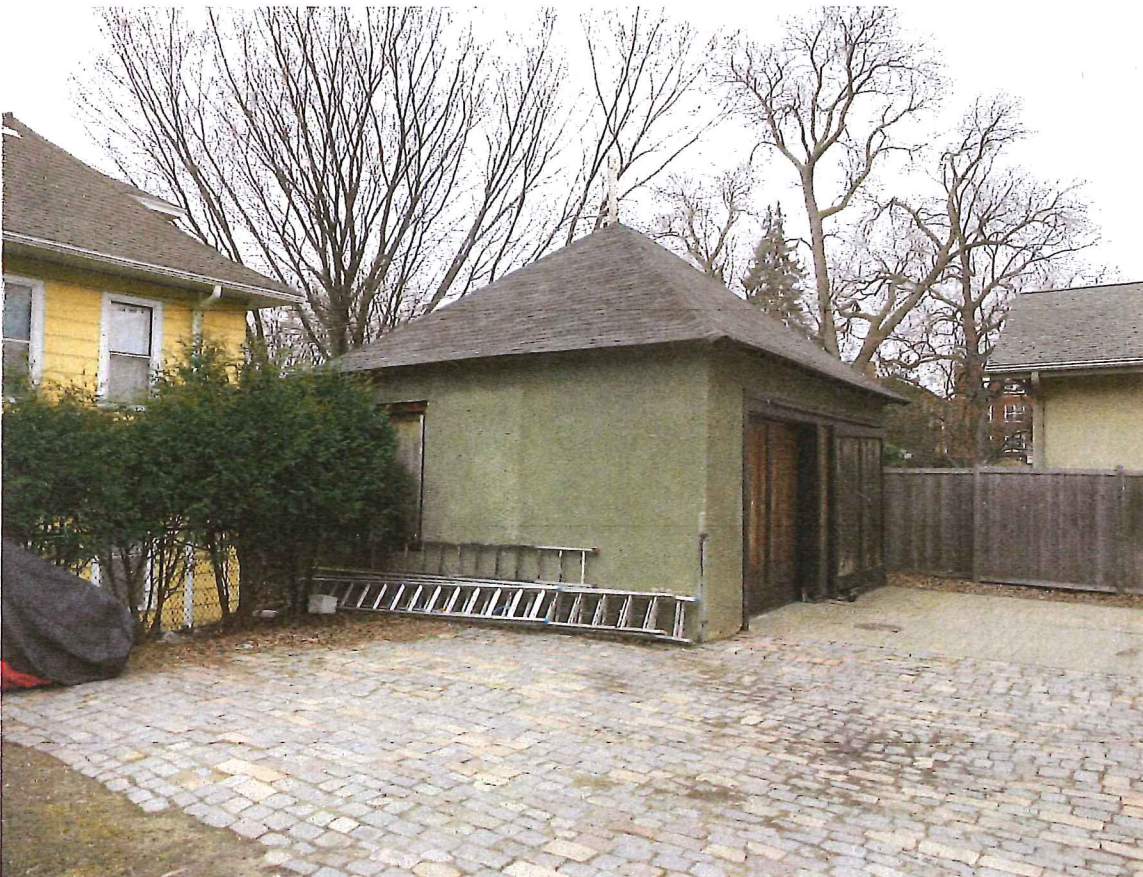
Northeast corner of existing garage
