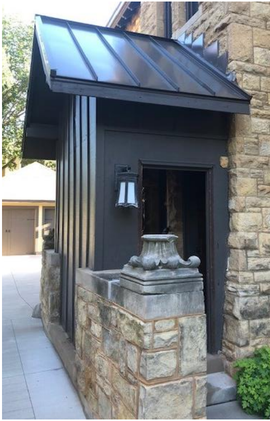
Existing side porch
