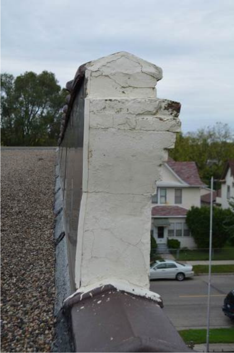
Photograph 5. Parapet of original portion of building. Photograph shows the addition of a parapet cap to match the detailing of the 1911 addition.
