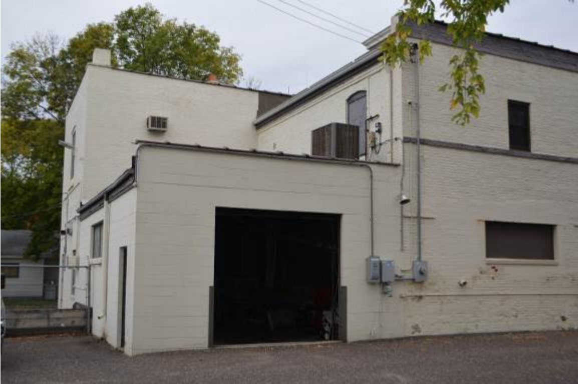
Photograph 4. East side of 1953 addition, taken from the parking lot. Camera facing northwest.
