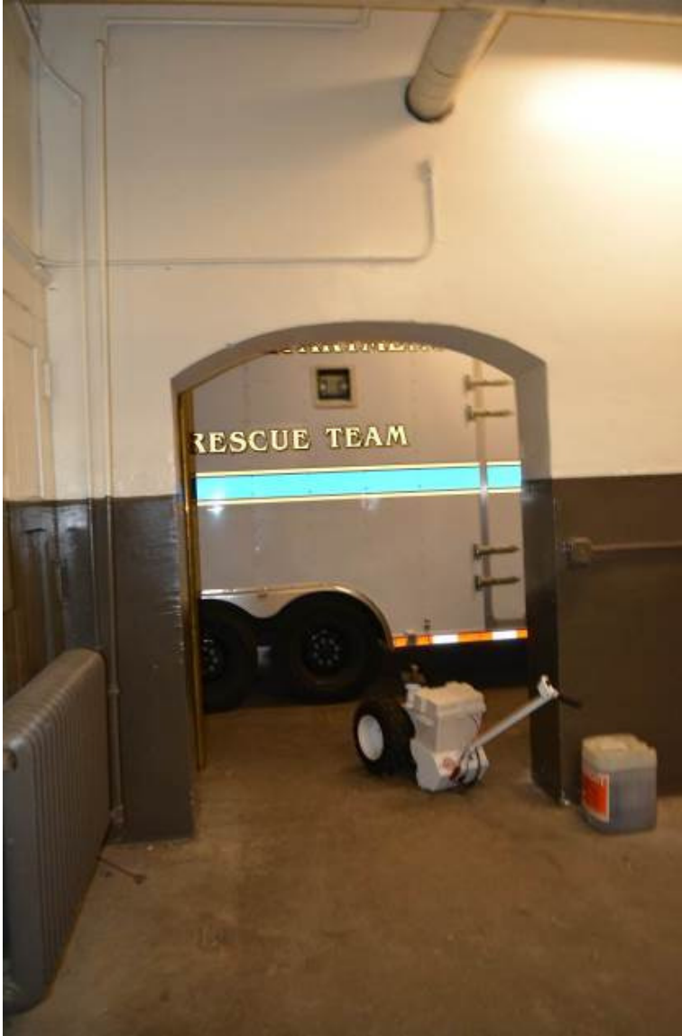
Photograph 10. Brick arch passage between 1885 building and 1911 addition, camera facing west. Photograph taken from 1885 apparatus bay.
