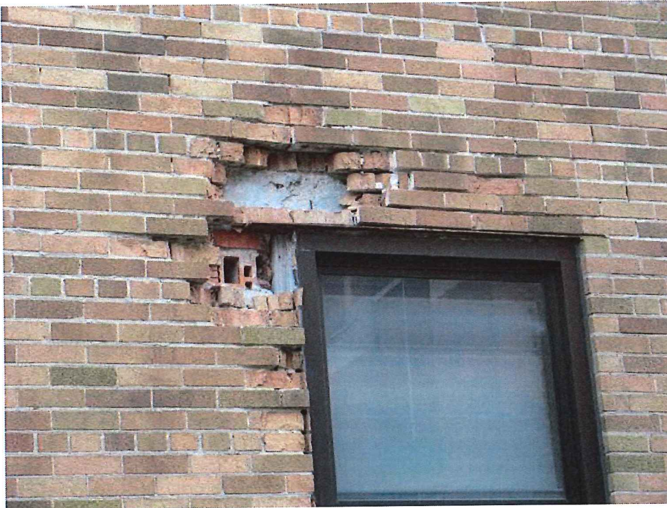
E.09 Photo of missing and damaged masonry units on southeast façade. Photo taken October 2017.
