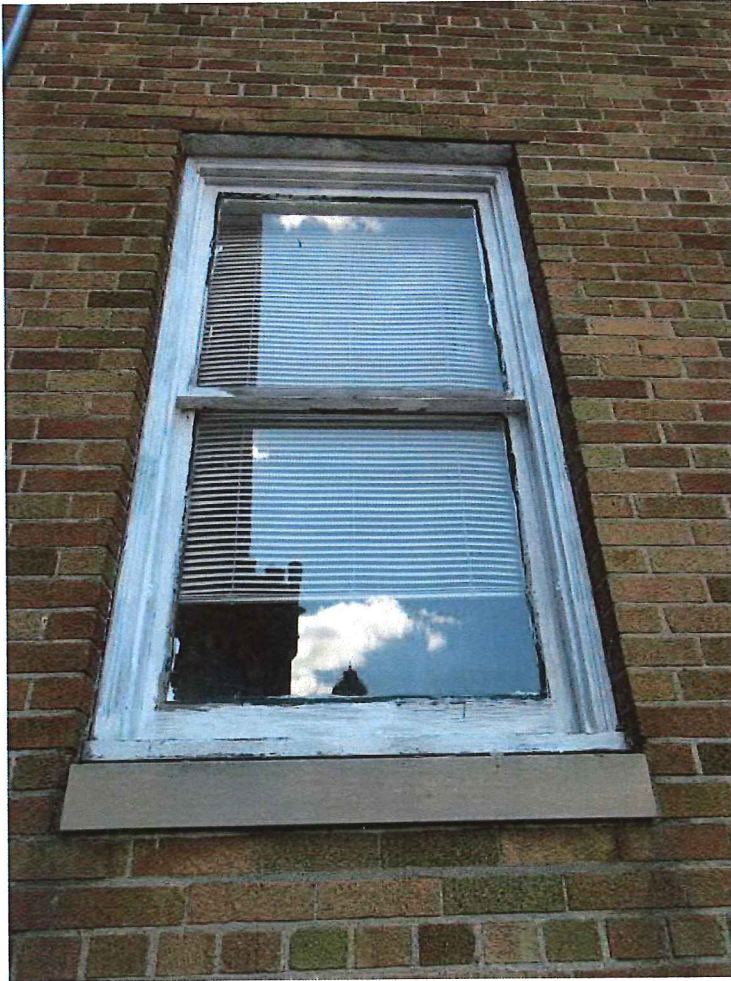
E.19 Detail of the condition of original wood window on southeast façade. Photo taken October 2017.
