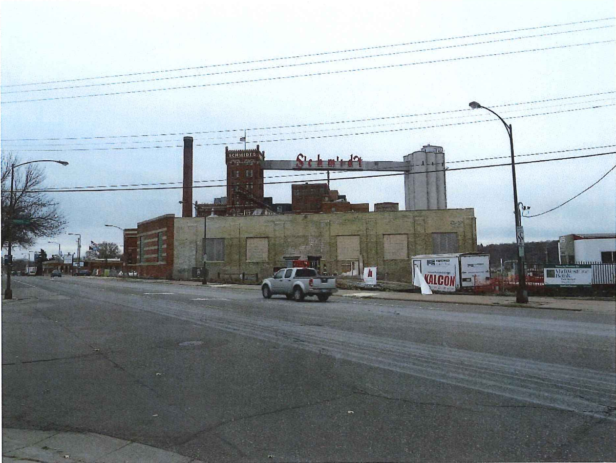
Photo 4. West and northwest elevations of building, December 2017.
