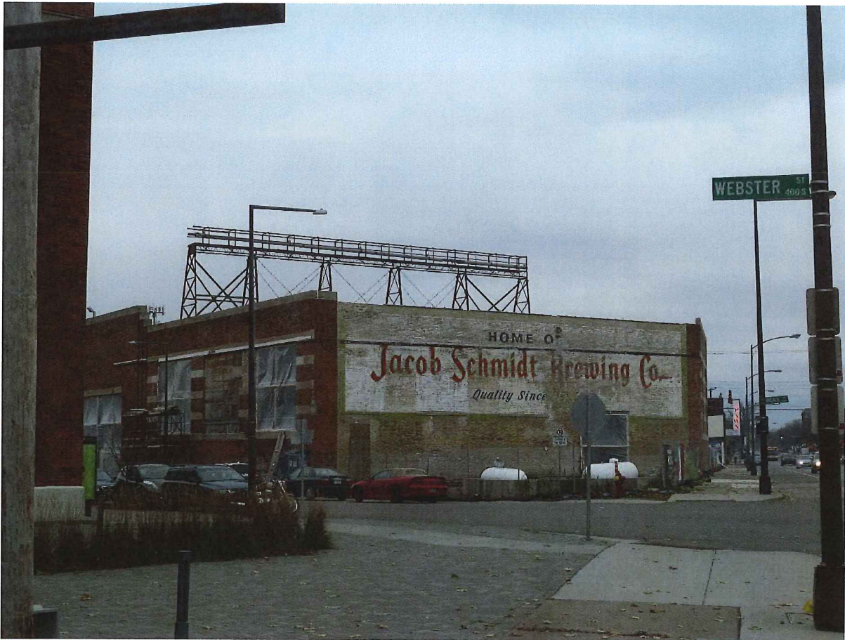
Photo 10. North and east elevations of building, December 2017.
