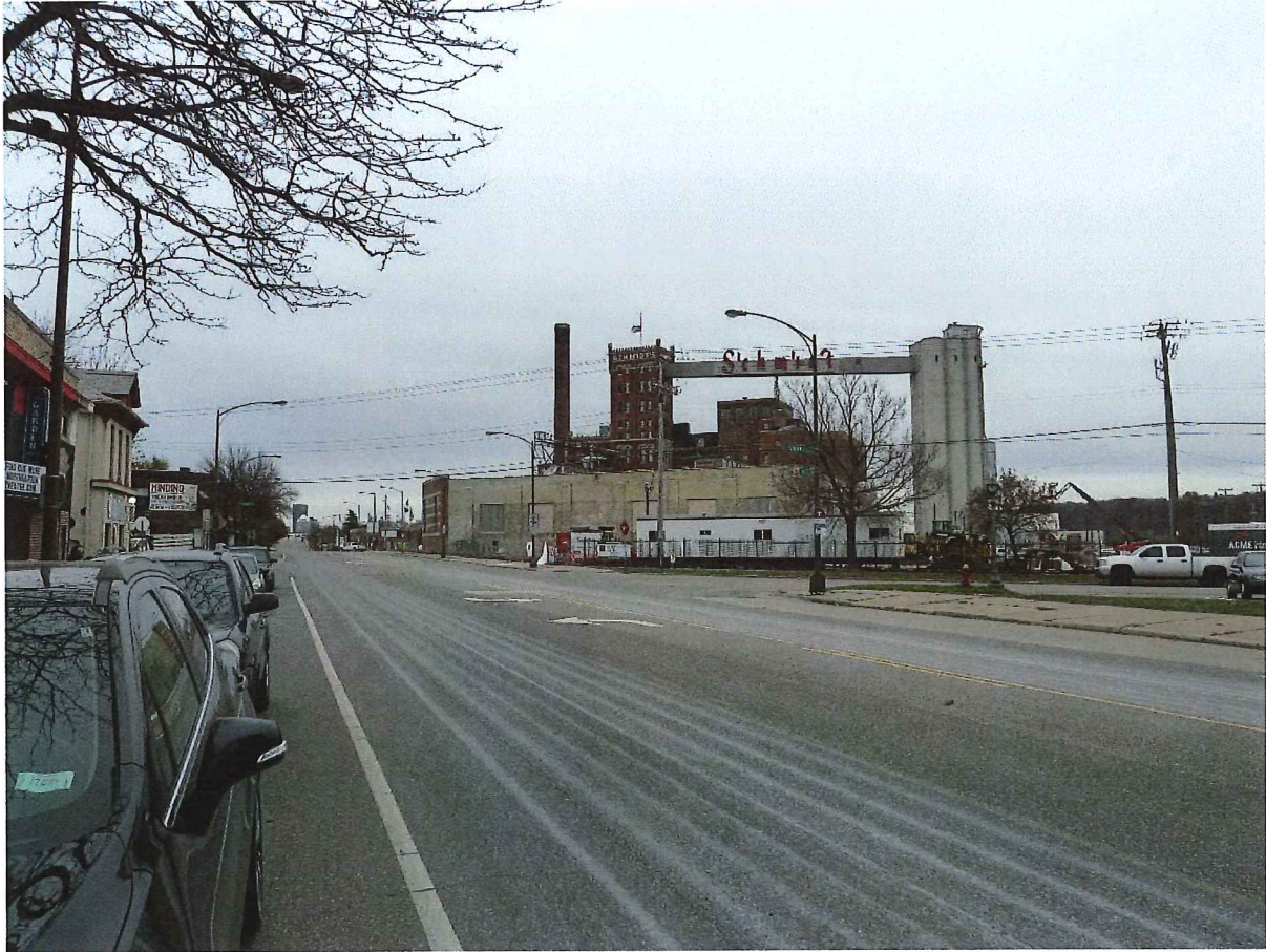
Photo 6. West elevation of building, December 2017.
