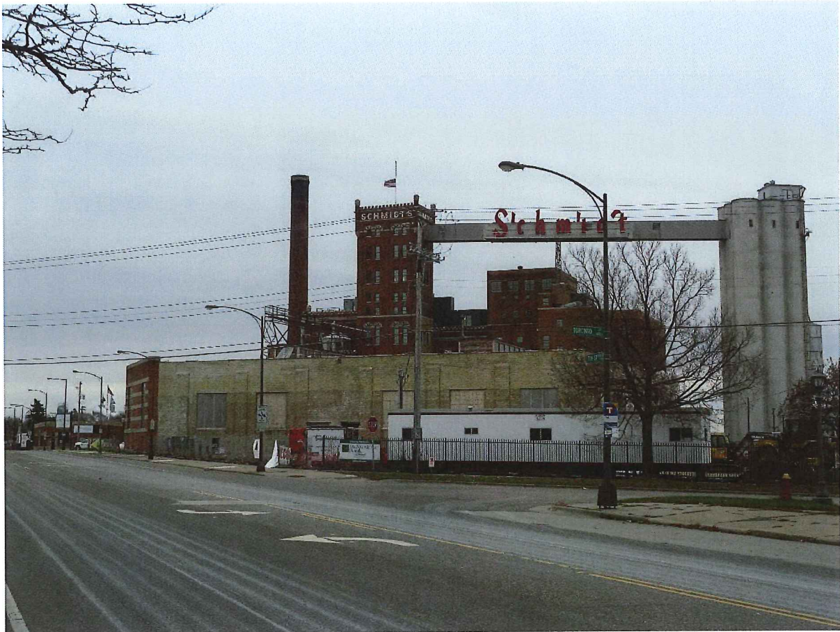
Photo 5. West elevation of building, December 2017.
