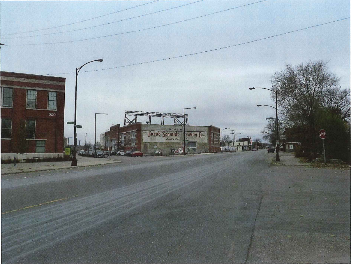
Photo 8. North, northwest, and east elevations of building, December 2017.
