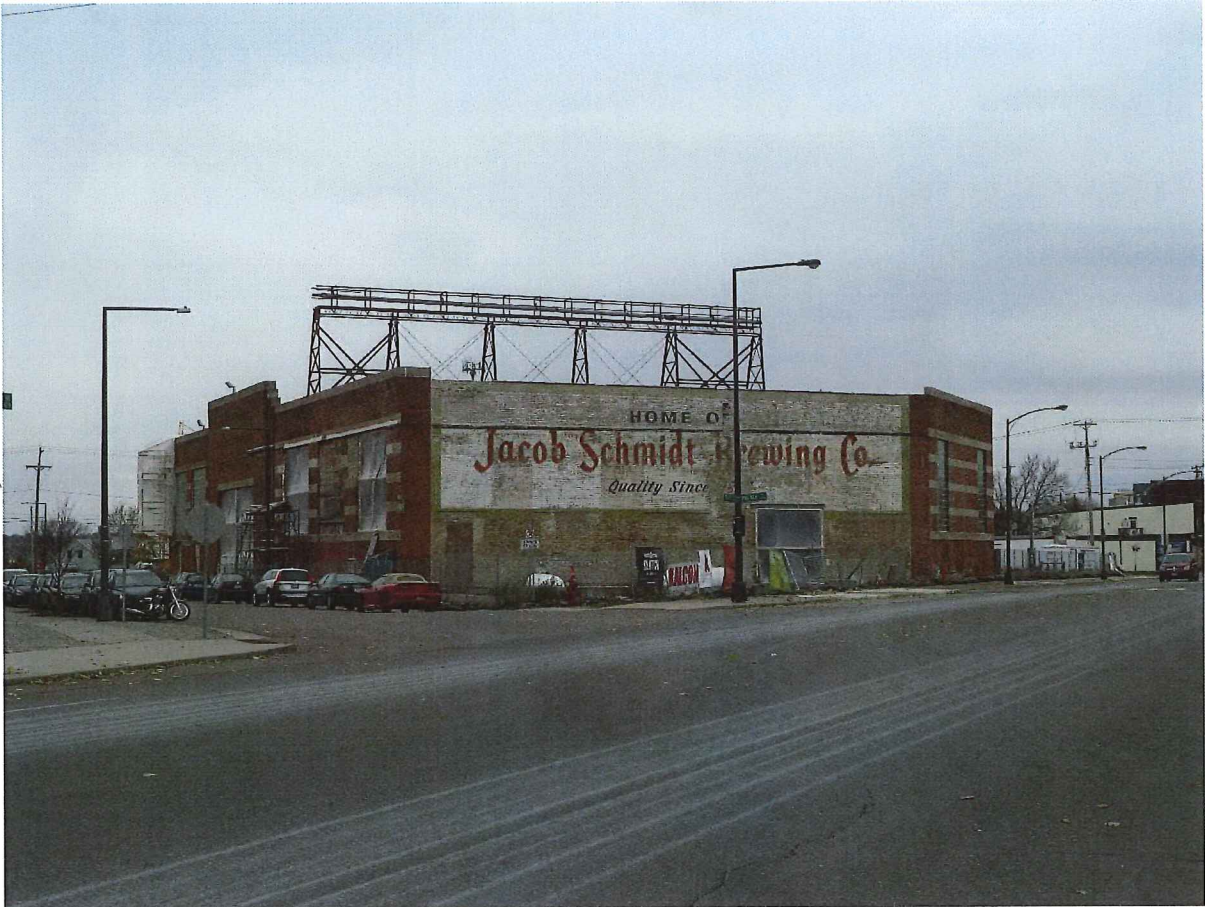
Photo 9. North, northwest, and east elevations of building, December 2017.
