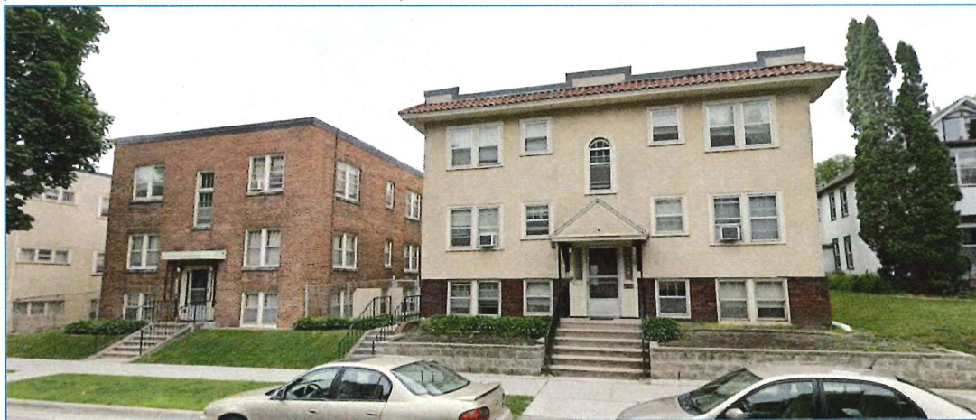
1848 St. Clair Ave – 14 units built in 1938 (~5' side yard on west side) & 1854 St. Clair Ave – 10 units built in 1935 (~4' on east side and ~5' on west side)
