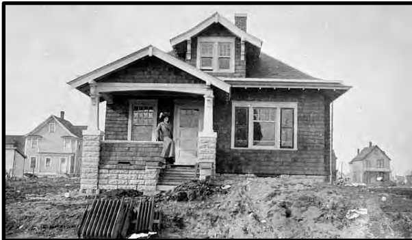
Hasslen House, 1912, looking north
