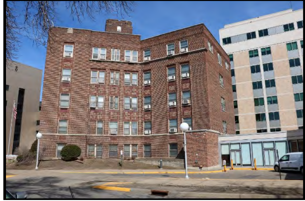
Midway Hospital, 2019, looking east
