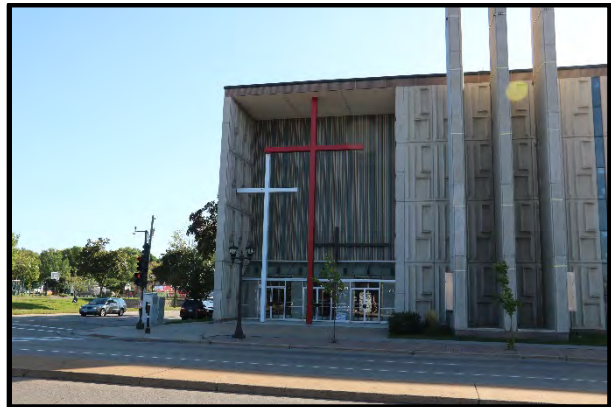
Jehovah Lutheran Church, 2019, entrance detail
