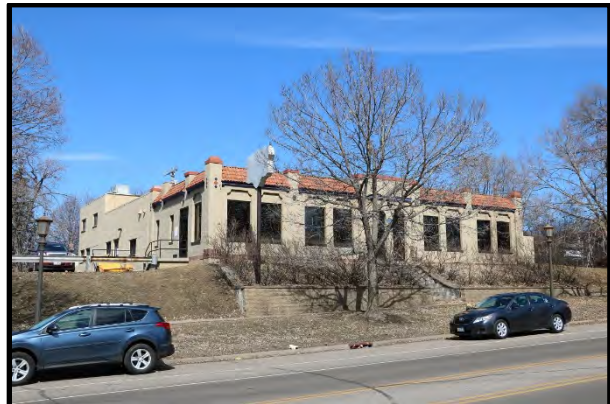
R. A. Myers & Co., 2019, looking northeast
