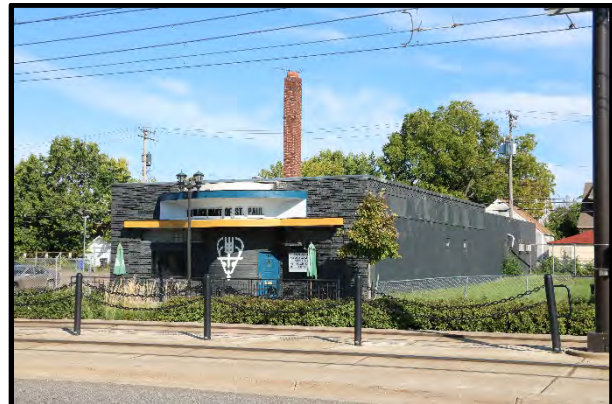
Town House Bar, 2019, looking northwest
