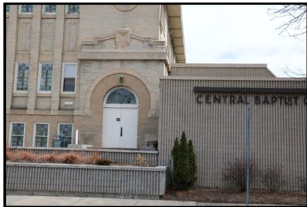
Central Baptist Church, 2019, addition connection
