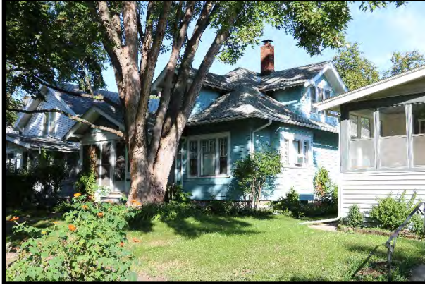
Hasslen House, 2019, looking northwest
