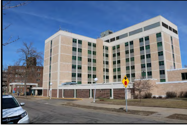
Midway Hospital South Building, 2019, looking northeast
