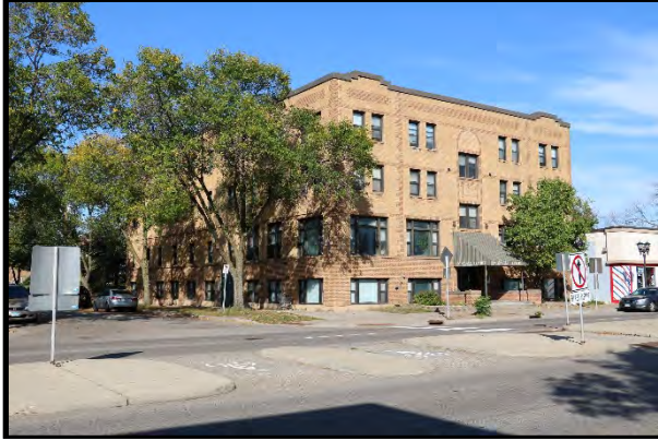
Hamline Hotel, 2019, looking northwest
