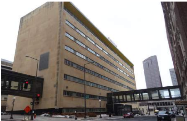
Figure 2.15: Block D, Minnesota Mutual Life Insurance Company/ Pioneer Press Building
