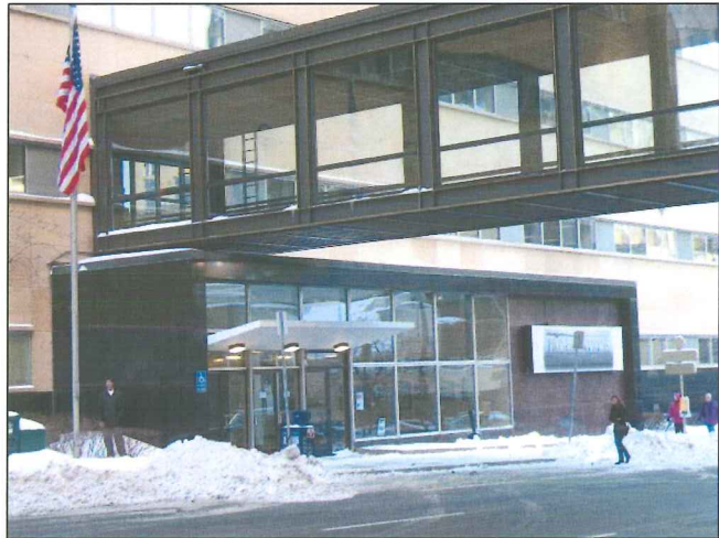
Detail photographs of the building cornice (upper) and Cedar Street entrance (lower), 2008.
