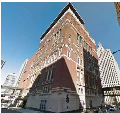
Figure 2.16: The Saint Paul Athletic Club occupies the southern corner of the Central Station block; Google, 2016
