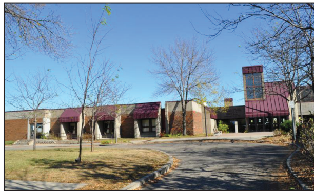
Figure 27. Martin Luther King Community Center (Prepare and Prosper 2017)
