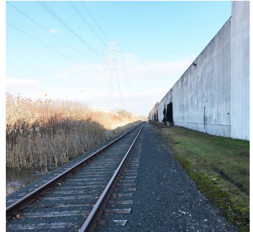
Existing conditions between Rankin and Homer Streets
