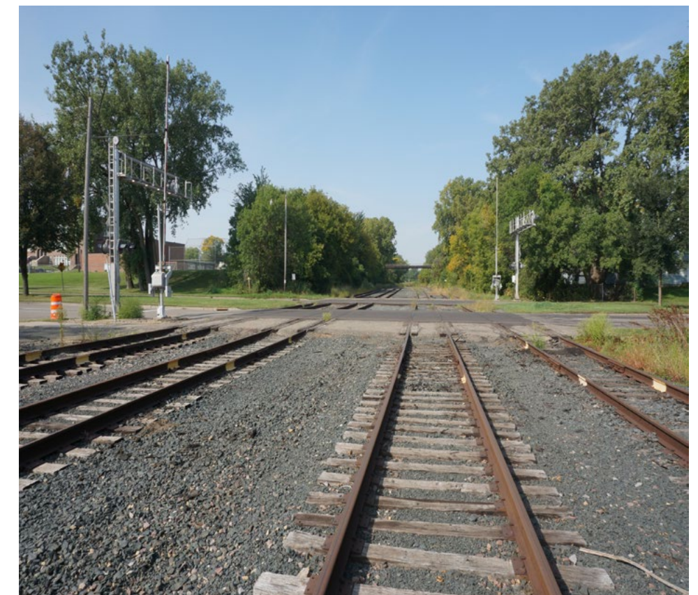
Existing conditions at Edgcumbe Road
