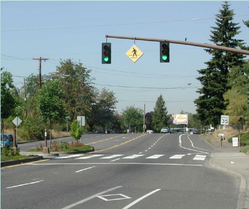
The Springwater Corridor in Portland, Oregon includes high visibility crosswalk markings, pedestrian warning signs, and pedestrian activated signals at crossings.
