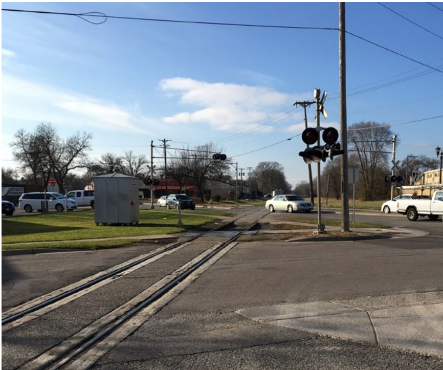
The spur crosses a complex intersection at W 7th and Alton St which will require a grade separated crossing for trail users.
