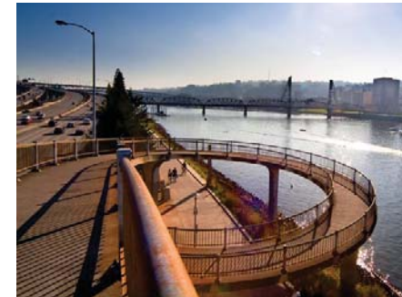
Grade-Separated Crossings: Structures are reserved for roadways with high traffic volumes and speeds, where crossing at a signal is not practical.
