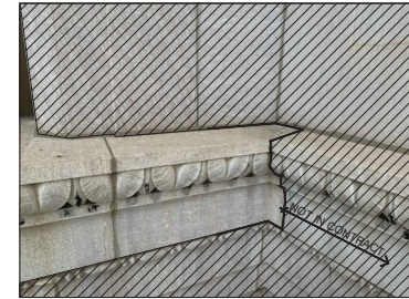
4 SE CORNER EXTENTS @ 4TH FLOOR WATERTABLE A3.2 SCALE: N.T.S.
