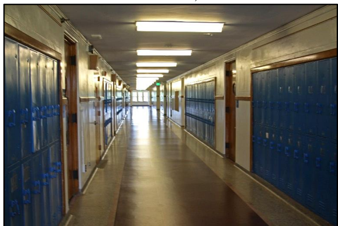
Hallway with recessed lockers, terrazzo and vinyl floors, and plaster ceiling
