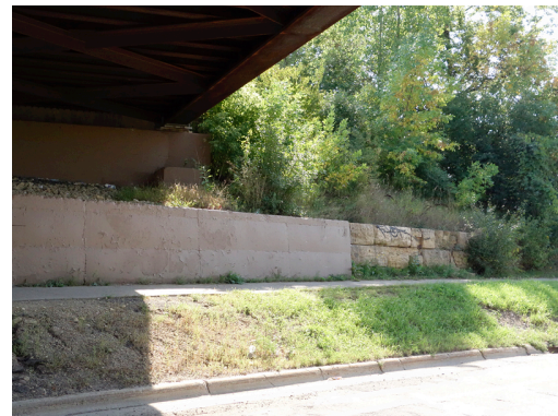
Figure 5. Stone and concrete retaining wall, under CM& StP Railway Bridge No. 92258, at Prior Avenue N.
