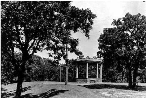
Figure 33. Pavilion, ca. 1909 (razed).
