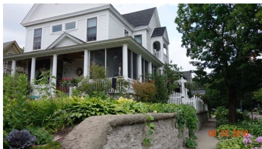
Figure 23a. 1818 Iglehart, limestone wall detail.
