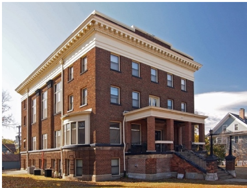
Figure 55. Charles Thompson Memorial Hall, 1824 Marshall Avenue (1916, NRHP).
