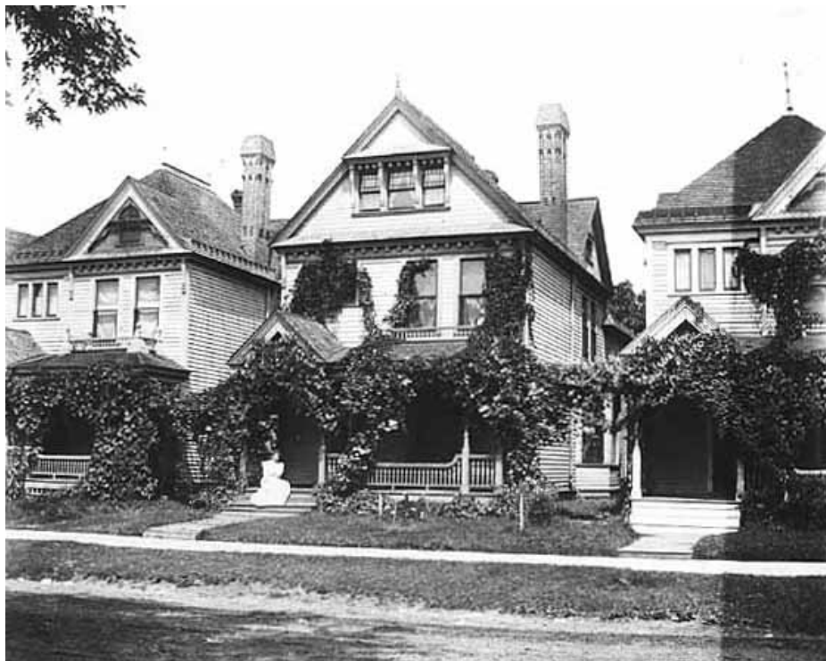
Figure 12. From left, 1927, 1925, and 1921-23 St. Anthony Avenue (1889), in ca. 1910 (razed).
