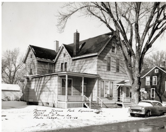
Figure 60. 335-337 N. Prior Avenue, razed for park expansion, ca. 1968. (RCHS)
