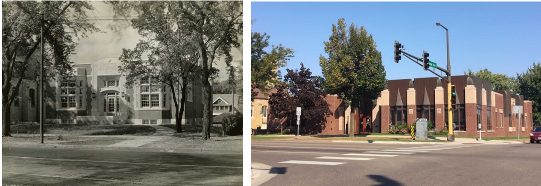
Figure 32. Henry Hale Branch Library, 1831 Marshall Avenue, 1930 (razed), at left; new building of 1993, at right.
