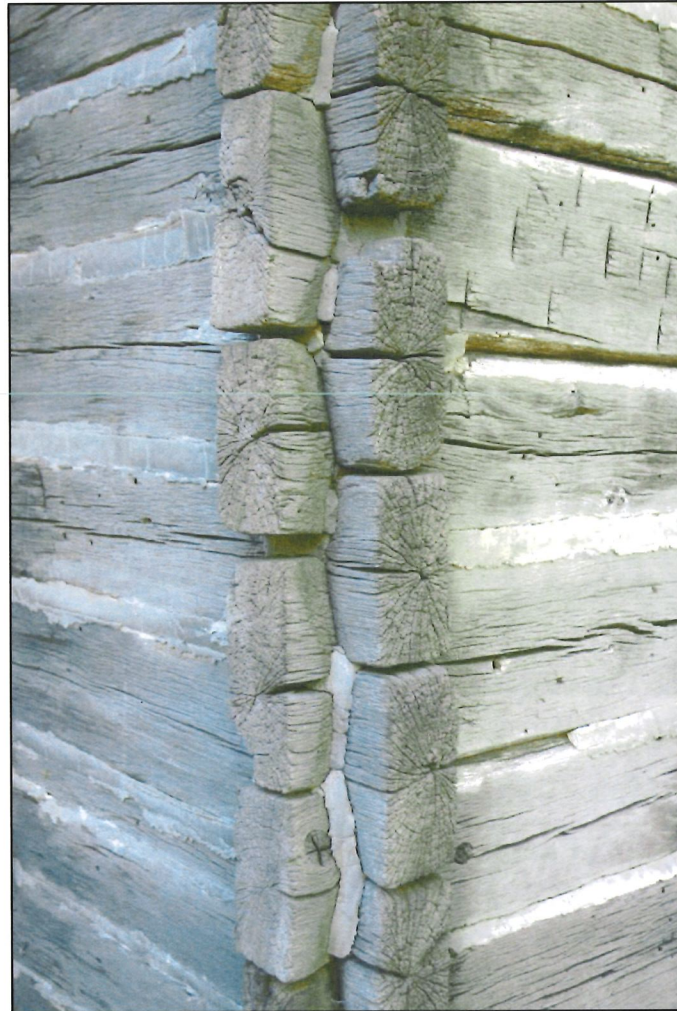
Photograph 5: Detail of log notching at northwest corner, looking southeast.
