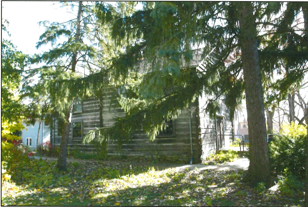
Photograph 4: West and north facades, looking southeast.
