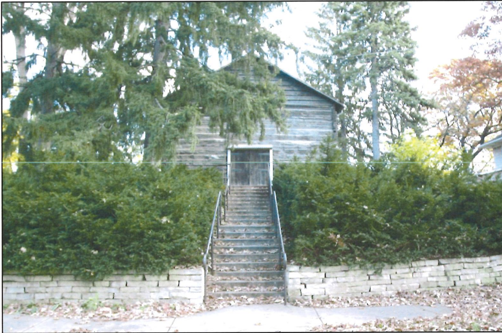
Photograph 1: West (front) facade, looking east.
