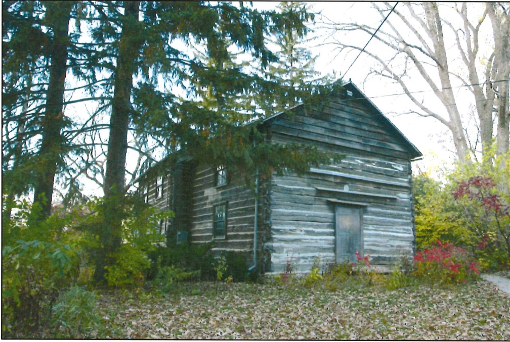
Photograph 3: East (rear) and south facades, looking northwest.
