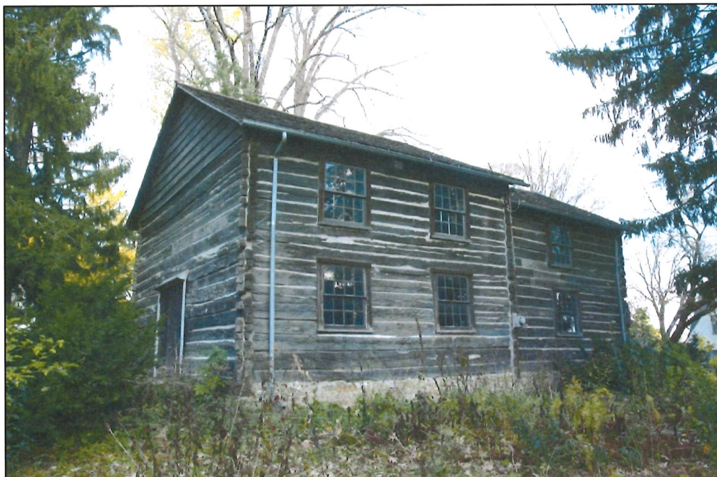
Photograph 2: West and south facades, looking northeast.
