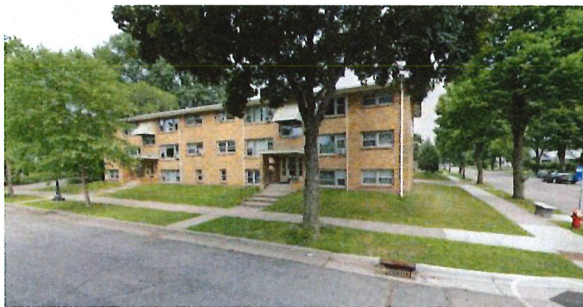
Suburban Style in-fill Multifamily: (RM2) Larger Complexes, 2.5 Stories, on combined/multiple lots, garages + surface parking (approx. 2 per unit)
