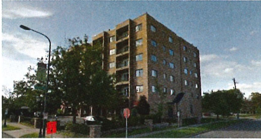
Suburban Style in-fill Multifamily (RM2): Larger Complexes, 5 Stories, on combined/multiple lots, structured parking (approx. 1.5 per unit) Est. FAR 1.3 Lot size 21,000 SF Block Density 6,800 PPM
