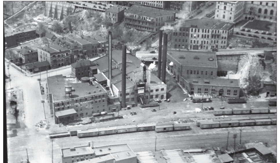
Figure 27. Mixed land uses along the rail corridor at the foot of the bluff at Hill Street, 1925.
