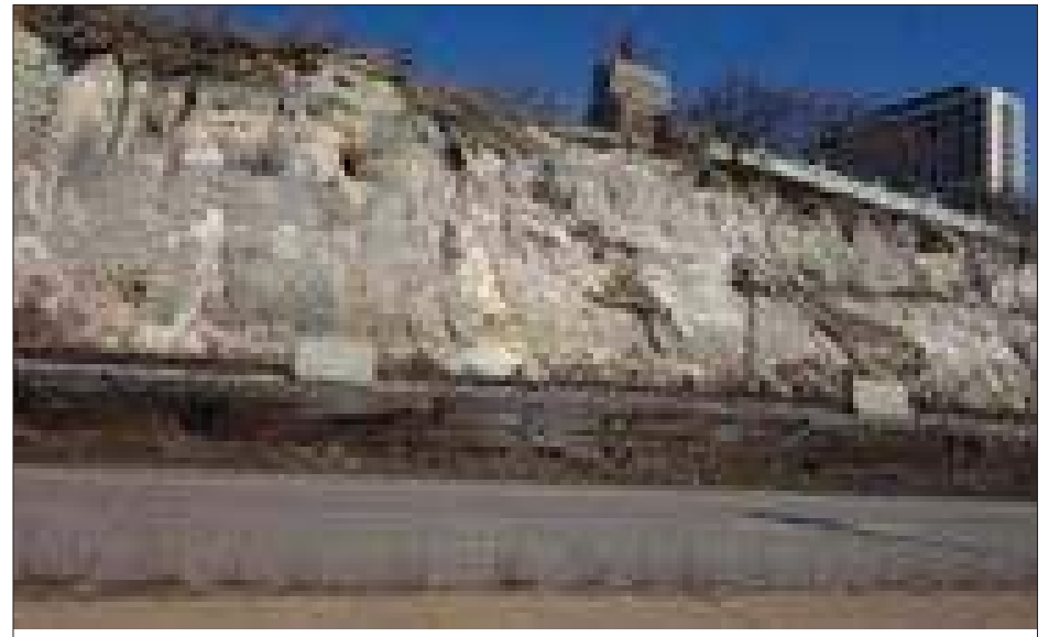
Figure 11. Bluff between Wabasha and Robert Street bridges above Shepard Road, 2015 (left); the bluff in ca. 1925 (right). Fuel storage tanks and billboards line the edge.
