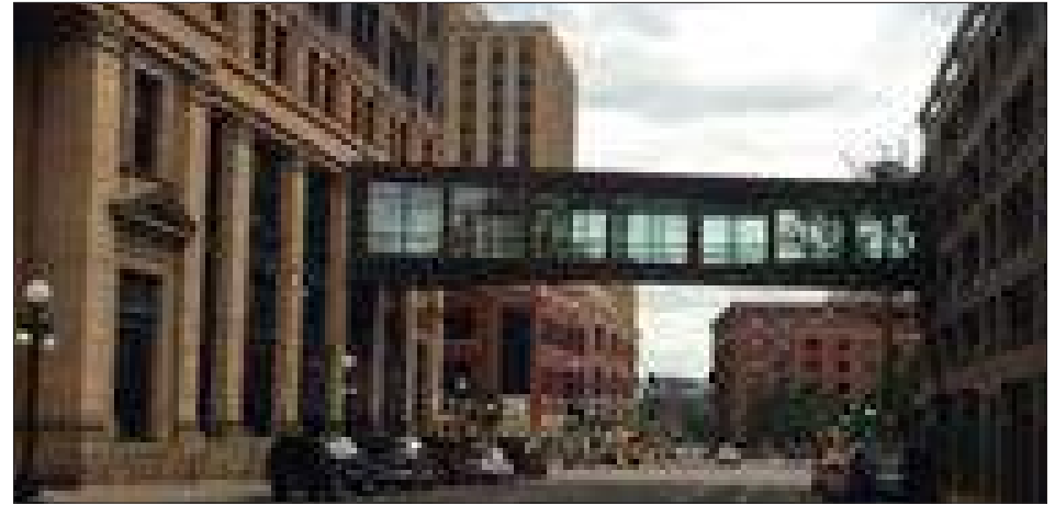
Figure 41. Example of one type of visual effect: looking south from Jackson Street in the Lowertown Historic District to Kellogg Boulevard and the Farwell, Ozmun & Kirk Warehouse (NRHP) and U.S. Post Office and Custom House (NRHP), August 2015. Physical connection to historic properties and obstruction of views NRHP facades would be among factors considered in design review.
