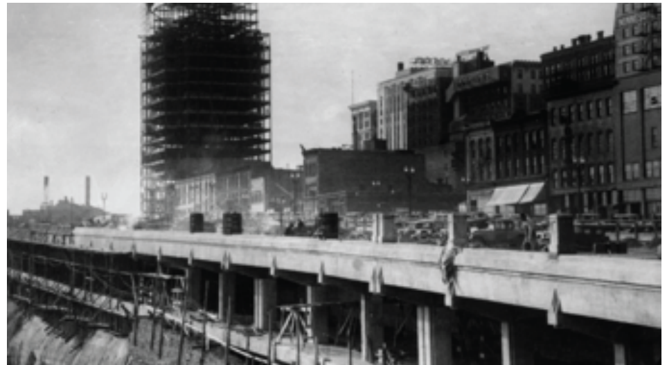
Figure 31. The skeleton of St. Paul City Hall/Ramsey County Courthouse rises above the new Kellogg Boulevard, ca. 1930.
