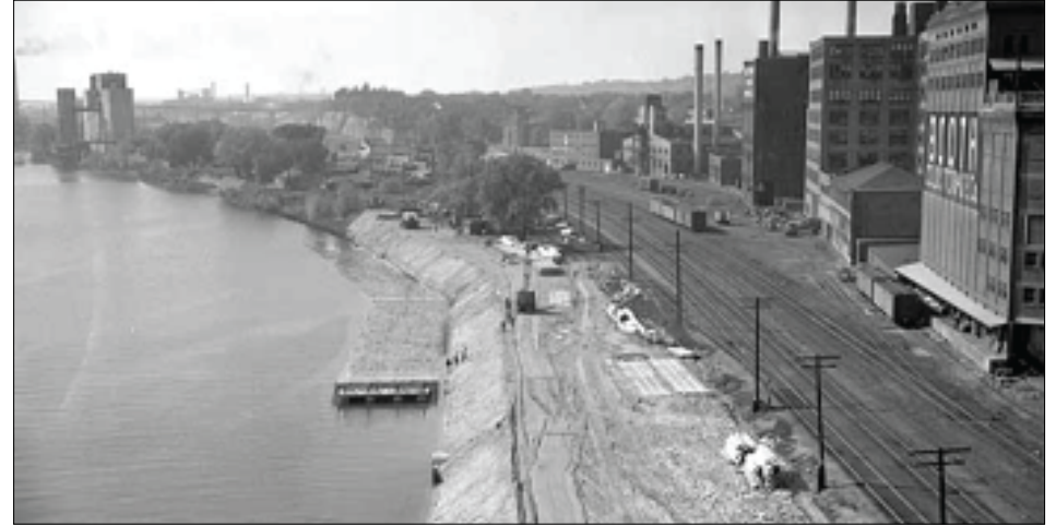
Figure 37. Filling along the future Shepard Road below the West Publishing Co. and Northern States Power and other plants, ca. 1947.
