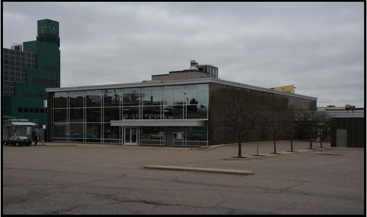
Figure Thirty: Rear (south) elevation of the former Midwest National Bank Building (Structure 1). View to northwest toward the intersection of Snelling and University Avenues.
