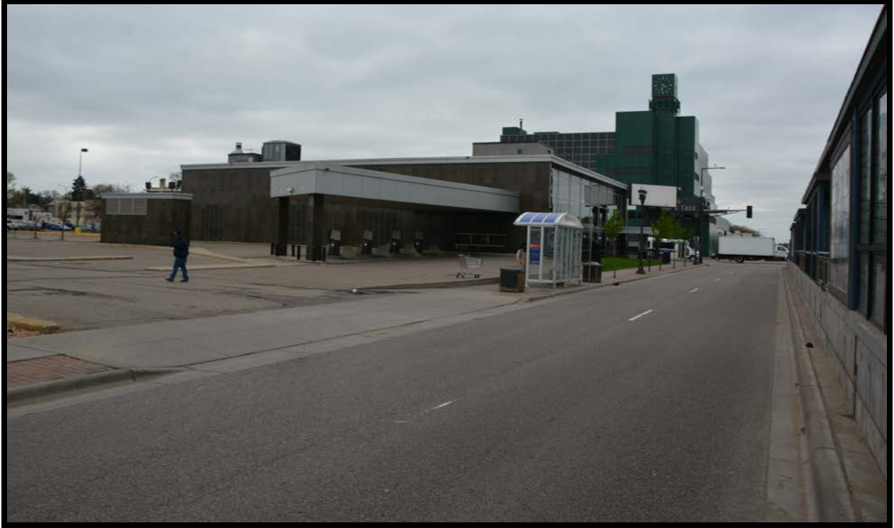
Figure Thirty-Four: Eastern and northern elevation of the former Midwest National Bank Building (Structure 1). View to southwest from University Avenue.
