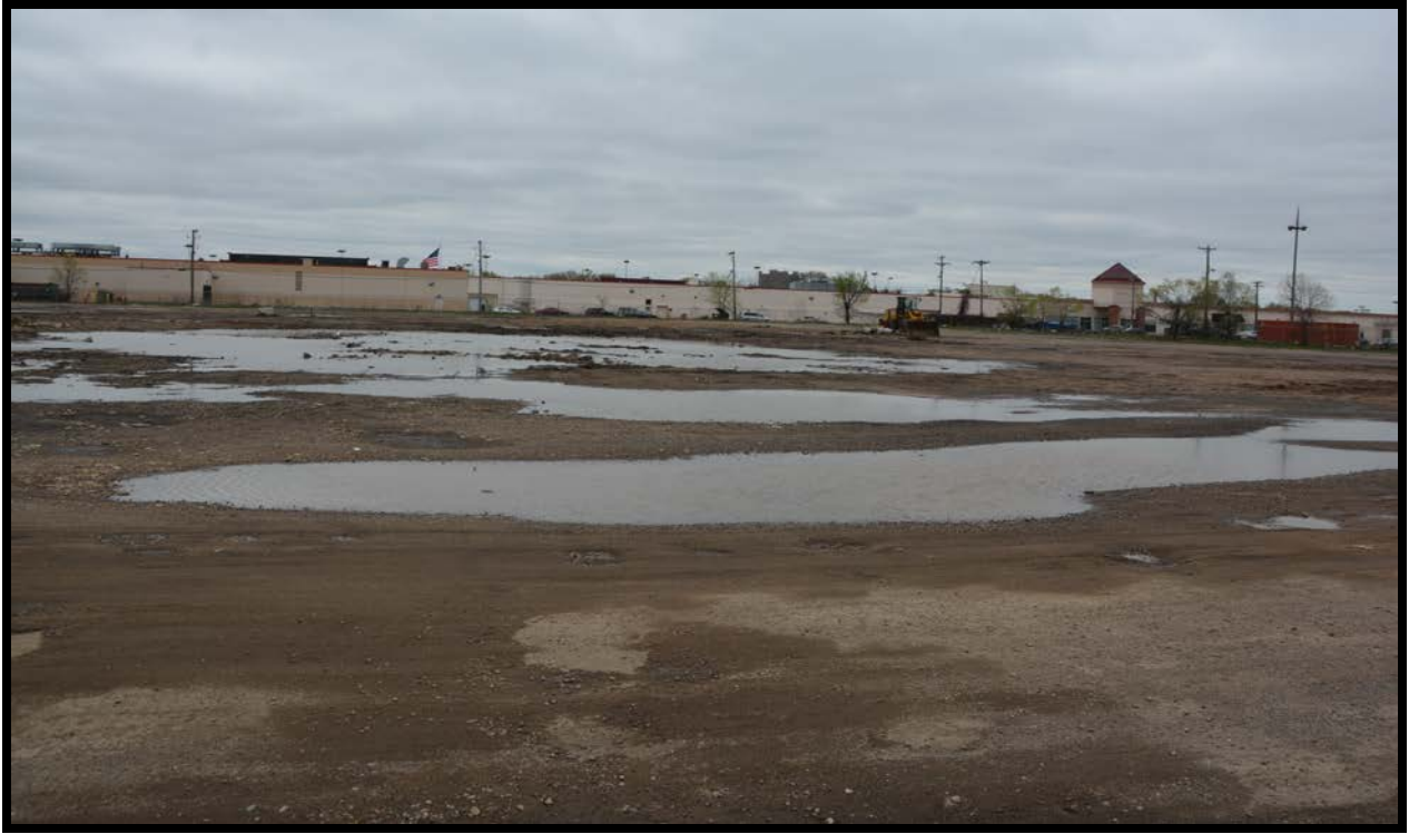
Figure Fifty-Five: North central area of Area A. View to north of former bus barn location and southern (rear) elevation of Structure 5.
