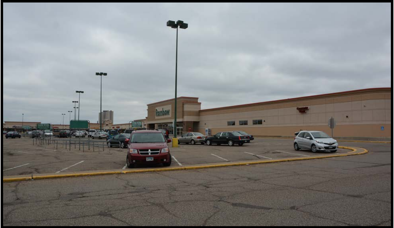
Figure Twenty-Three: Main parking area of the Midway Center Shopping Mall (Structure 5 in Figure Five) View to southeast.
