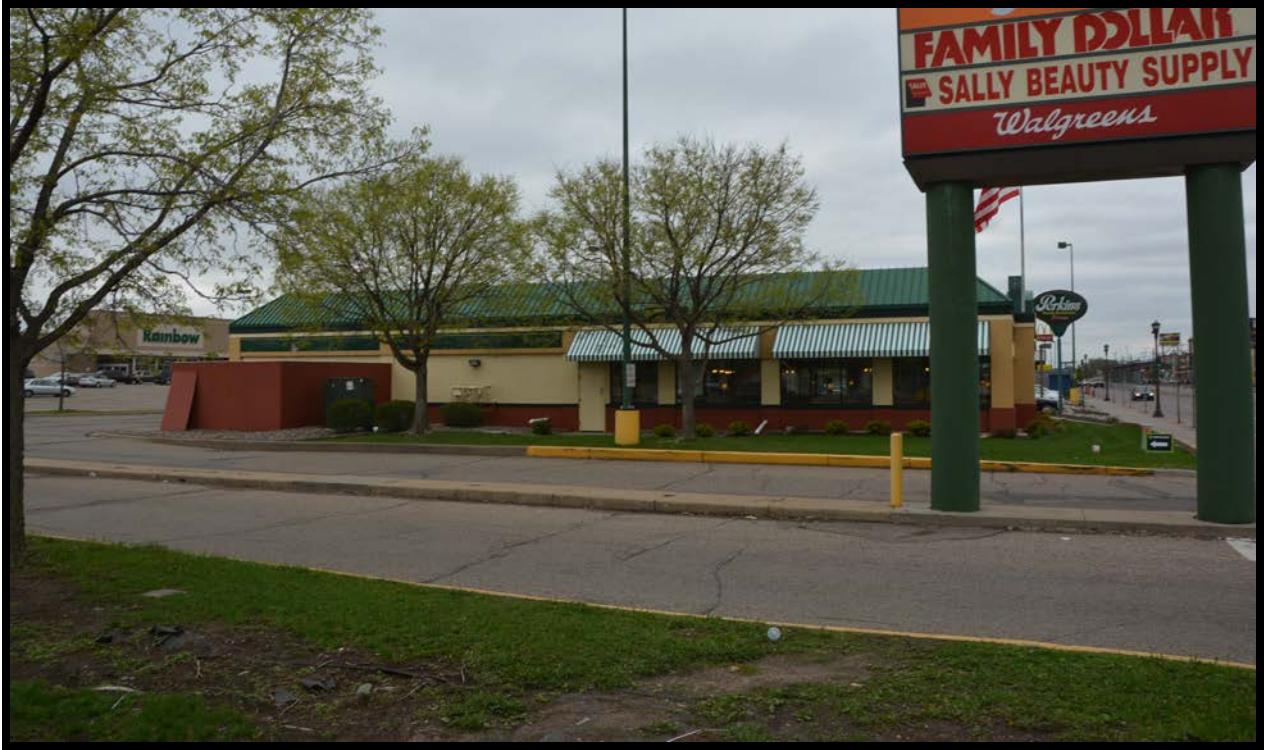
Figure Forty-Two: Eastern (rear) elevation of Structure 4. View to west.
