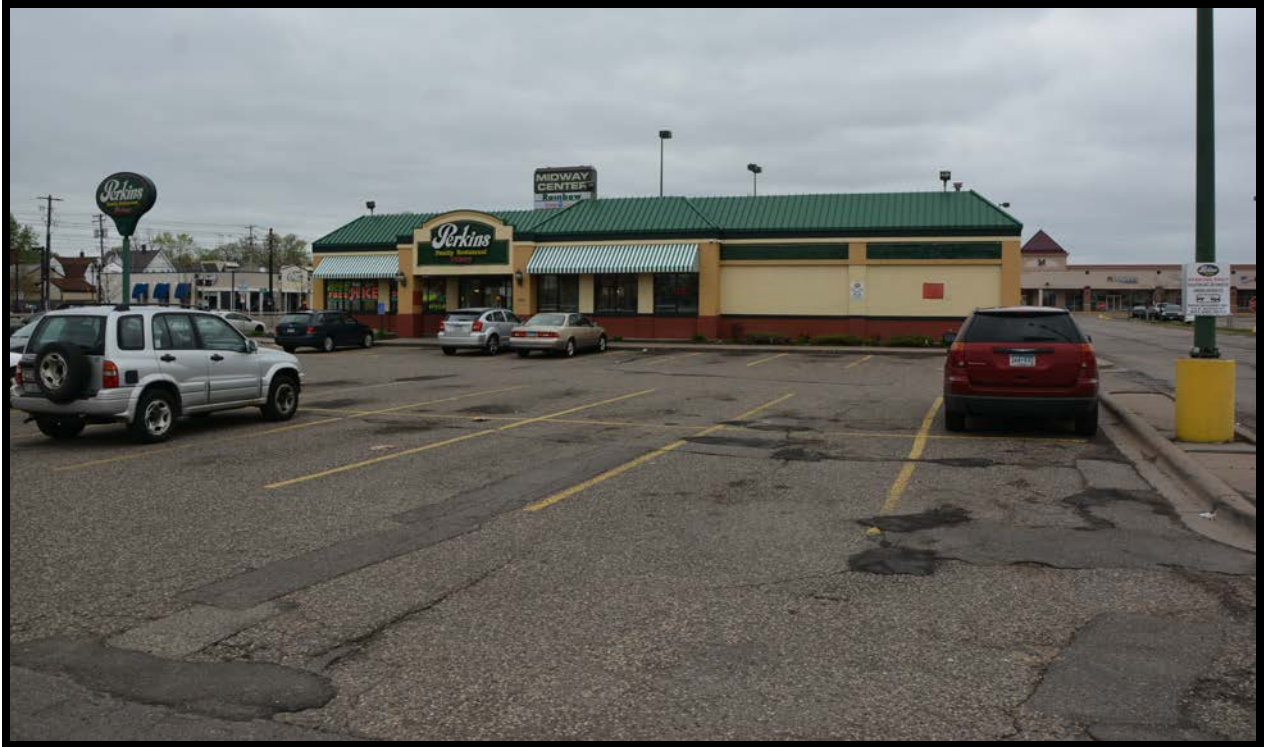
Figure Forty-One: Western (front) elevation of Structure 4. View to east.
