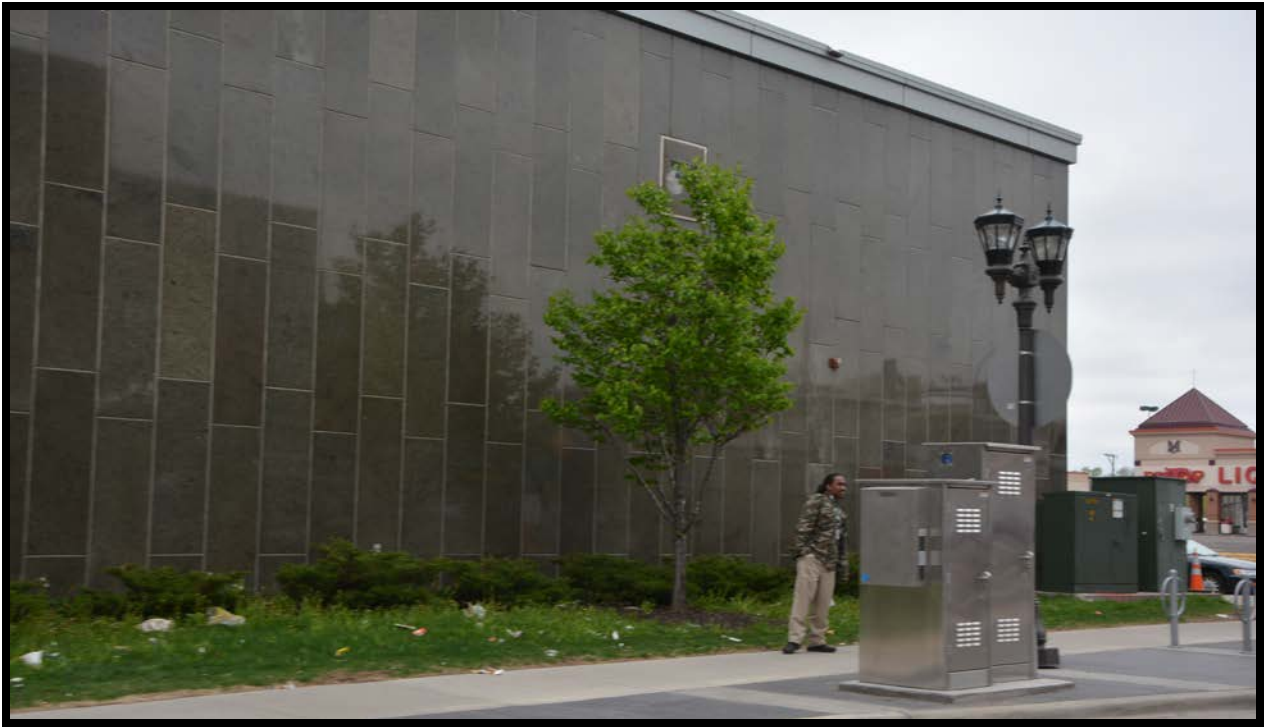
Figure Thirty-Seven: Southern areas of the western elevation of the former Midwest National Bank Building (Structure 1). View to southeast from Snelling Avenue.
