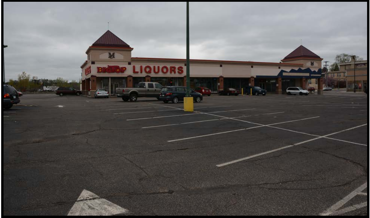
Figure Twenty-Four: Front (northern) elevation of Structure 2. View to south/southwest.
