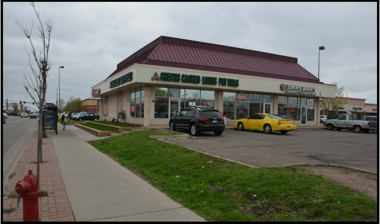
Figure Forty-Three: Western elevation of Structure 6. View to east/southeast.
