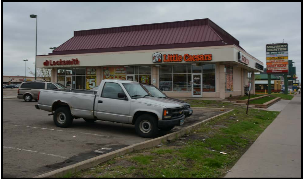
Figure Forty-Four: Eastern elevation of Structure 6. View to west/southwest.
