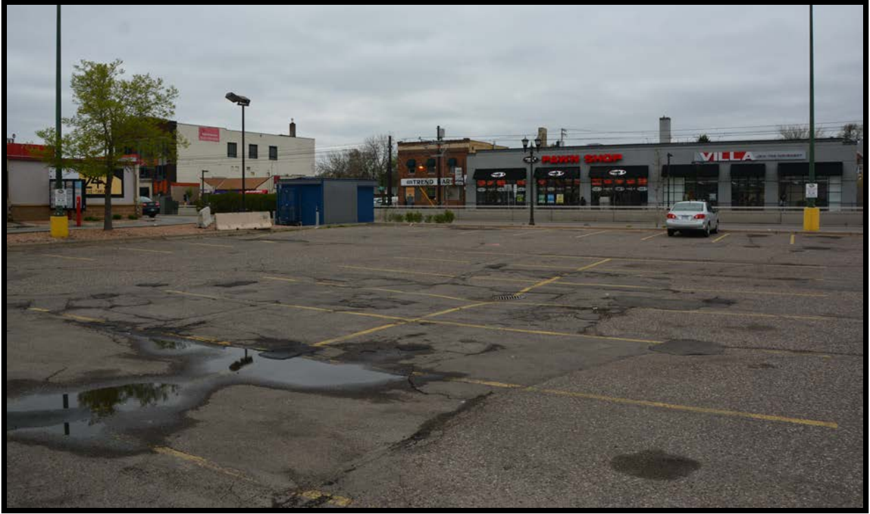
Figure Nineteen: Main parking area of Structure 4 View to northwest towards University Avenue.
