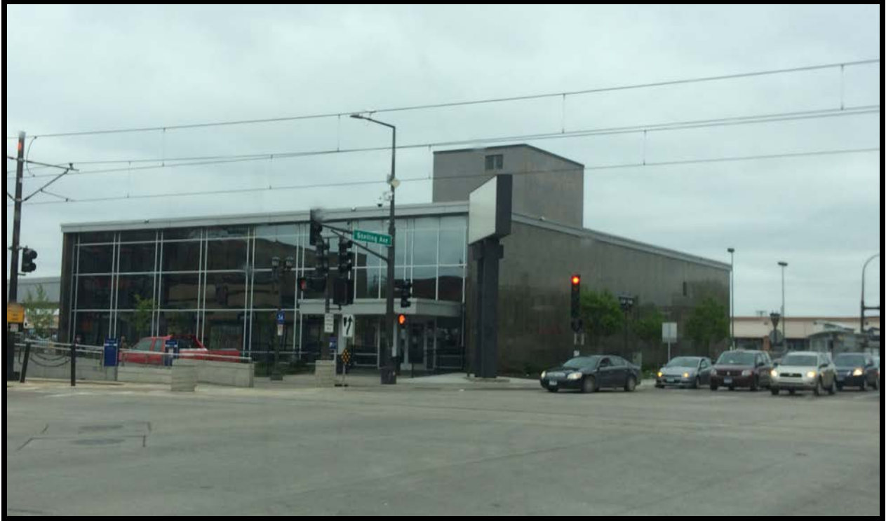
Figure Twenty-Six: Front (North) elevation of the former Midwest National Bank Building (Structure 1) . View to southeast from the intersection of Snelling and University Avenues.
