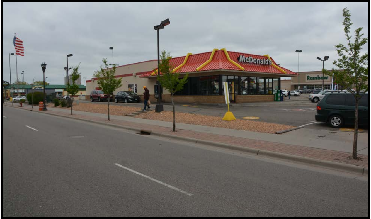
Figure Thirty-Nine: Northern and western (front) elevations of Structure 3. View to southeast.
