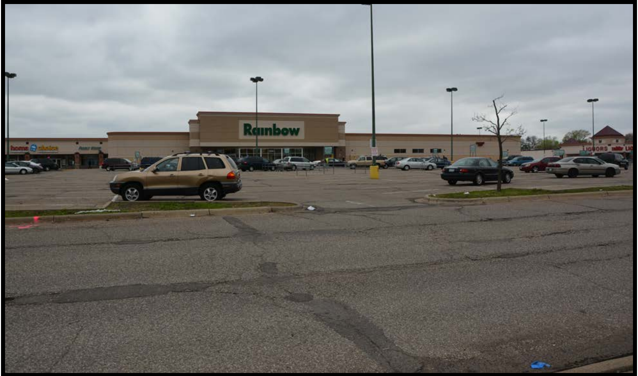
Figure Twelve: Front (northern) elevation of the Midway Center Shopping Mall (Structure 5 in Figure Five) showing post 1991 façade, paved parking areas and signage. View to south.
