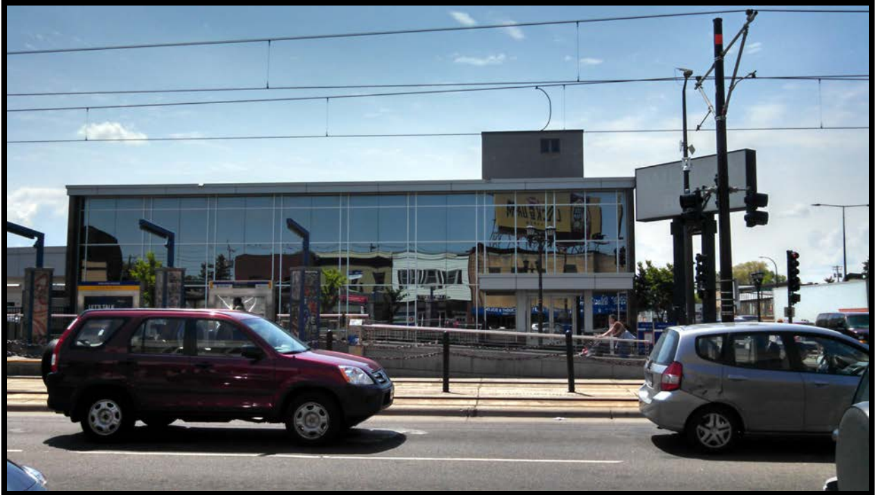
Figure Twenty-Nine: Front (North) elevation of the former Midwest National Bank Building (Structure 1). View to south with the intersection of Snelling and University Avenues to the right.
