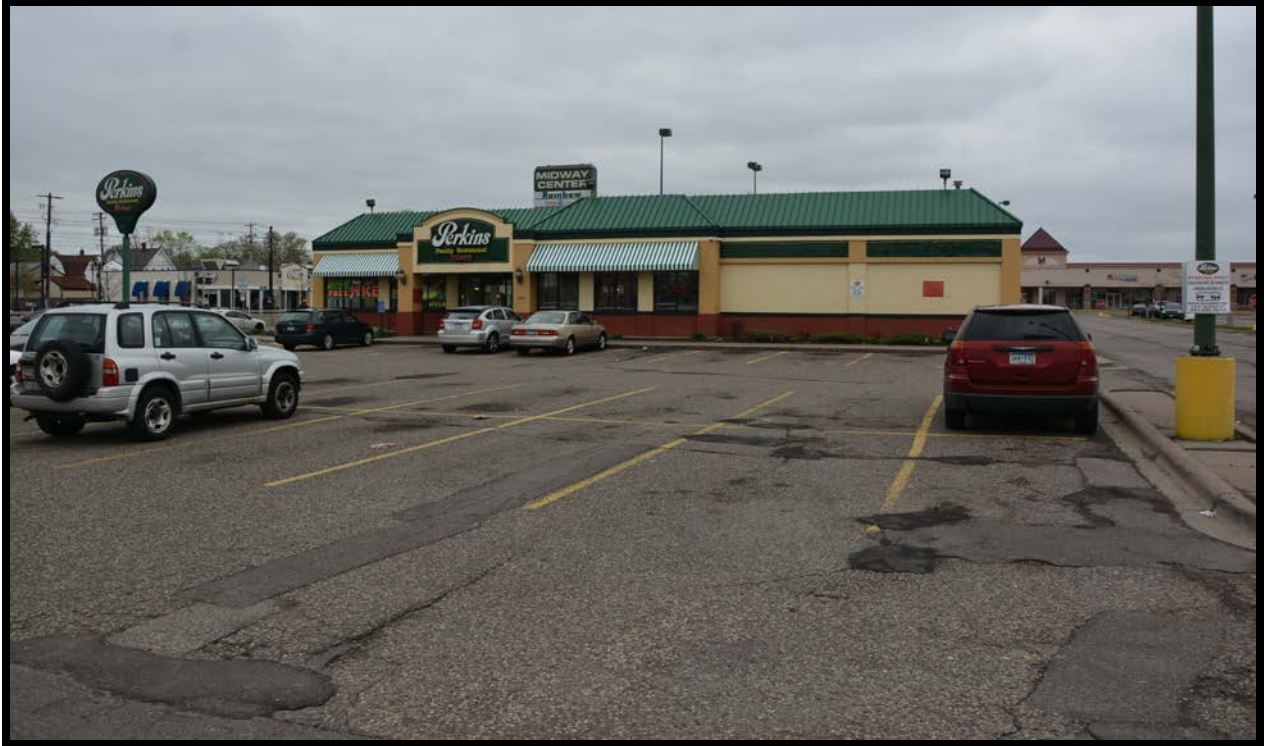
Figure Sixteen: Front elevation (west) of Structure 4 (Figure Five) View to east.
