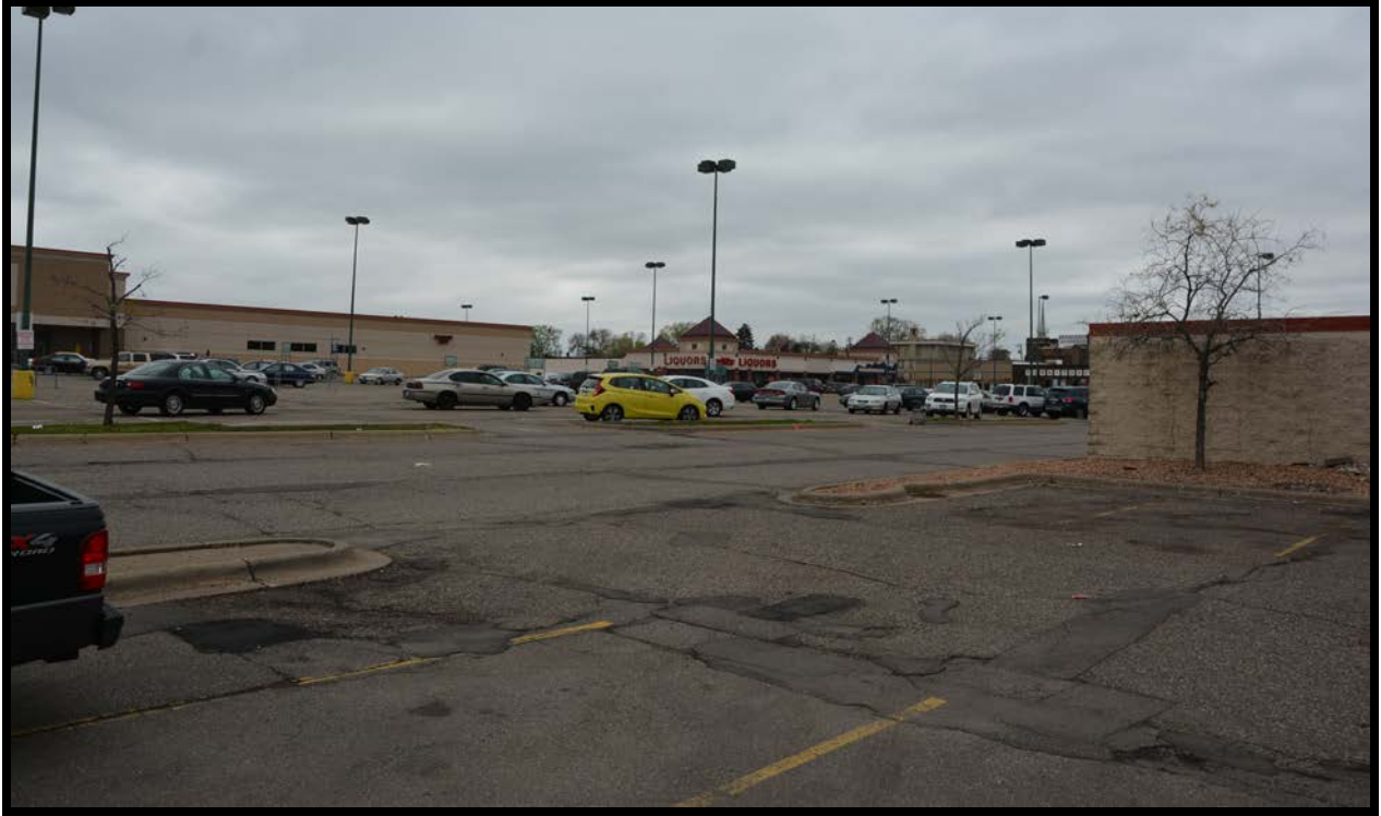
Figure Twenty-Two: Main parking area of the Midway Center Shopping Mall (Structure 5). View to southwest.
