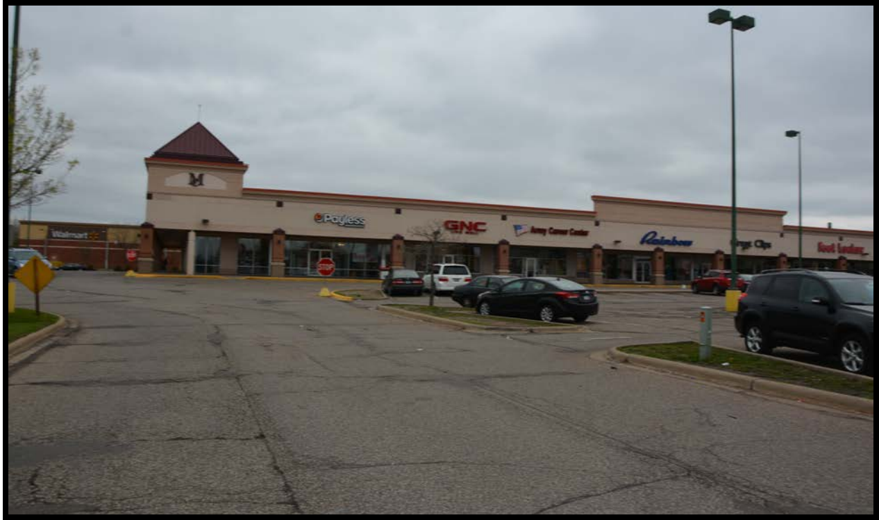
Figure Forty-Five: Front elevation (western) of the eastern wing of Structure 5. View to east/southeast.
