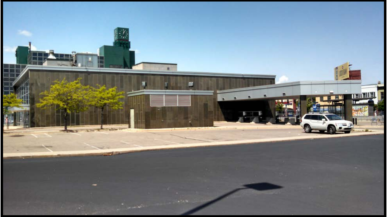
Figure Thirty-Three: Eastern elevation of the former Midwest National Bank Building (Structure 1). View to west/northwest showing drive-through lanes and parking area.
