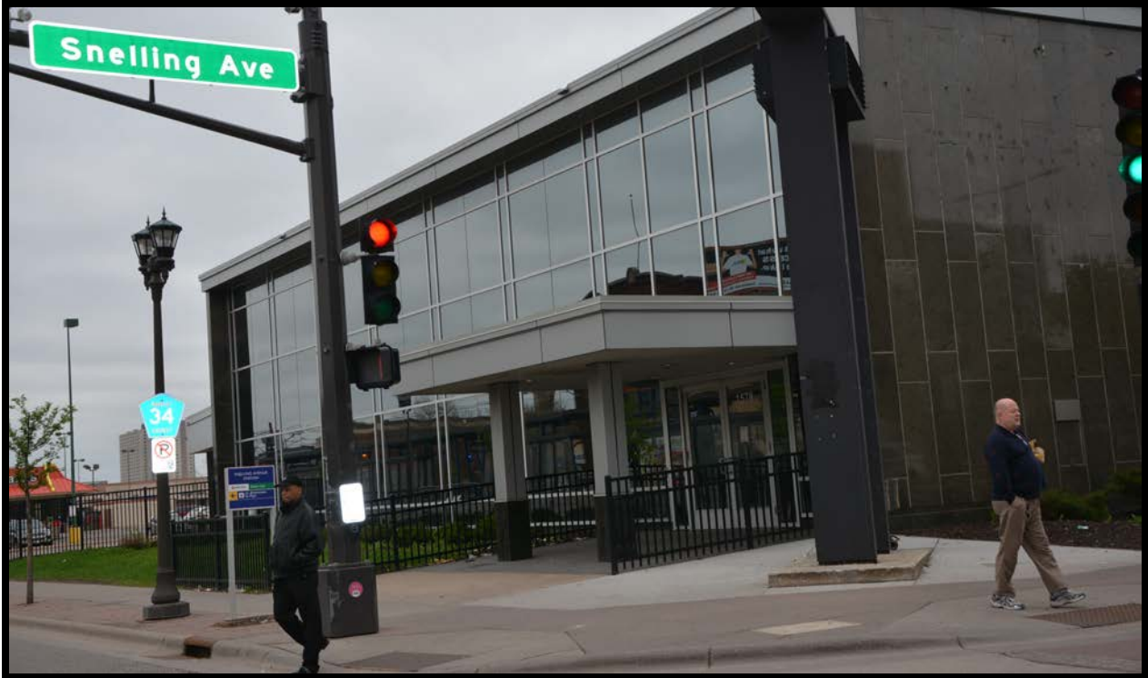
Figure Twenty-Seven: Front (North) elevation of the former Midwest National Bank Building (Structure 1) . View to southeast from the intersection of Snelling and University Avenues.
