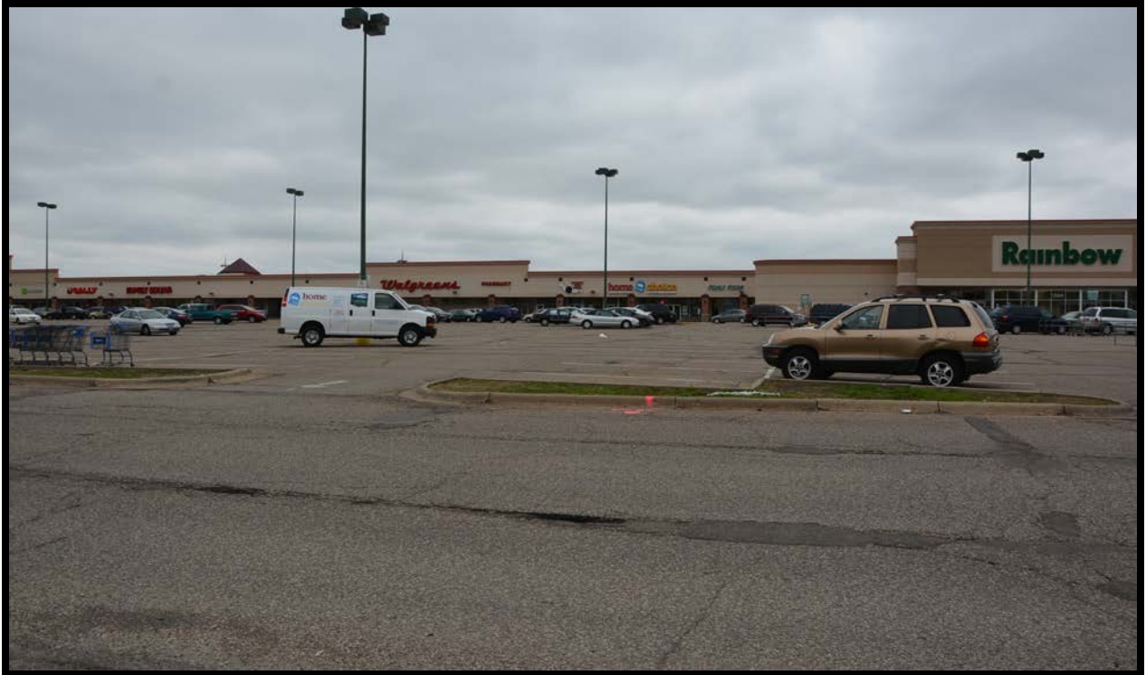
Figure Thirteen: Front (northern) elevation of the Midway Center Shopping Mall (structure 5 in Figure Five) showing post-1991 facade and signage. View to southeast.
