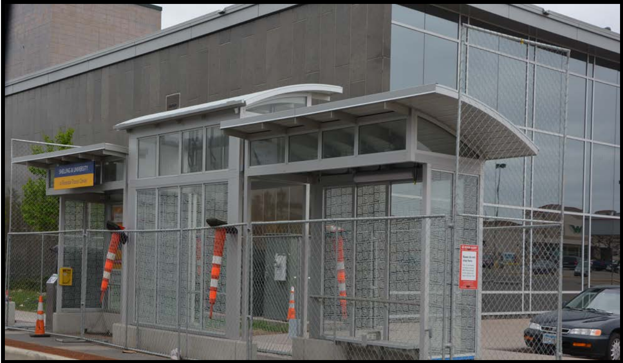
Figure Thirty-Five: Western elevation of the former Midwest National Bank Building (Structure 1). View to northeast from Snelling Avenue.
