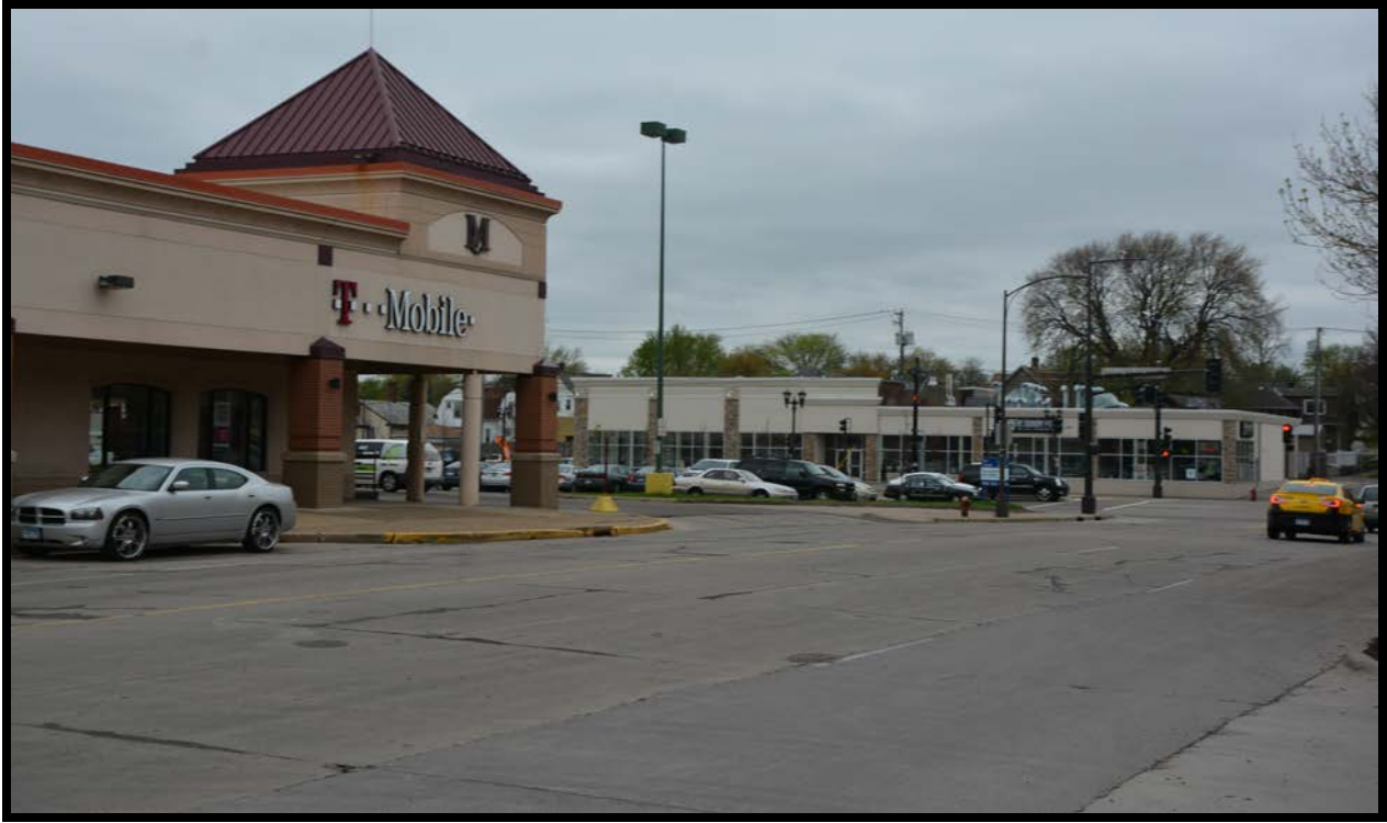
Figure Forty-Seven: Eastern elevation of the eastern wing of Structure 5. View to north/northwest from Pascal St.
