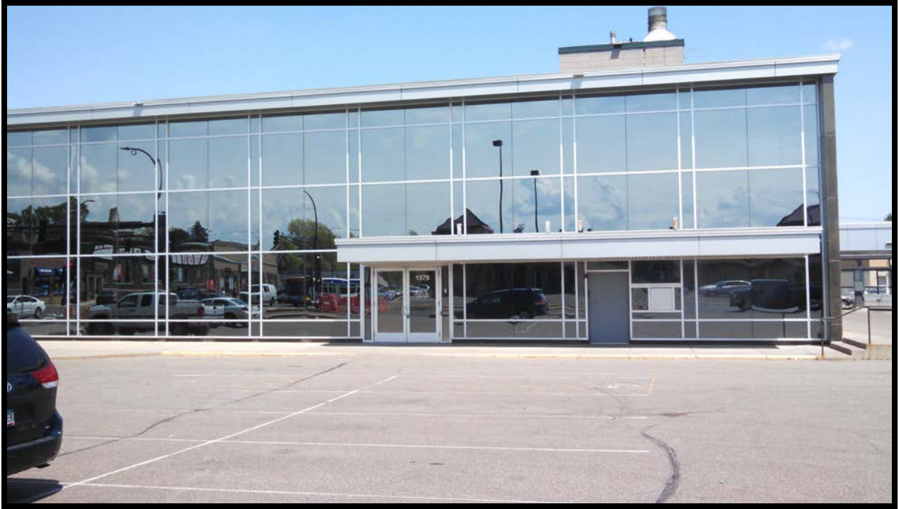
Figure Thirty-One: Detail of rear (south) elevation of the former Midwest National Bank Building (Structure 1). View to north toward the intersection of Snelling and University Avenues.
