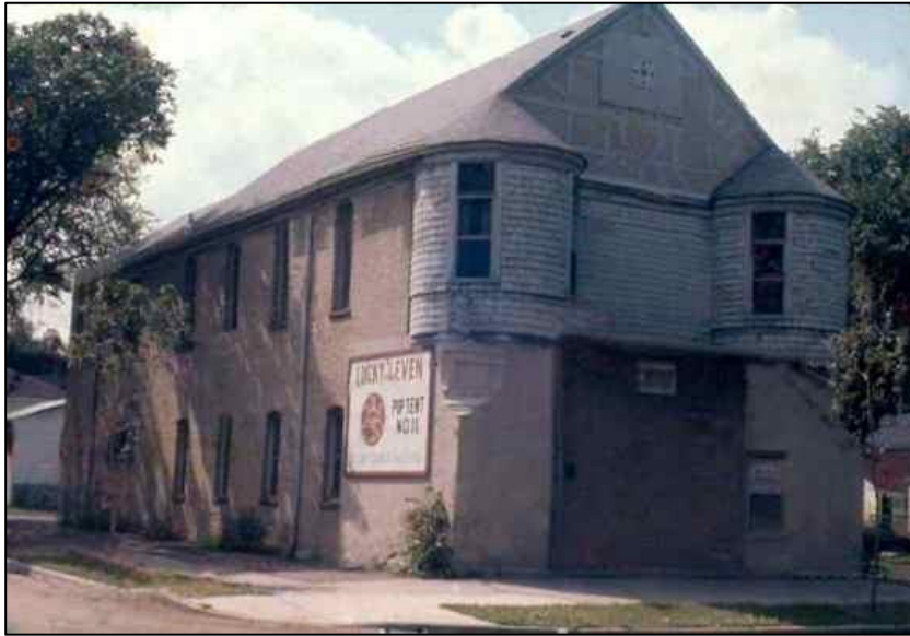
Figure 11. Station 12 at 700 Jackson Street NE, n.d. 57
