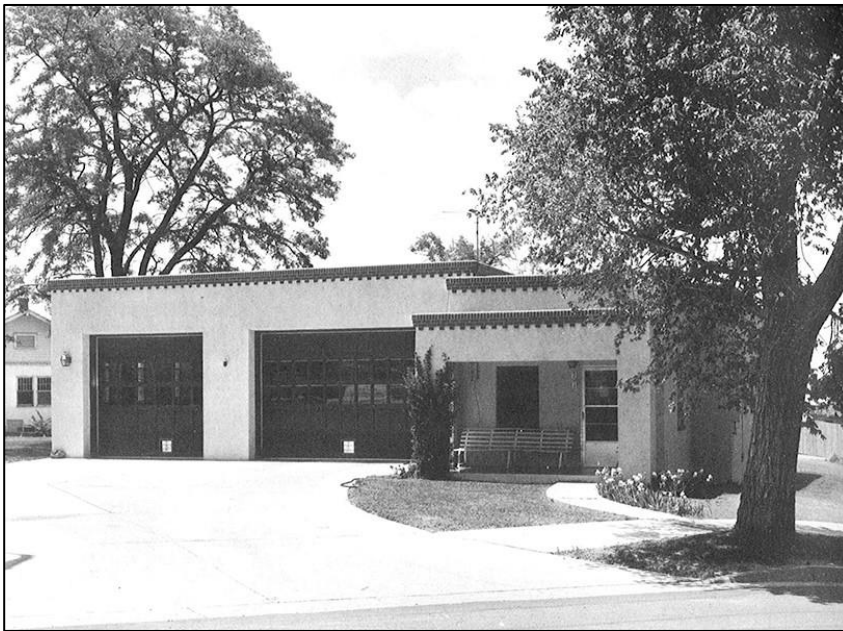
Figure 9. Fire Station 2, Albuquerque, New Mexico, built 1937 46
