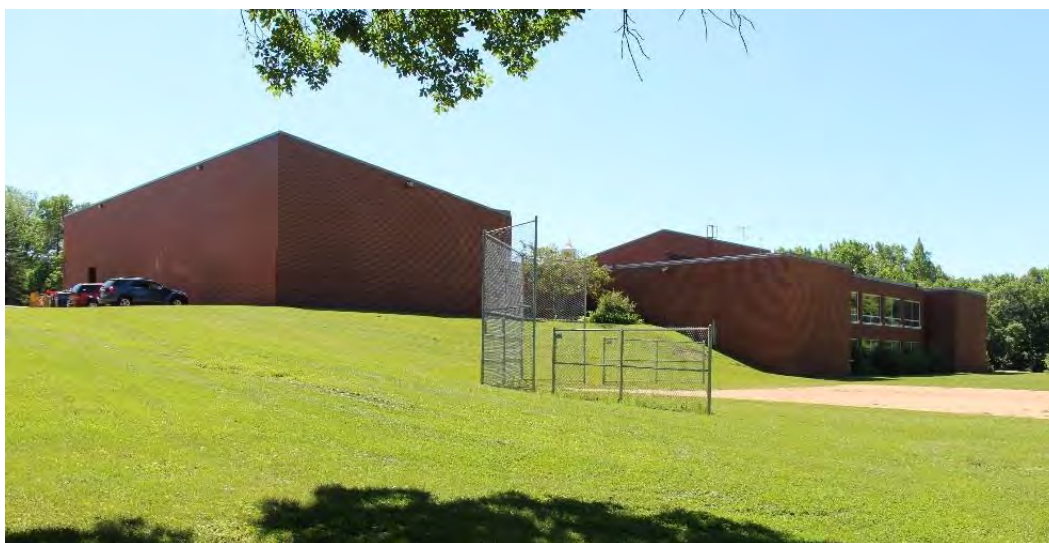
Figure 170. 1969 addition and baseball field, facing east.
