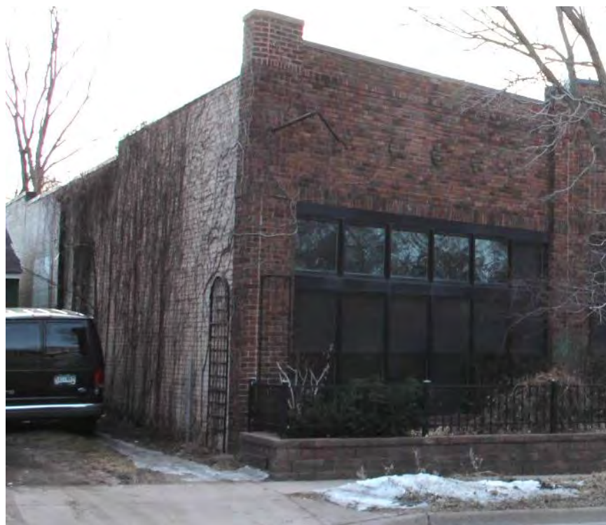
Figure 34. Side (north) elevation, view facing southeast. Note a bricked-in window at the far left of the image.
