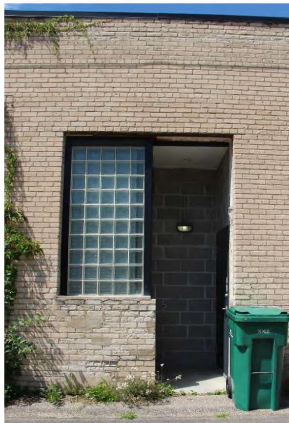
Figure 37. Detail of recessed entry with glass block wall and concrete block vestibule.
