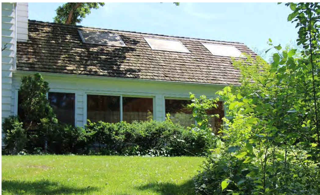
Figure 156. Overview of southern wing rear elevation, view facing southeast.
