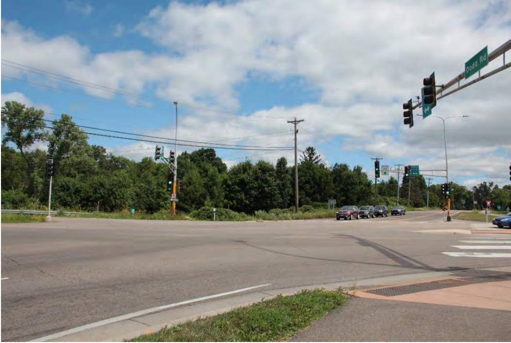
TH 149 Dodd Road at intersection with TH 110 in Mendota Heights, view facing northwest.
