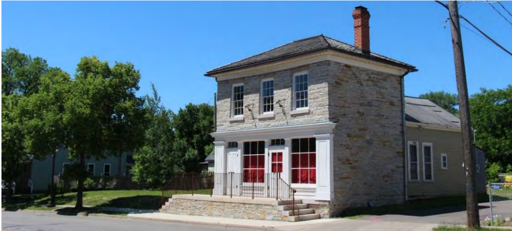
Front (east) facade and side (north) elevation of the Waldman Saloon, view facing southwest.
