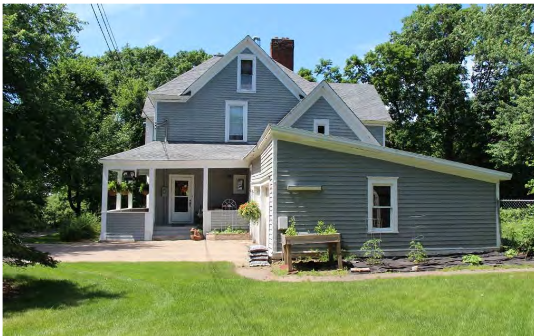
Figure 139. Rear (southeast) elevation, view facing northwest.
