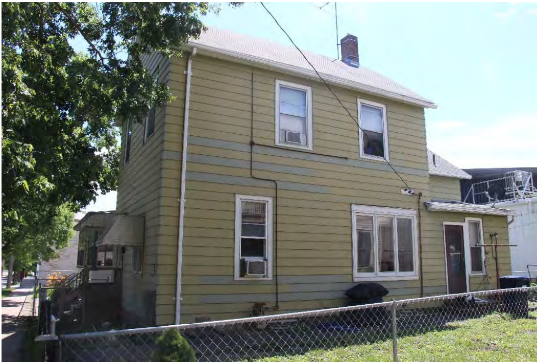
Side (north) elevation, view facing southwest.
