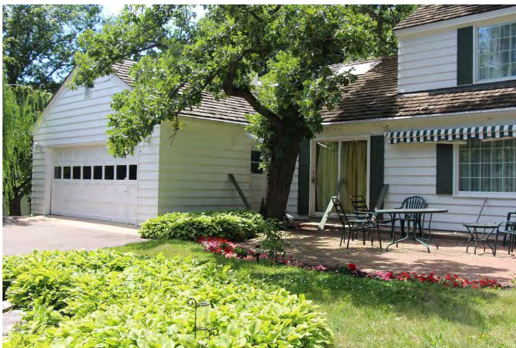
Figure 152. Overview of the attached garage on the front facade, view facing southwest.
