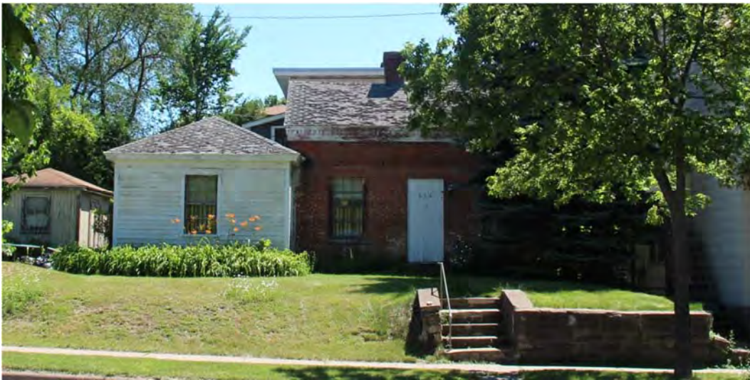
Front facade of the Adams House, view facing east.
