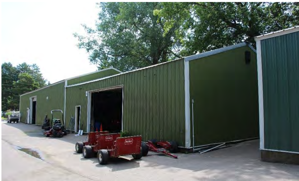
Figure 193. c.2005 and c.1987 maintenance buildings, view facing southeast.
