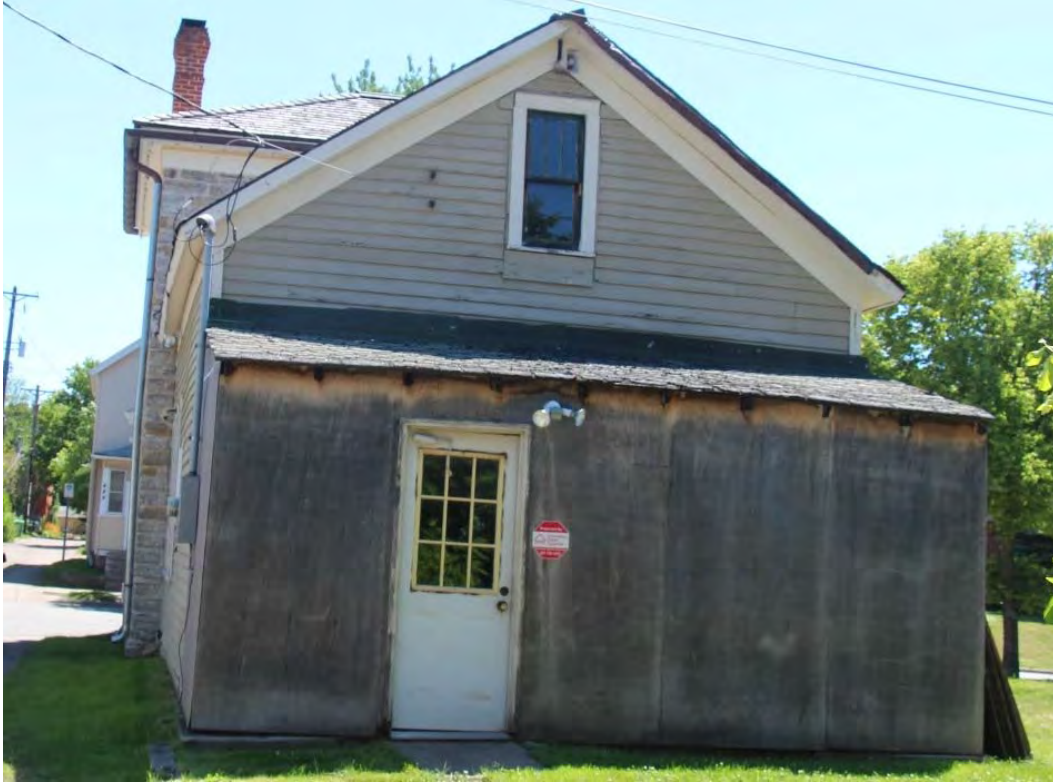
Rear (west) elevation, view facing east.
