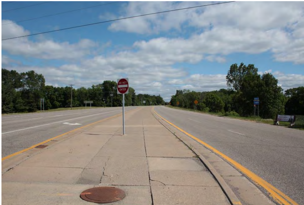
Figure 223. Dodd Road at Mendota Heights Road in Mendota Heights, view facing north.
