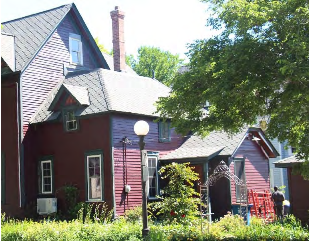
Rear (south) and side (west) elevations, view facing northeast.
