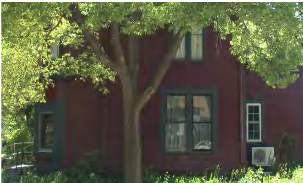
Figure 99. Side (west) elevation, view facing east.
