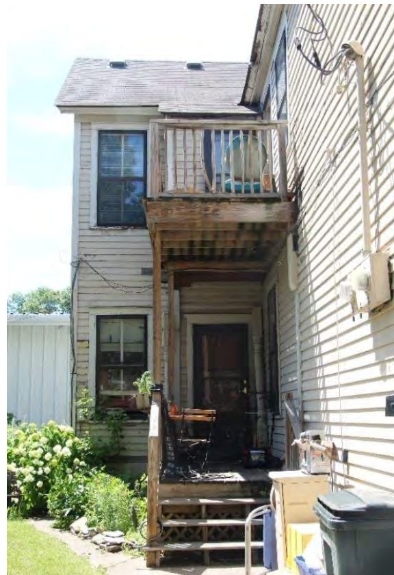
Figure 7. Detail of porch and upper balcony.
