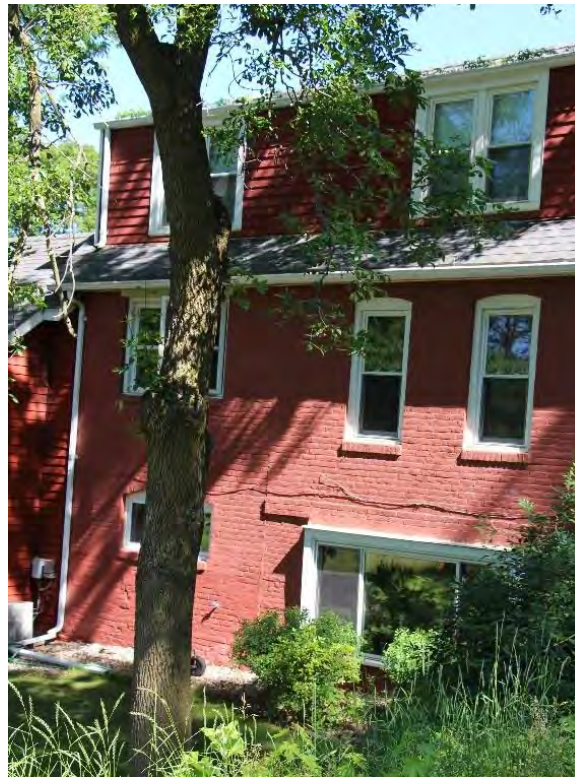
Figure 200. Side (south) elevation basement, view facing northwest.
