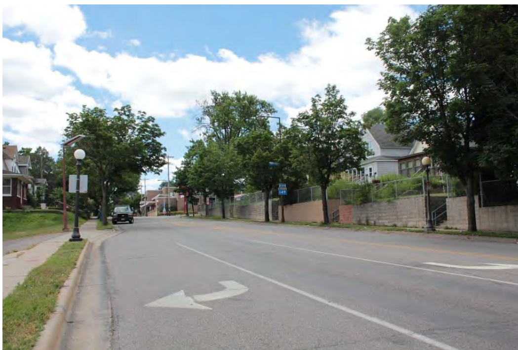
Figure 214. TH 149/Smith Avenue South at George Street, south of High Bridge, view facing south.
