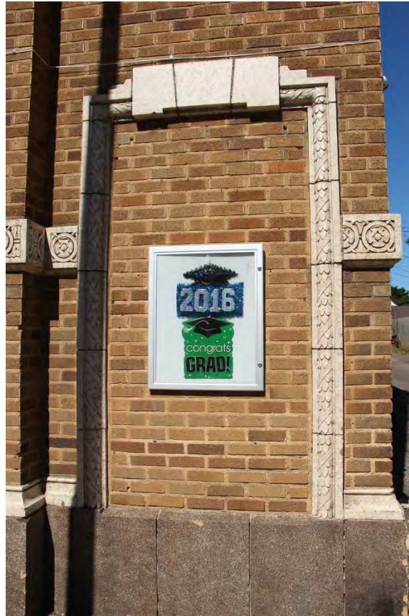
Figure 113. Detail of the original display frames with decorative terra cotta panels.
