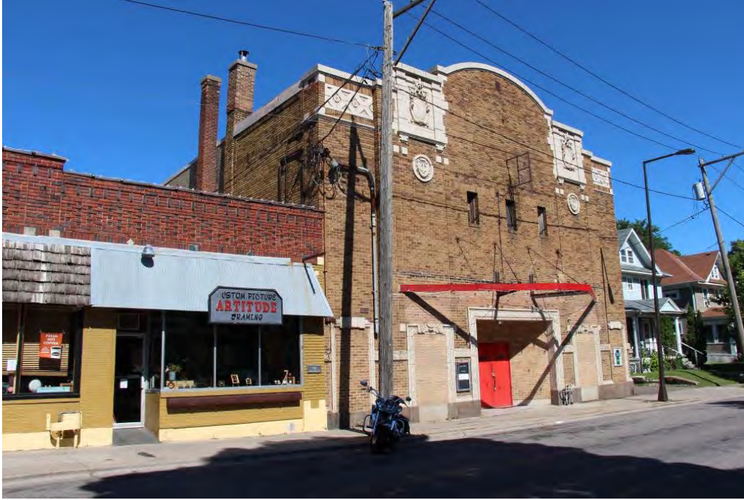
View of side (south) elevation and front (east) facade.
