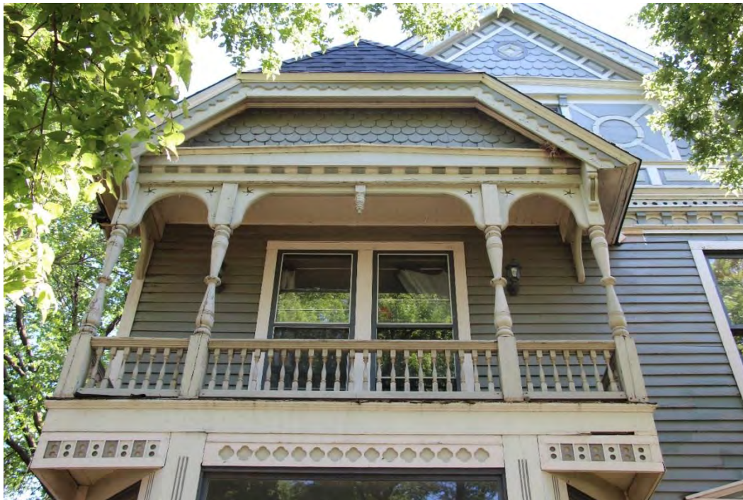
Figure 105. Detail of balcony at the Gardener House. Note the corner brackets and drop-bead detail, delicate balustrade, and details at the cutaway windows.
