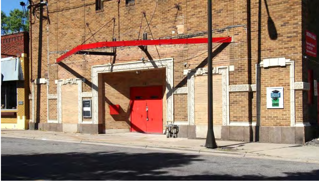
Figure 111. Street level of the front (east) facade. Note the mid-twentieth-century steel marquee, which replaced the original flat roof projecting entryway canopy, over the altered primary entry.
