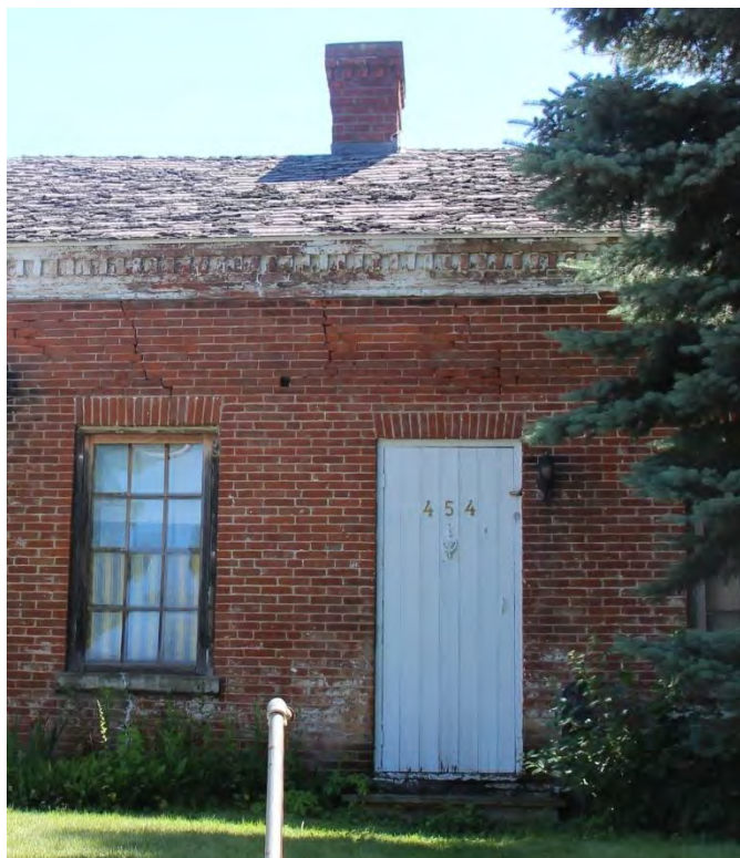
Figure 66. Detail of front (west) facade entrance. Note the dentil detail on the cornice.
