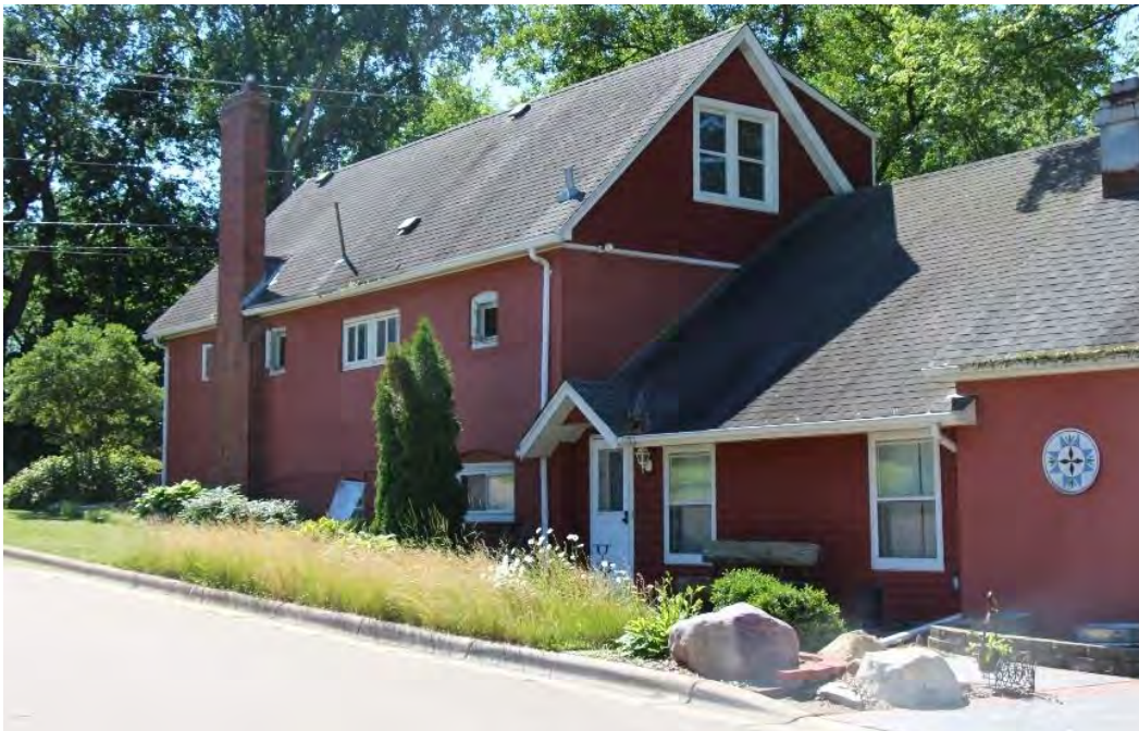
Figure 202. Side (north) and rear (west) elevations, view facing northeast.
