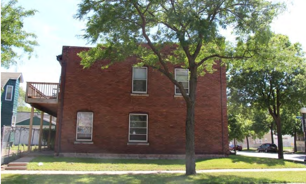
Figure 25. North elevation of the Johnson Building, view facing south.
