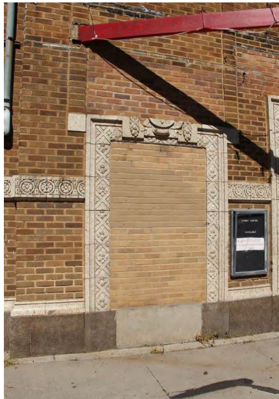
Figure 112. Detail of the altered doorway including removal of the original terra cotta door hood. Note the various terra cotta ornamental panels around the door and extending horizontally across the facade.
