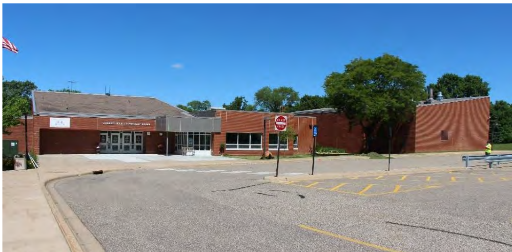
Figure 169. 1969 and 2016 additions, facing west.
