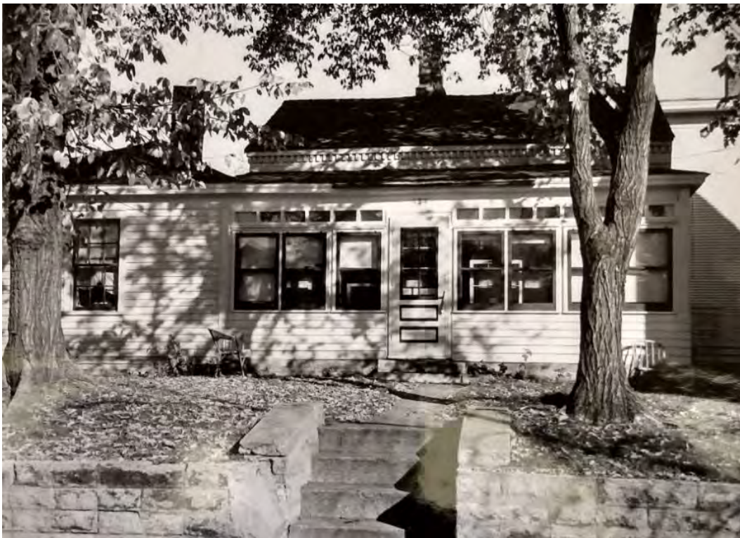
Figure 74. 1961 image of Adams House with the enclosed late-nineteenth-century porch. 138
