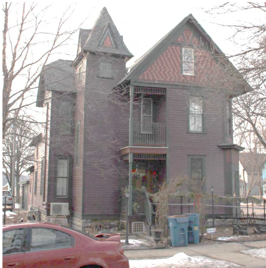
Figure 97. Front (north) facade and side (east) elevation, view facing southwest.
