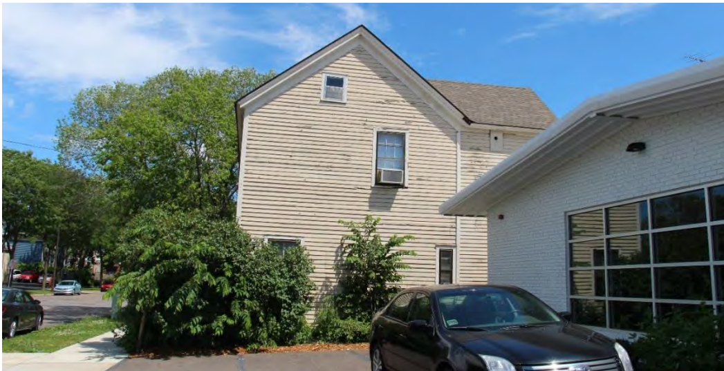
Figure 9. Side (west) elevation, view facing east.
