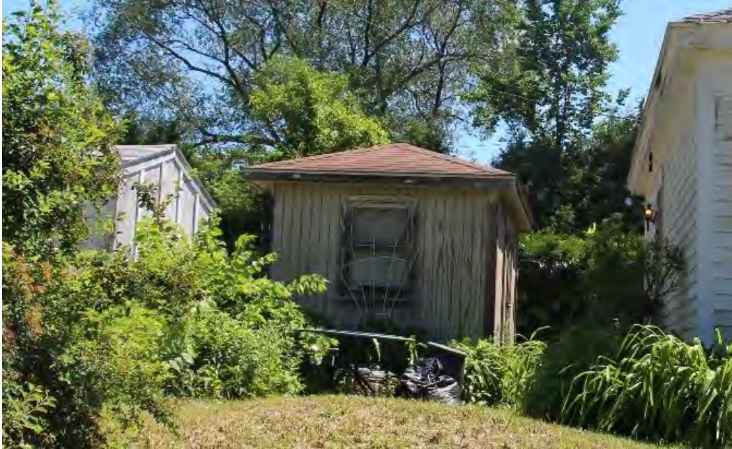
Figure 71. West elevation of shed, view facing east.
