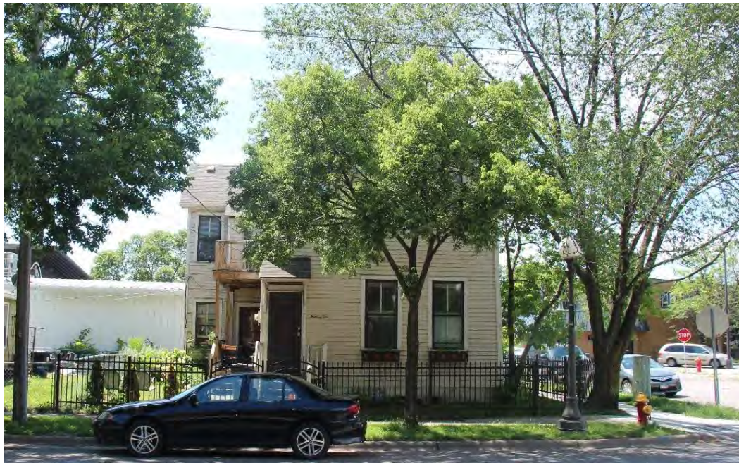
Figure 4. Front (east) facade, view facing west.
