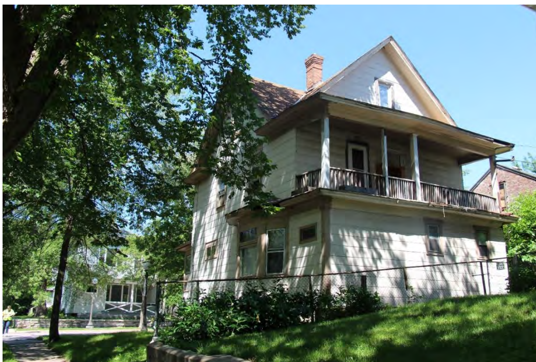
Figure 82. Rear (back) elevation, view facing northwest.
