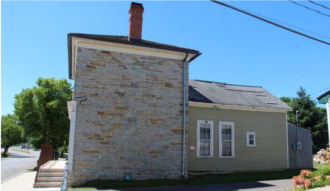
Side (north) elevation, view facing south.
