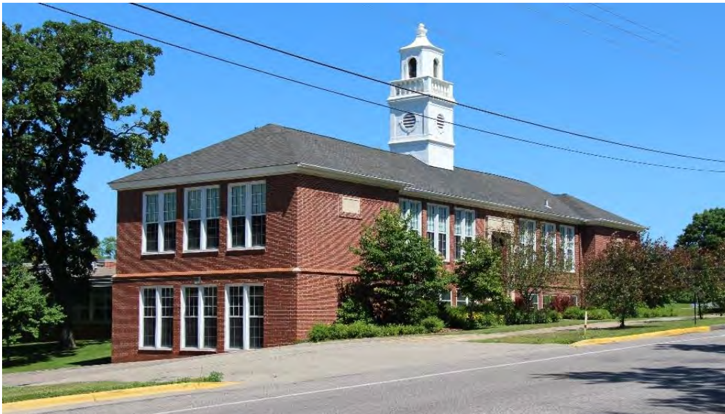
Figure 161. 1936 school building, facing northwest. Note replacements windows.
