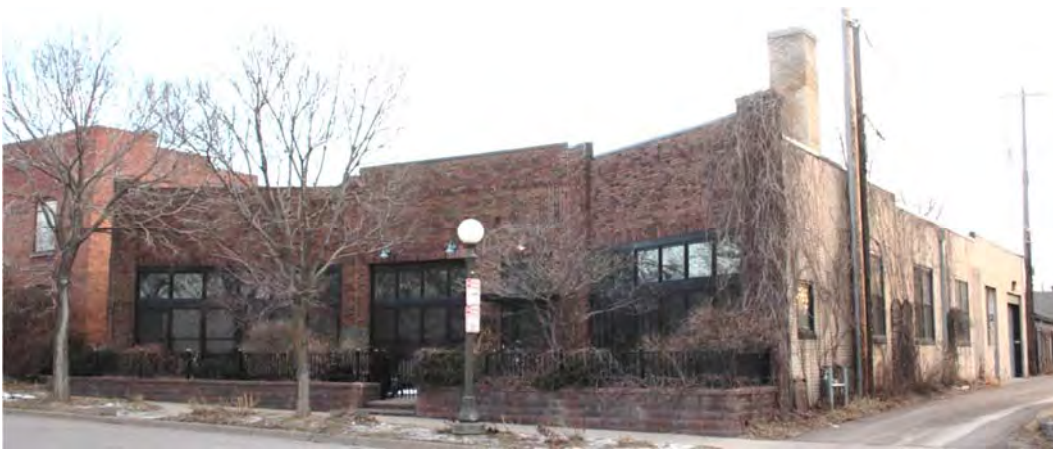
Front (west) facade and side (south) elevation, view facing northeast.
