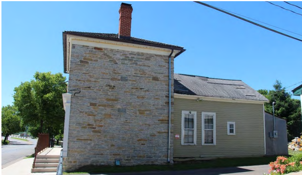
Figure 47. Side (north) elevation, view facing south.
