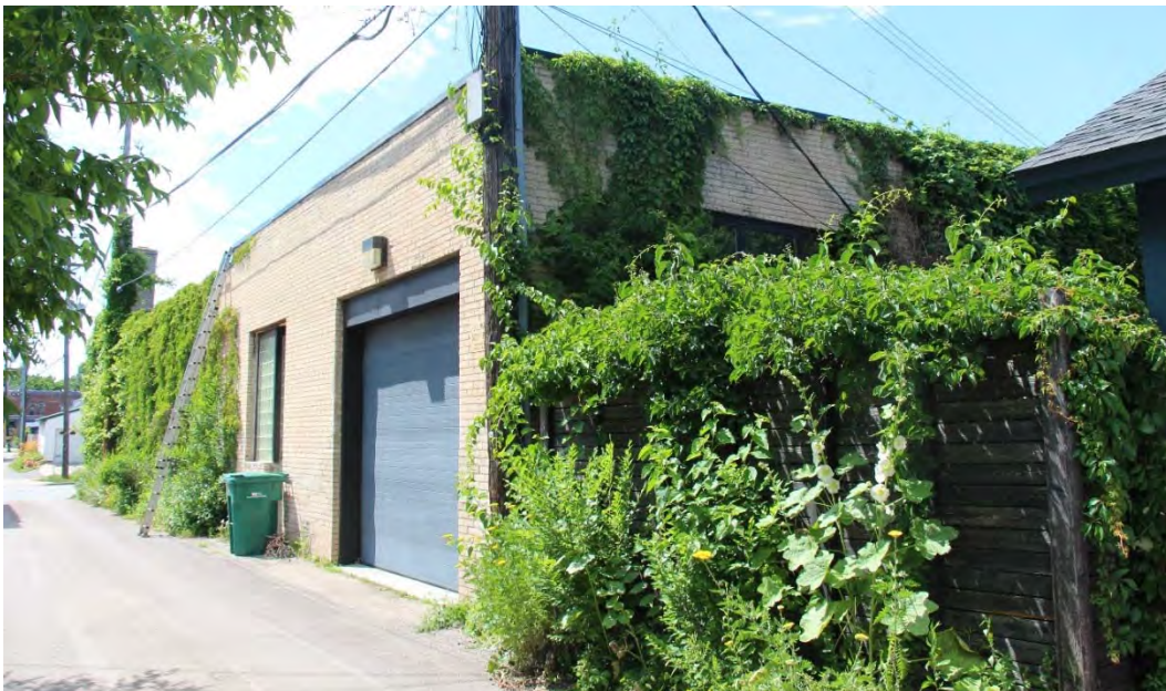
Side (south) and rear (east) elevations, view facing northwest. Note the multi-pane window visible above the fence.
