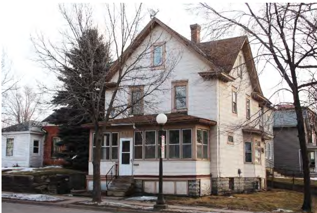
Figure 76. Front (west) facade and side (south) elevation of the Haag House, view facing northeast.
