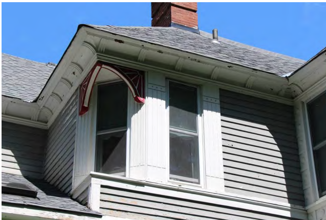
Figure 132. Detail of cornice decorative details and brackets.
