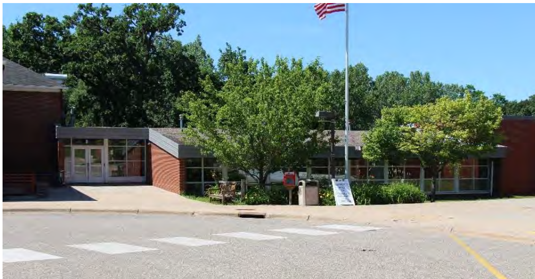
Figure 167. Northeast elevation of the 1953 addition and hyphen.
