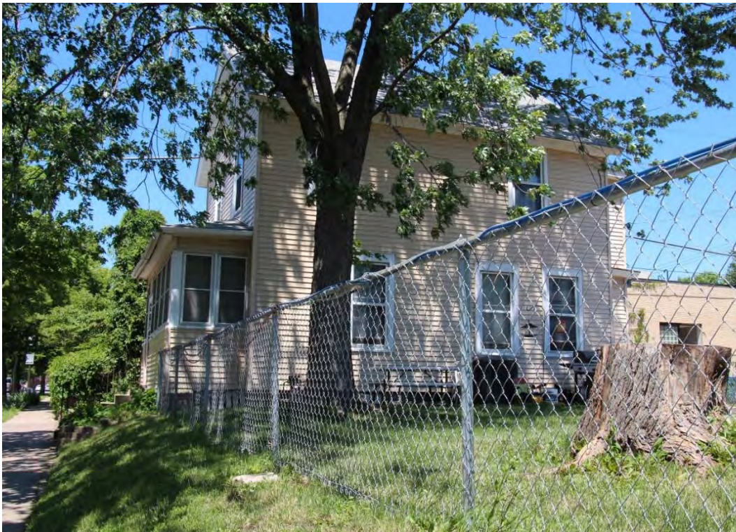
Side (south) elevation, view facing northeast.
