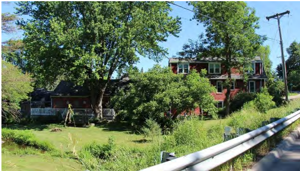
Figure 198. Side (south) elevation, yard, and drainage pond, view facing north.
