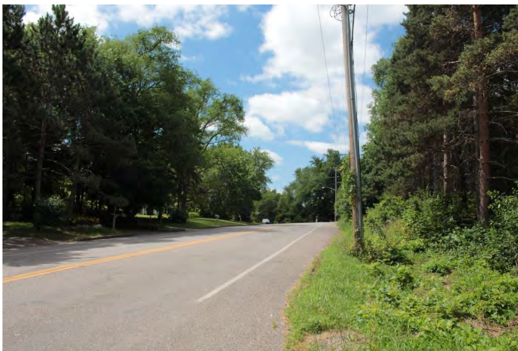
Figure 219. Dodd Road at Spring Creek Circle in Mendota Heights, view facing southeast.
