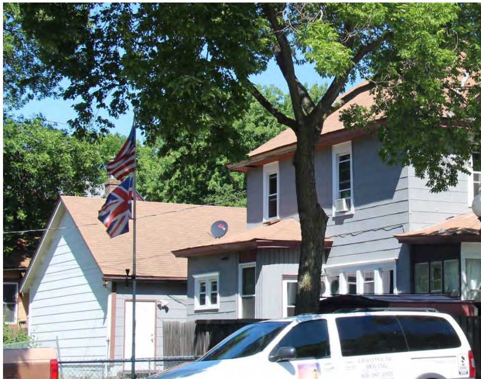
Side (south) elevation, view facing northwest.
