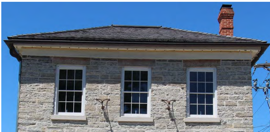
Figure 45. Detail of second-story windows on the front (east) facade.
