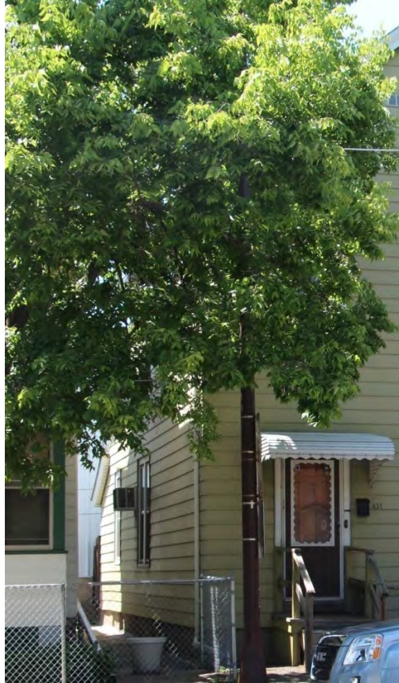
Side (south) elevation, view facing northwest.
