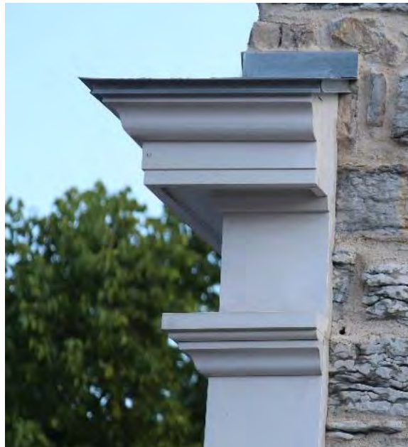
Figure 44. Detail of molding profile of friezeboard and corner pilaster.
