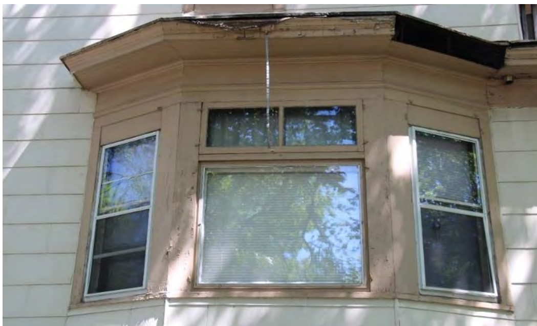
Figure 81. Detail of bay, view facing north.
