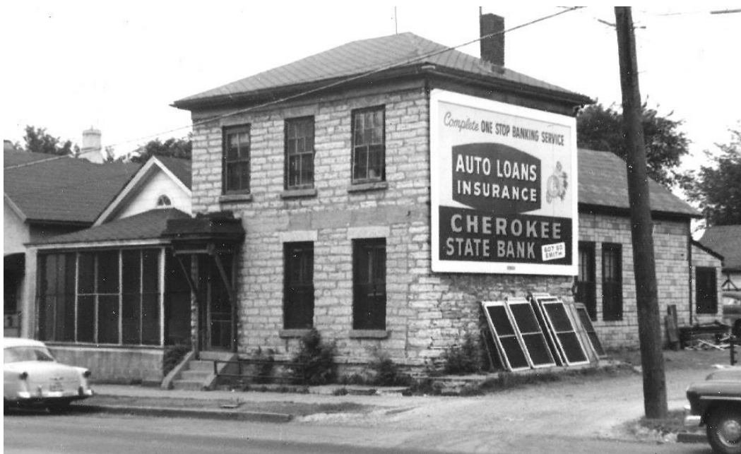
Figure 52. c.1960 photograph of the Waldman Saloon with the residential facade and blank north elevation utilized for advertising. 89
