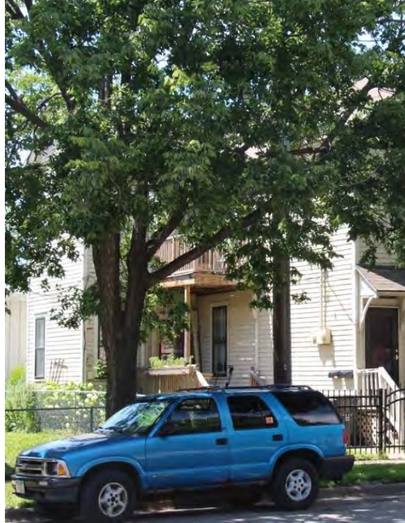
Side (south) elevation, view facing northwest.
