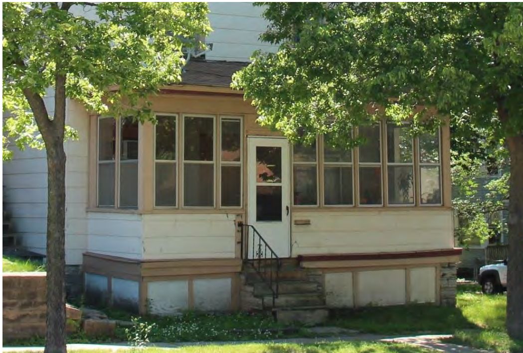
Figure 77. Detail of enclosed porch on front (west) facade, view facing southeast.
