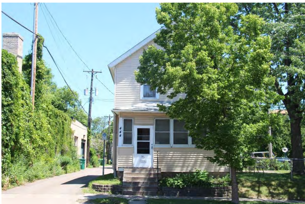
Figure 57. Front (west) facade, view facing east.
