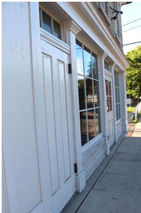
Figure 43. Detail of restored storefront, view facing northwest.
