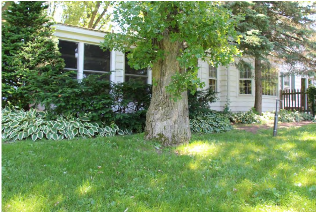
Figure 155. Overview of enclosed porch on the side elevation, view facing southeast.
