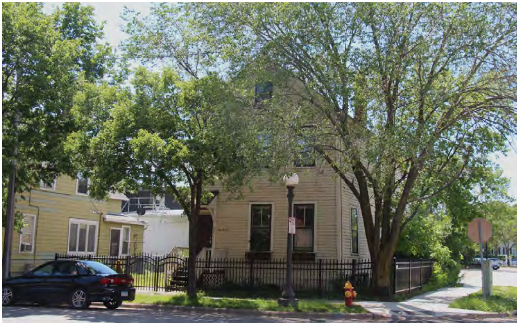
Figure 3. Front (east) facade and side (north) elevation of 425 Smith Avenue North, view facing southwest.
