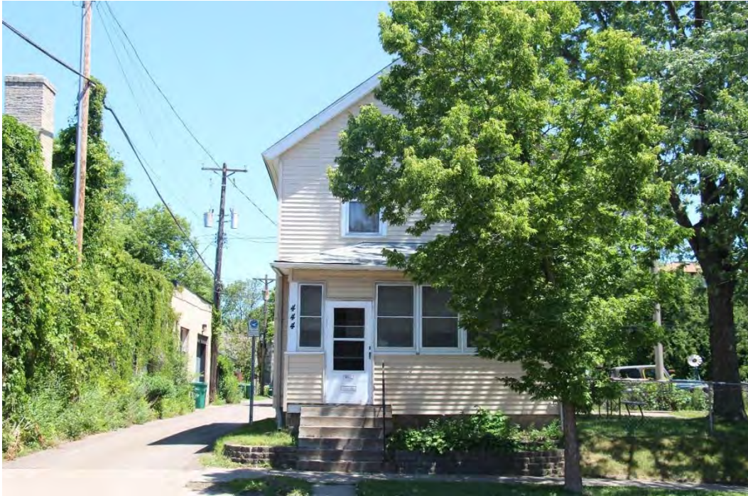
Front (west) facade, view facing east.
