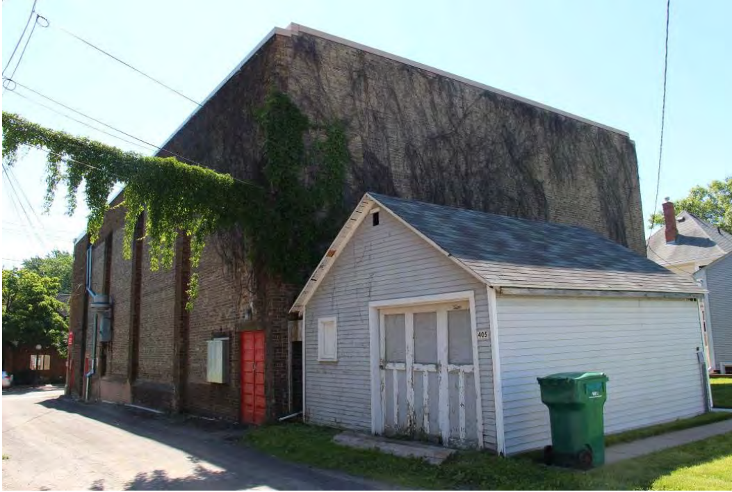
View of rear (west) elevation.
