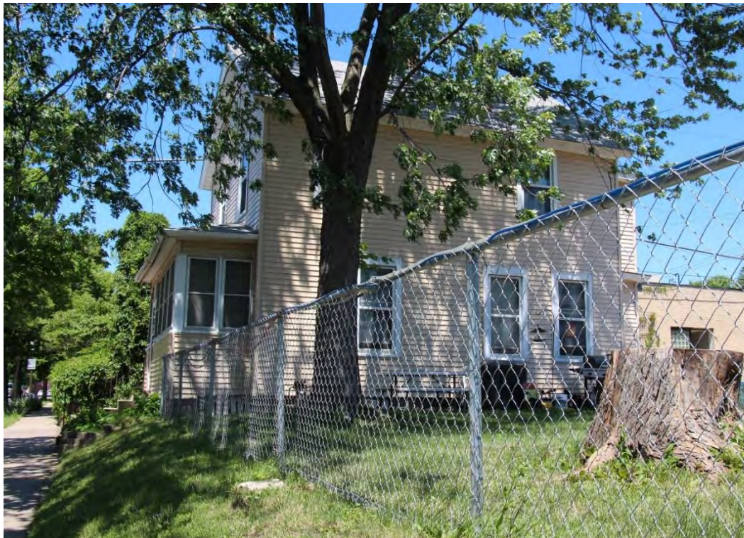
Figure 59. Side (south) elevation, view facing northeast.
