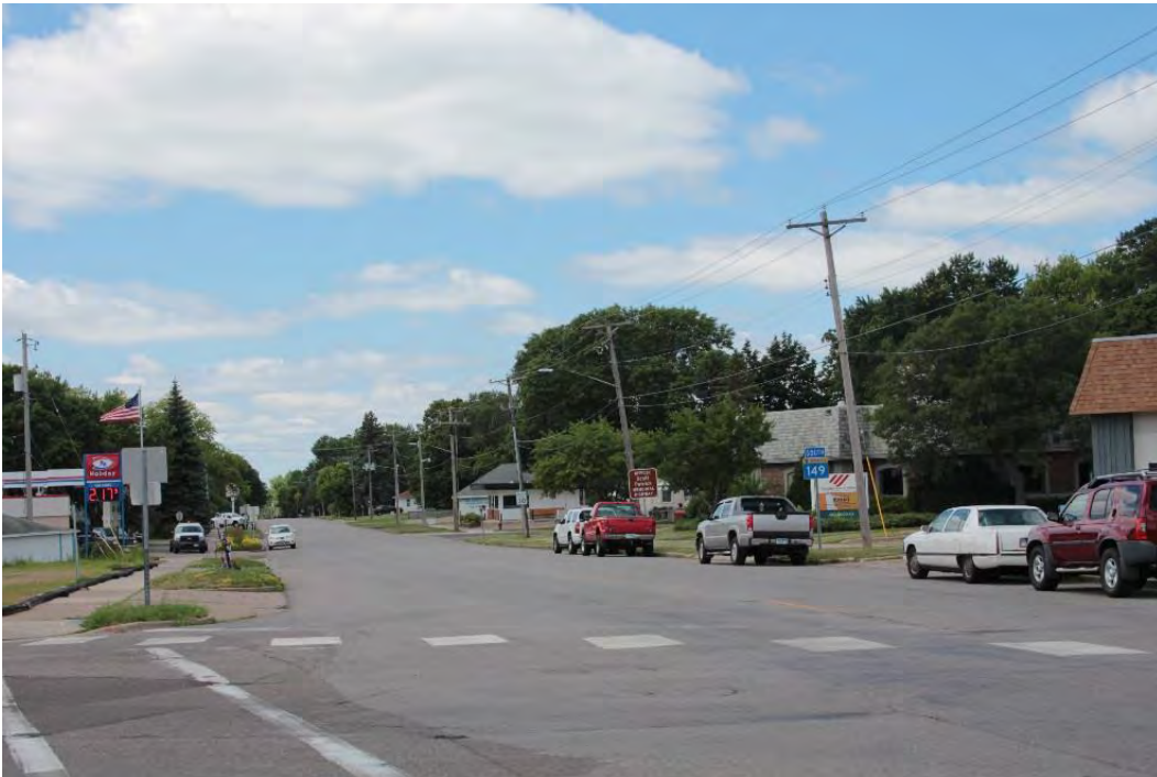
TH 149, intersection of Smith Avenue and Dodd Road, view facing southwest along Dodd Road.
