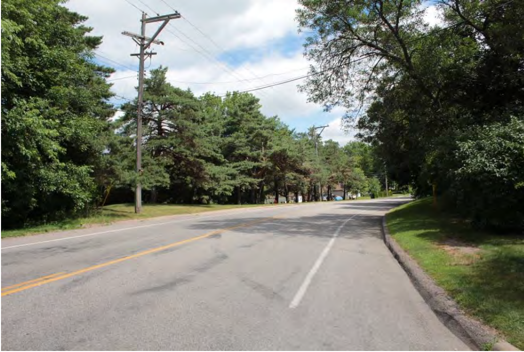
TH 149/Dodd Road at Mears Avenue in Mendota Heights, view facing north.
