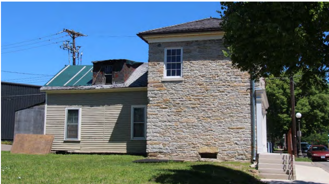
Side (south) elevation, view facing north.
