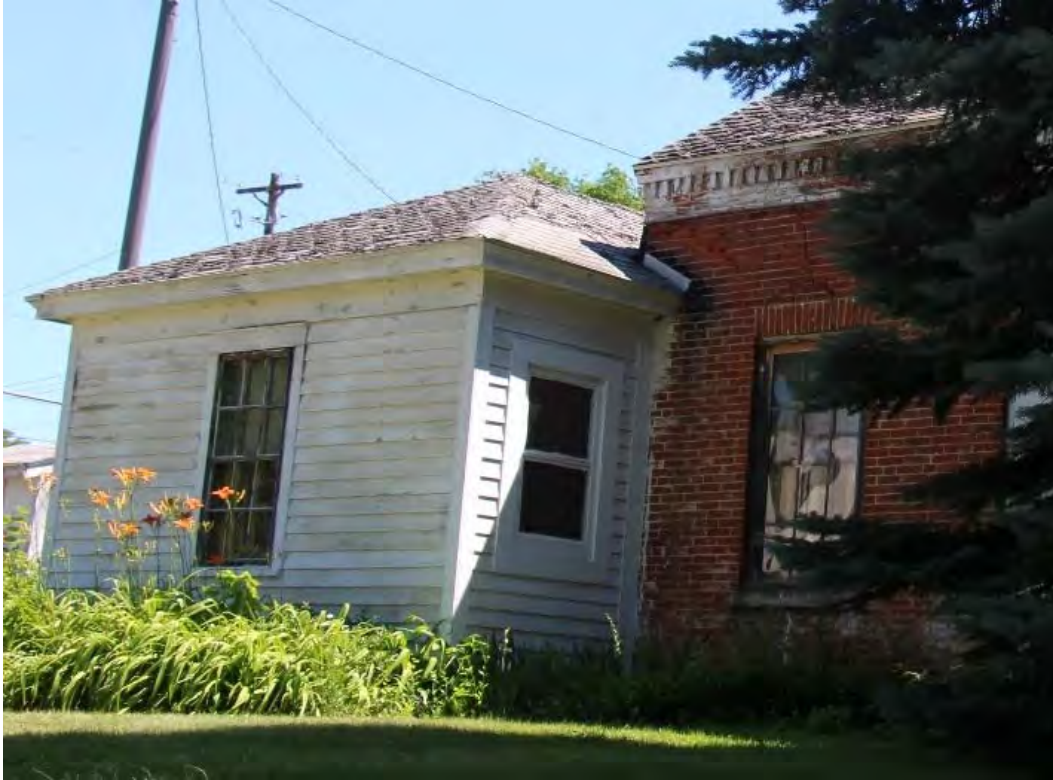
Addition on north elevation, view facing northeast.
