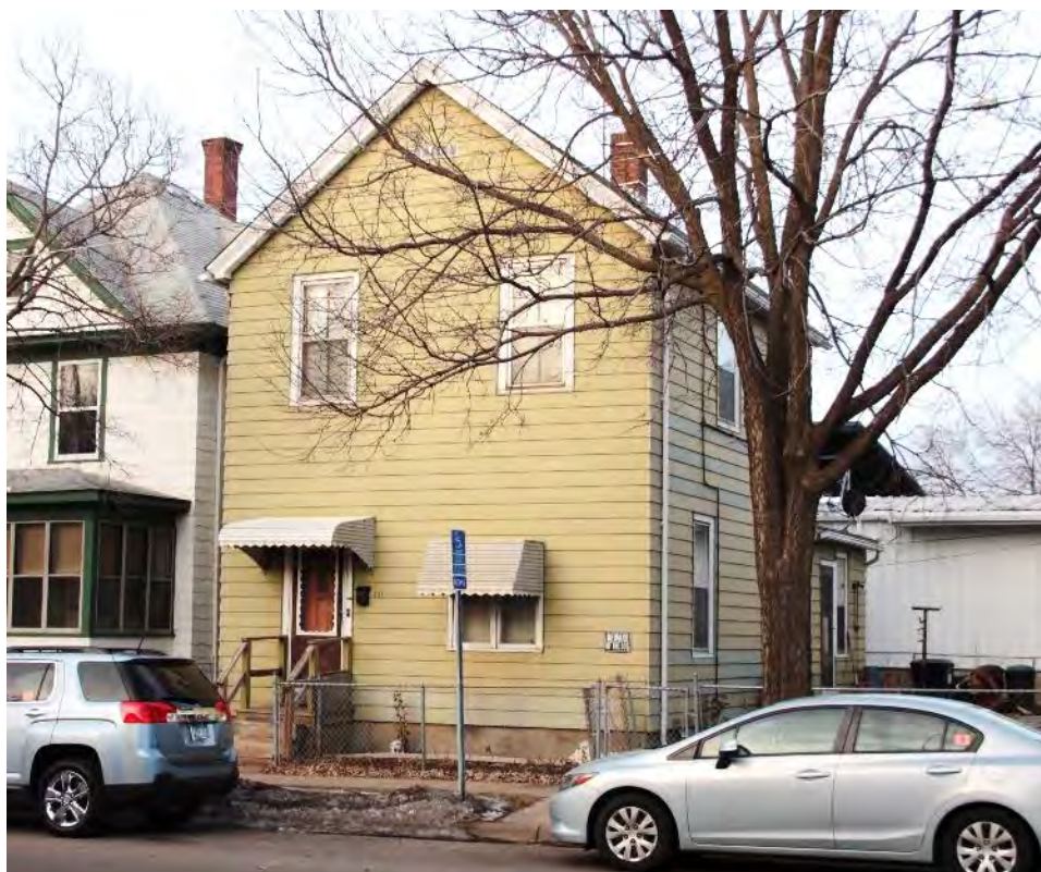
Figure 15. Front (east) facade and side (north) elevation of 431 Smith Avenue North, view facing southwest.
