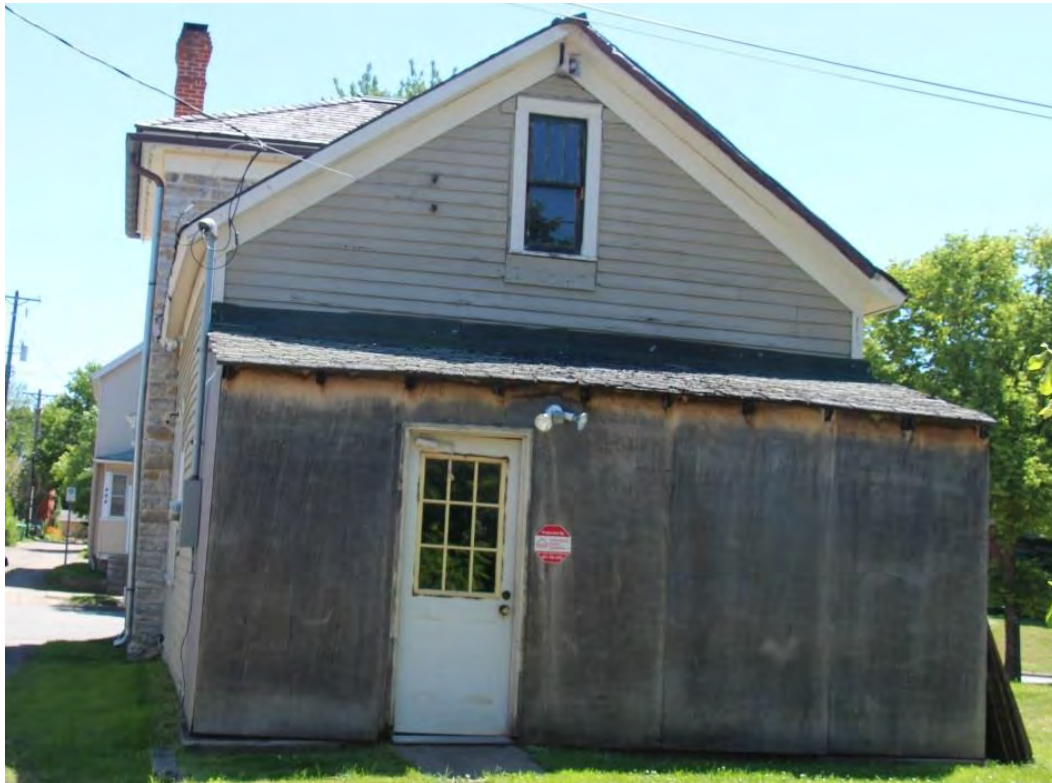
Figure 51. Rear (west) elevation, view facing east.
