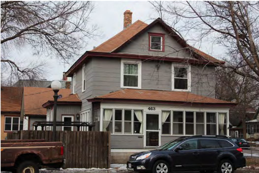
Front (east) facade, view facing west.
