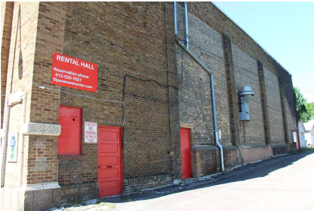
Figure 115. View of side (north) elevation.
