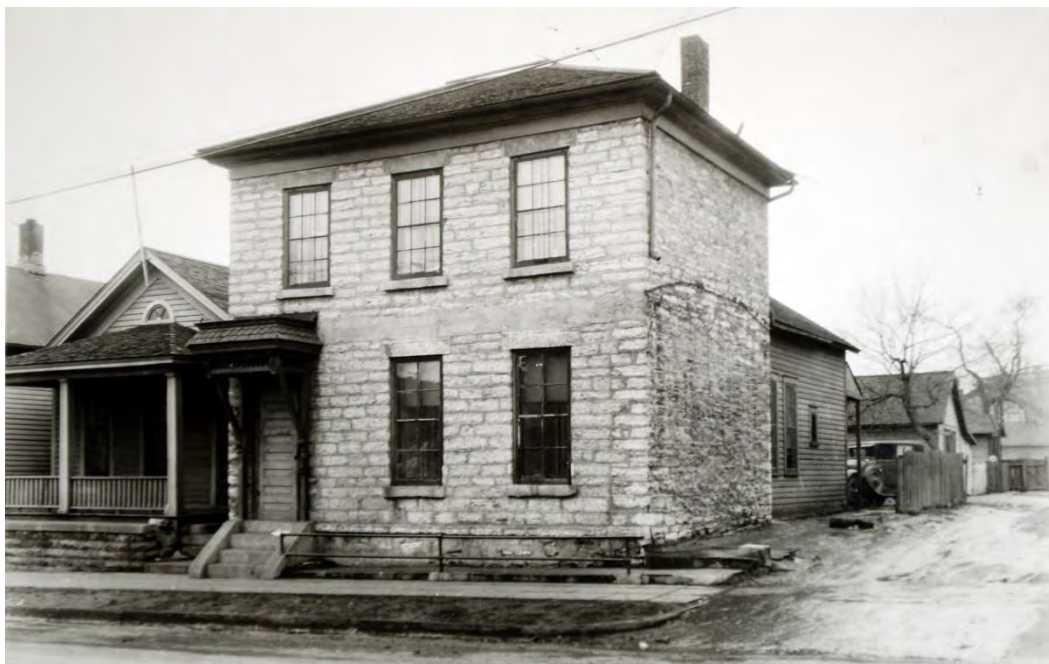
Figure 46. A 1936 photograph of the Waldman Saloon showing six-over-six, double-hung, sash windows on the second story of the front (east) facade. 85 Note the ghost image of a one-story hip-roofline on the side (north) elevation that indicates a lean-to shed was once located here that extended towards the alley.
