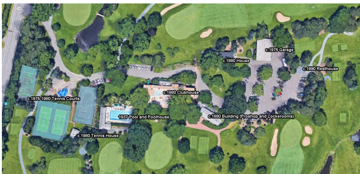
Figure 176. Somerset Country Club central group of buildings. 269
