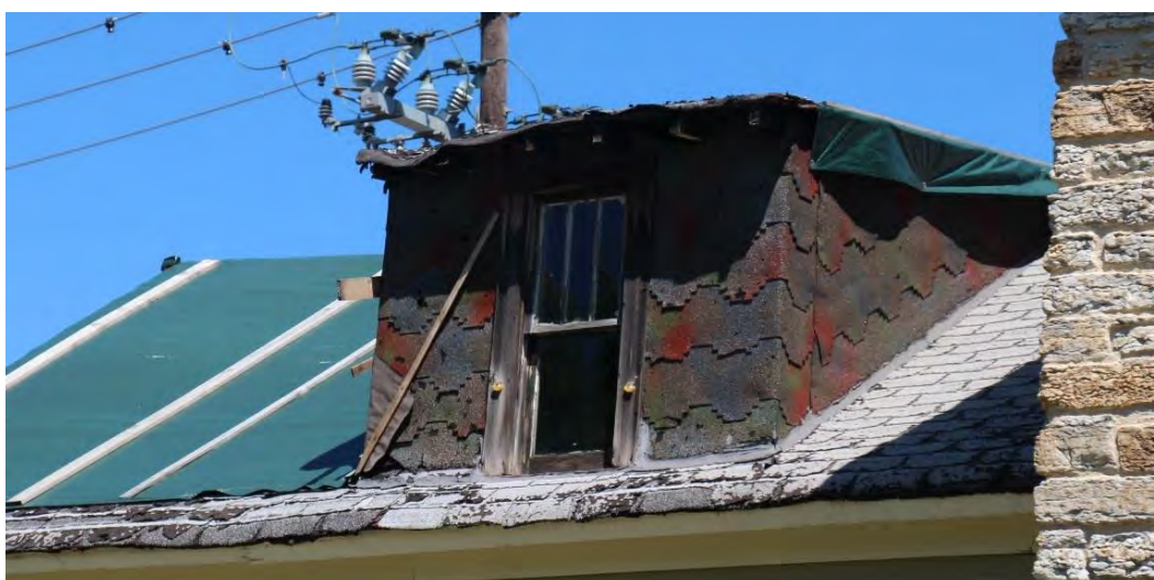
Figure 50. Detail of shed roof dormer on side (south) elevation, view facing northwest.
