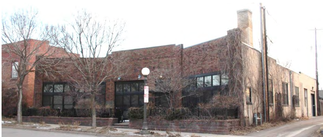
Figure 35. Front (west) facade and side (south) elevation, view facing northeast.
