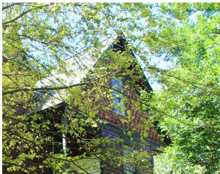
Figure 98. Detail of tower at northeast corner. Note the gable detail over the fixed window.
