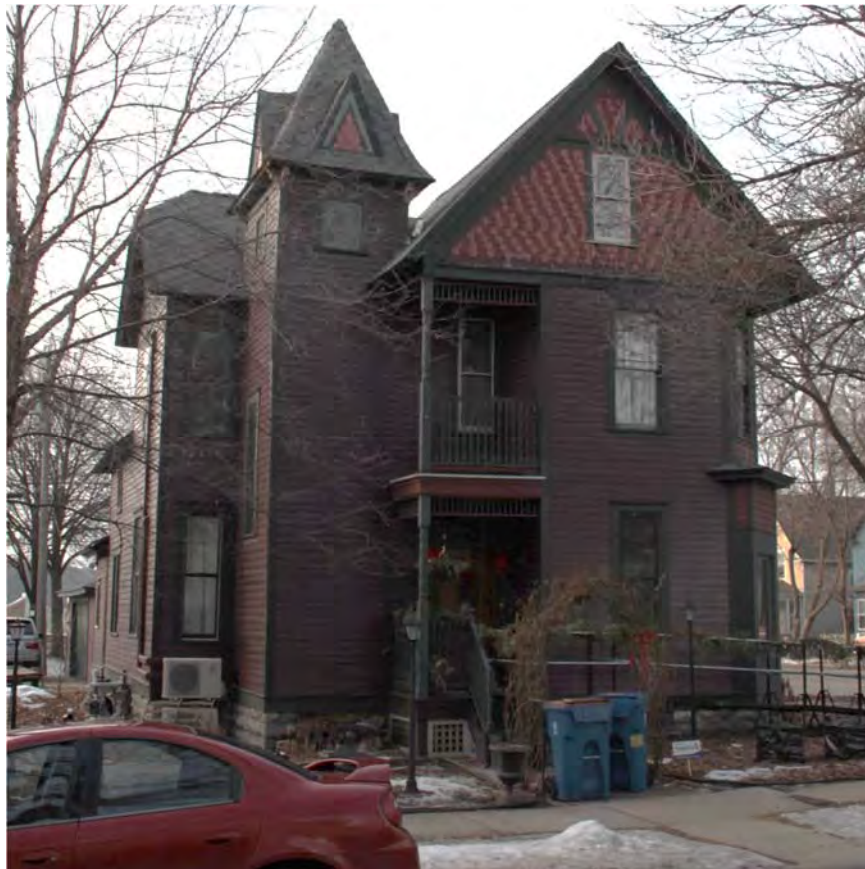
Front (north) facade and side (east) elevation, view facing southwest.
