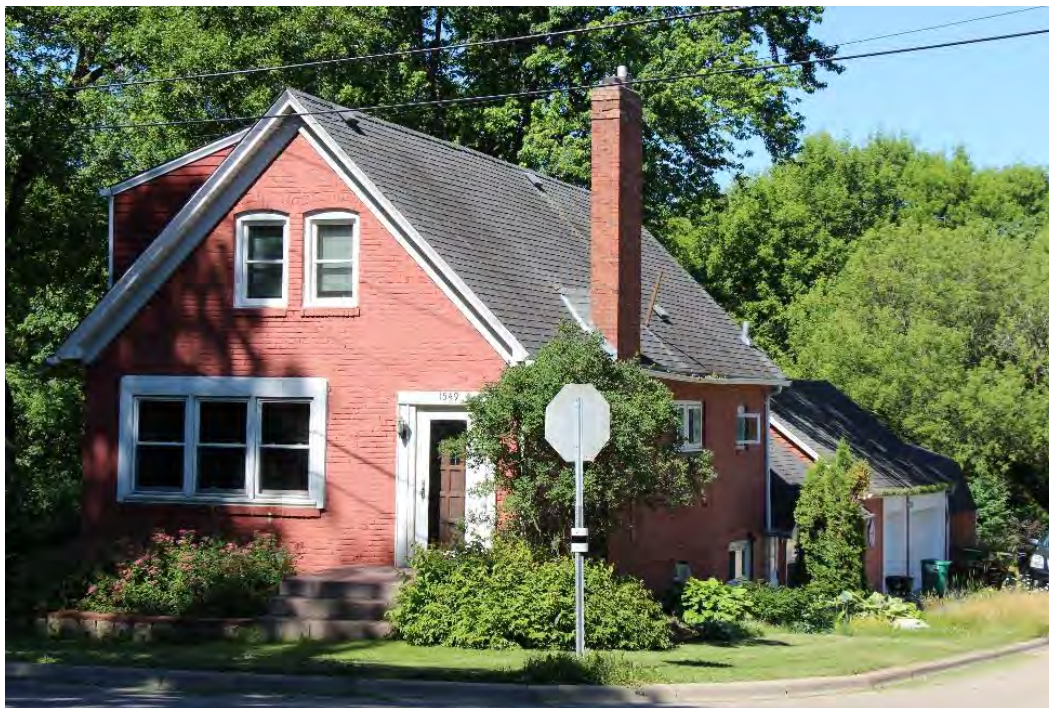
Figure 197. Front (east) facade and side (north) elevation of the house at 1549 Dodd Road, view facing southwest.
