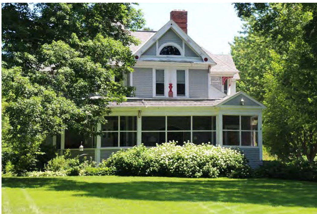
Figure 134. Front (northwest) facade, view facing southeast.
