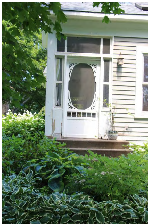
Figure 136. Concrete steps located at the northwest corner of the porch and decorative screen door.
