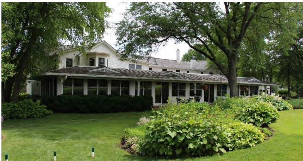
Figure 181. c.1880 clubhouse and 1980 dining room addition, view facing northeast.
