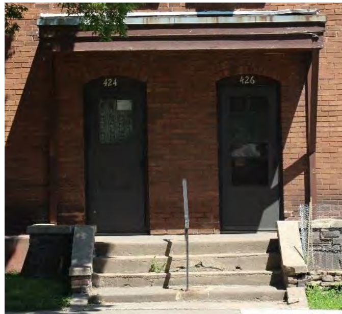
Figure 24. Detail of Johnson Building entrance, units 424 and 426.
