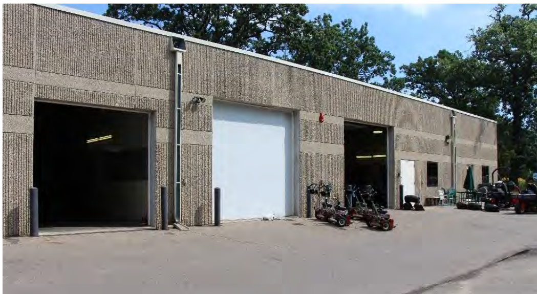
Figure 192. c.2005 maintenance building, view facing northeast.
