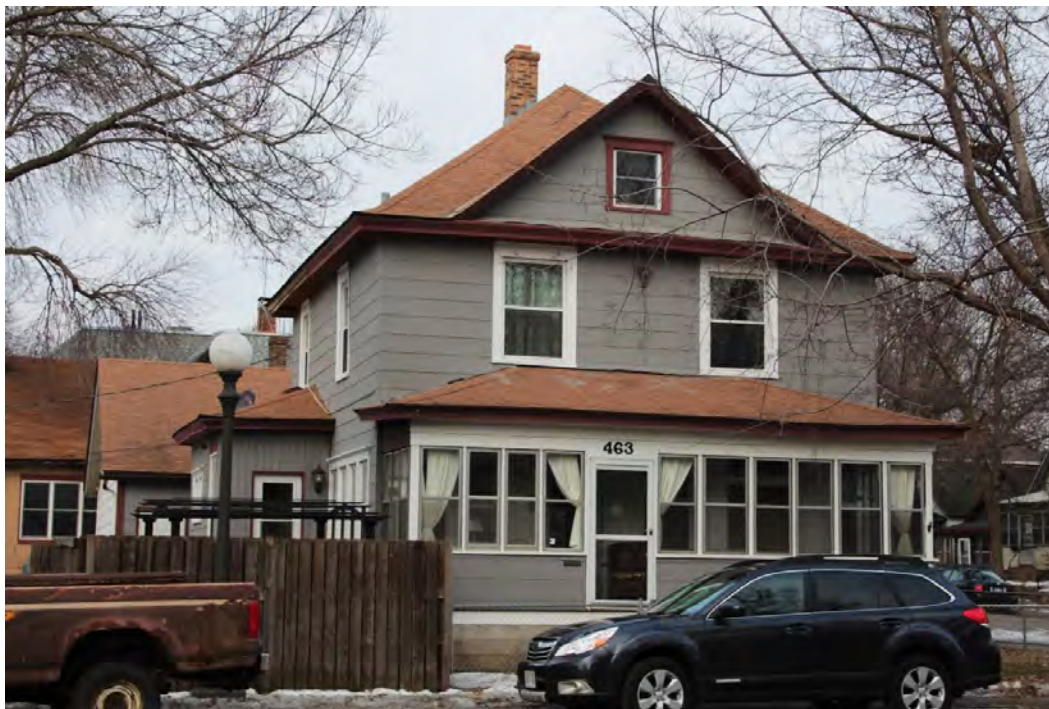
Figure 87. Front (east) facade, view facing west.
