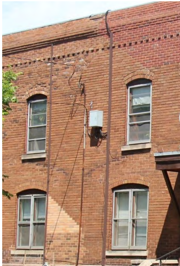
Figure 28. Detail of front (west) facade of the Johnson Building showing areas of brick repair. Note the variation in brick color used.
