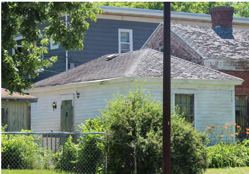
Figure 69. Side (north) elevation, view facing southeast.
