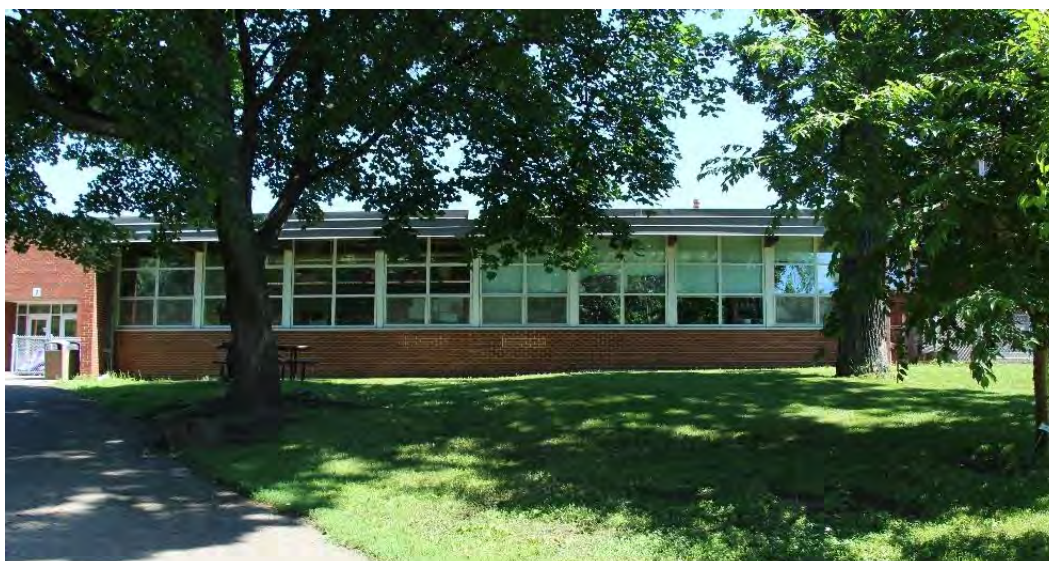
Figure 168. Southwest elevation of the 1953 addition.
