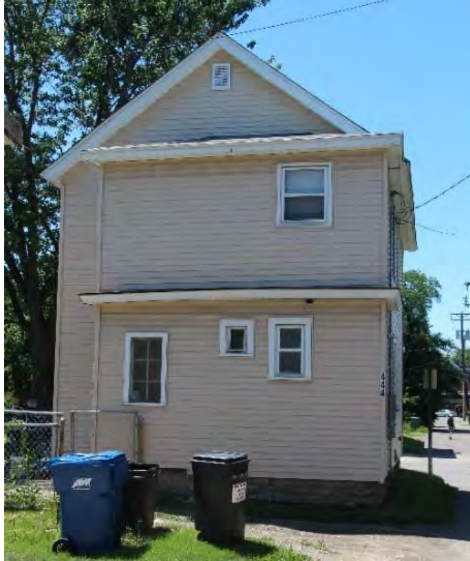
Rear (east) elevation, view facing west.
