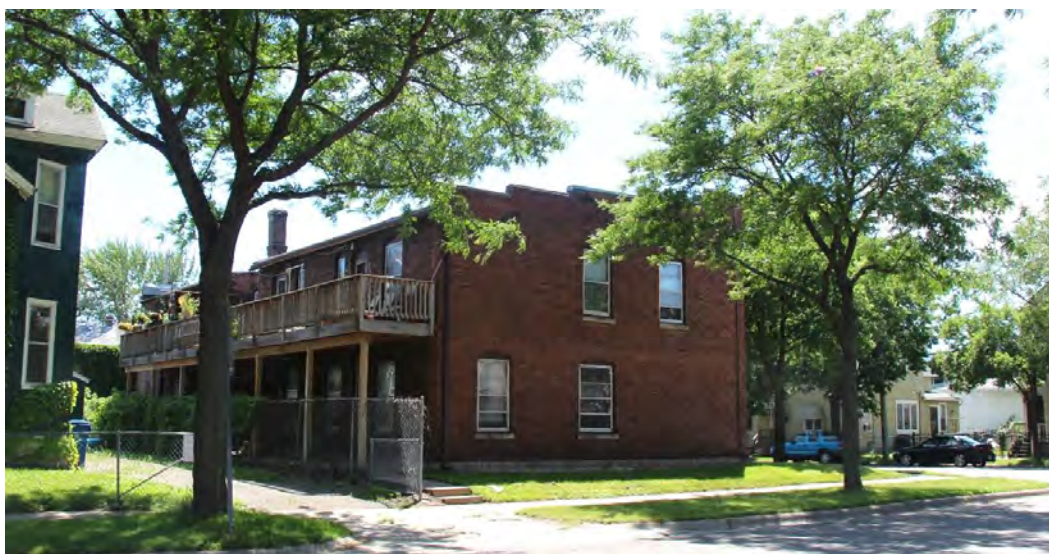
Figure 27. Rear (east) elevation of the Johnson Building, view facing southwest.
