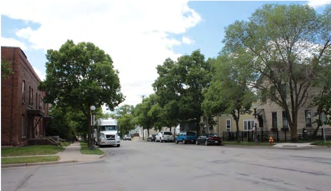
TH 149/Smith Avenue North just south of intersection with W. 7 th Street, view facing south.
