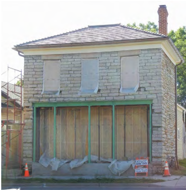
Figure 54. Front (east) facade under renovation in 2014. Photograph courtesy of property owner Tom Schroeder.
