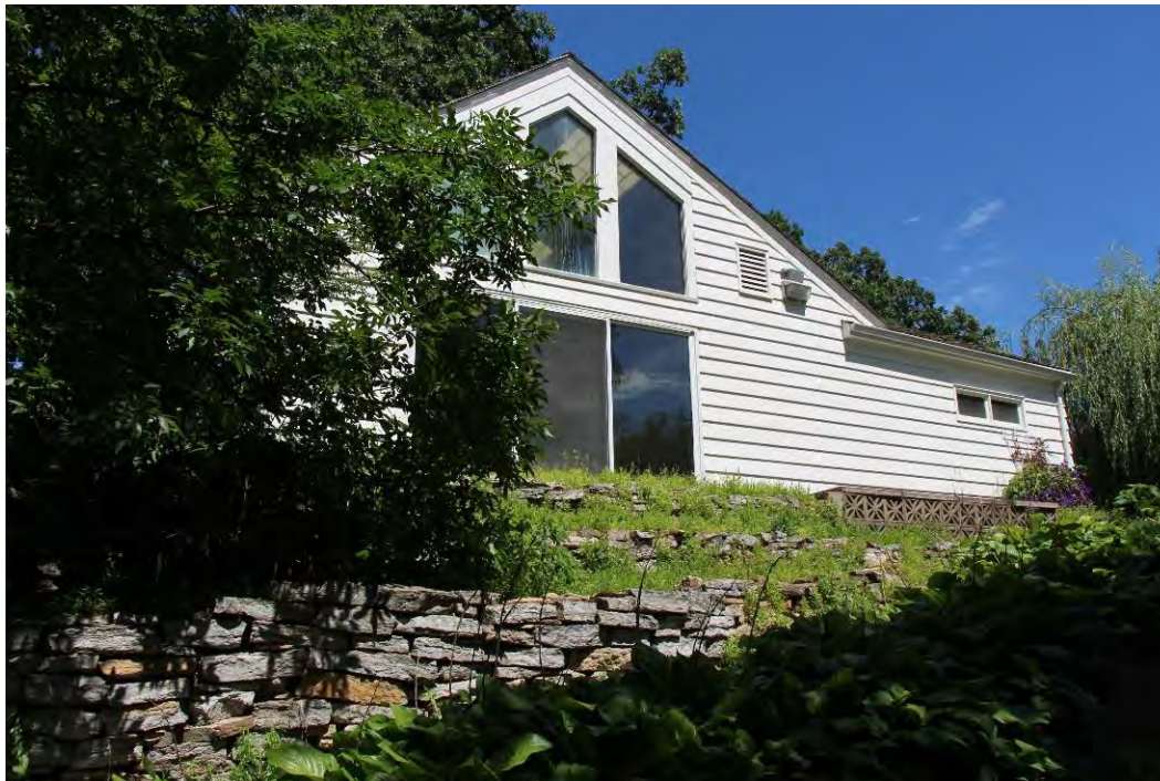
Figure 157. Overview of the side (south) elevation with attached garage, view facing northeast.
