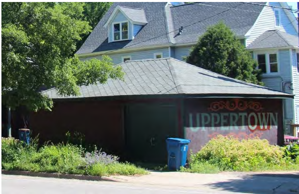
Figure 102. Detached garage, view facing northeast.
