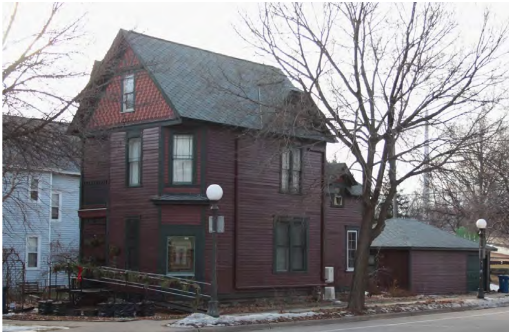
Figure 96. Front (north) facade and side (west) elevation, view facing southeast.
