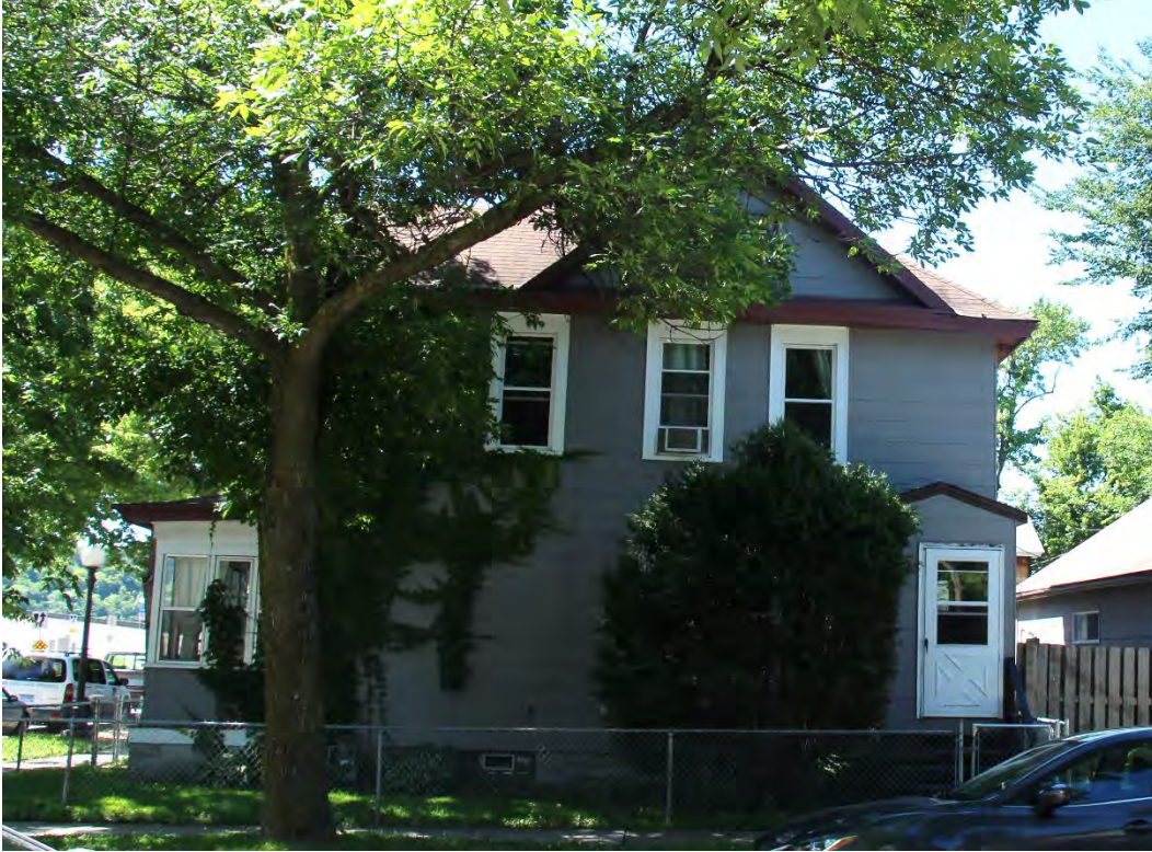
Figure 88. Side (north) elevation, view facing south. Note how the vegetation obscures architectural details of the house.
