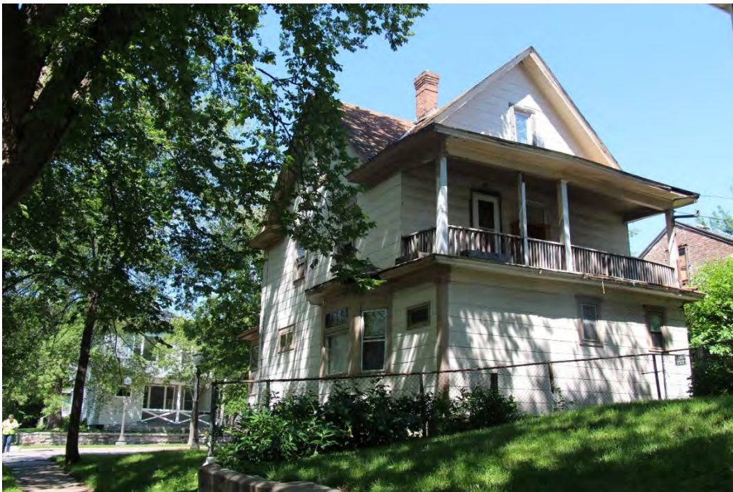
Rear (back) elevation, view facing northwest.
