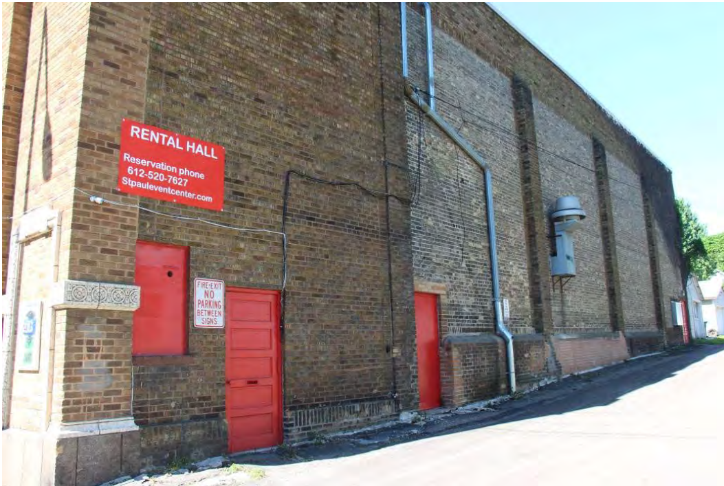
View of side (north) elevation.
