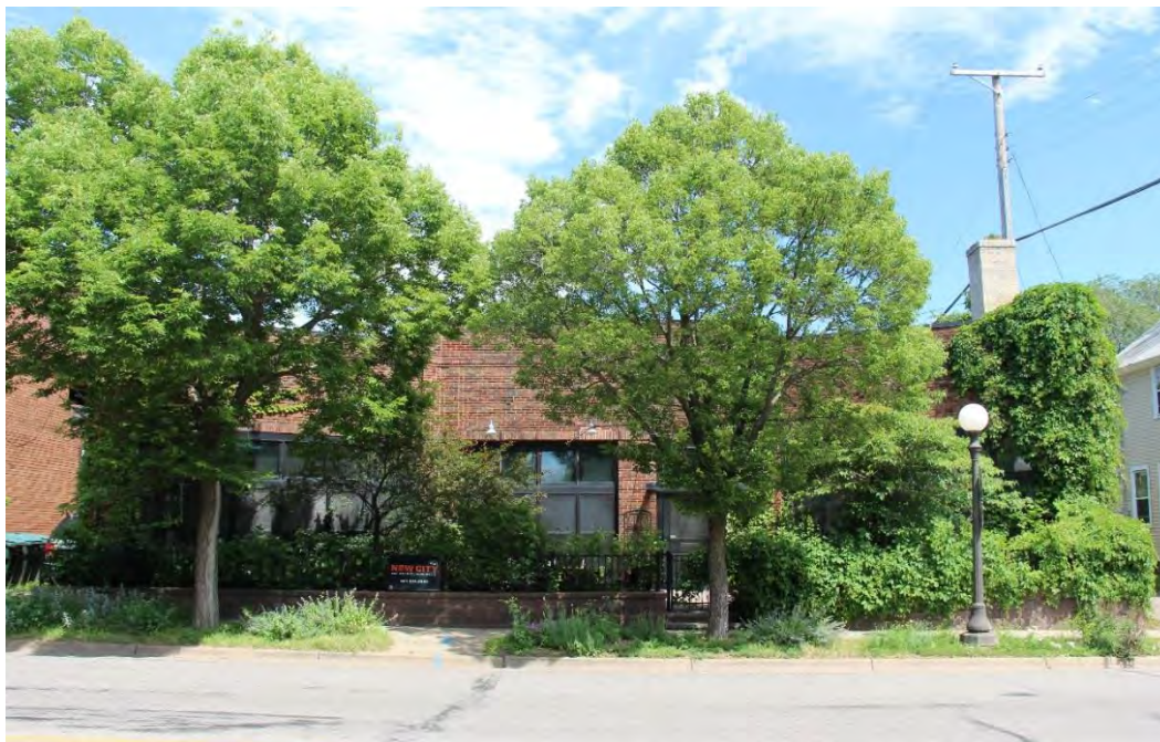
Figure 32. Front (west) facade, view facing east. Note the ivy obscuring architectural details at the corners of the building.
