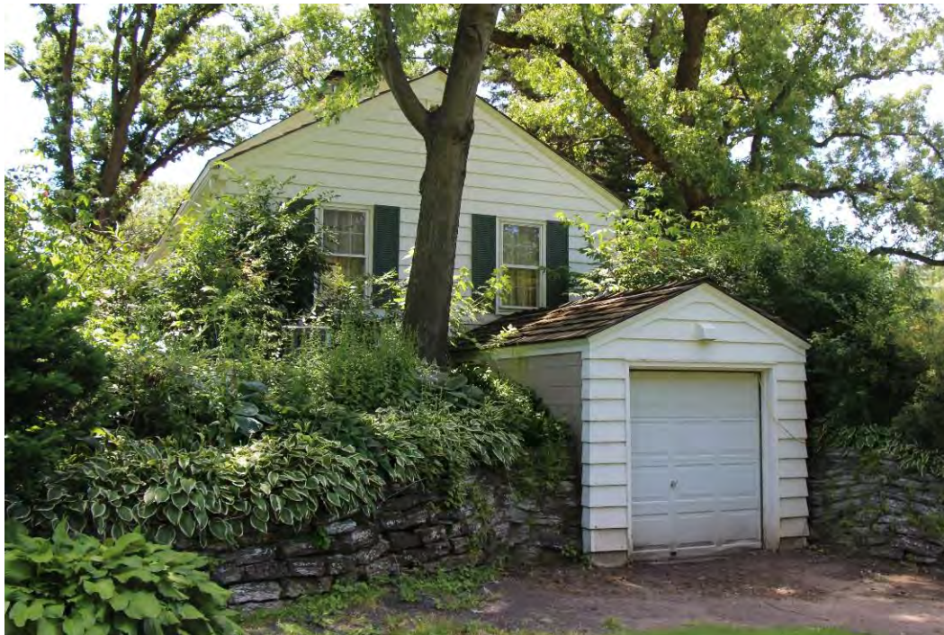
Figure 150. Single-bay garage attached at the side (north) elevation, view facing southwest.
