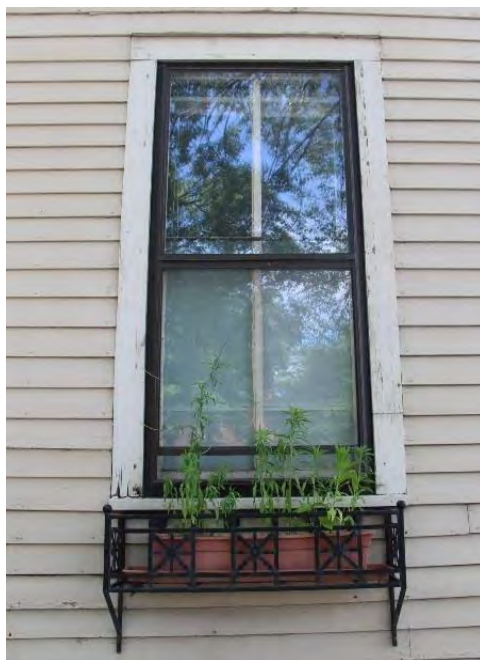
Figure 5. Detail of window on front (east) facade.
