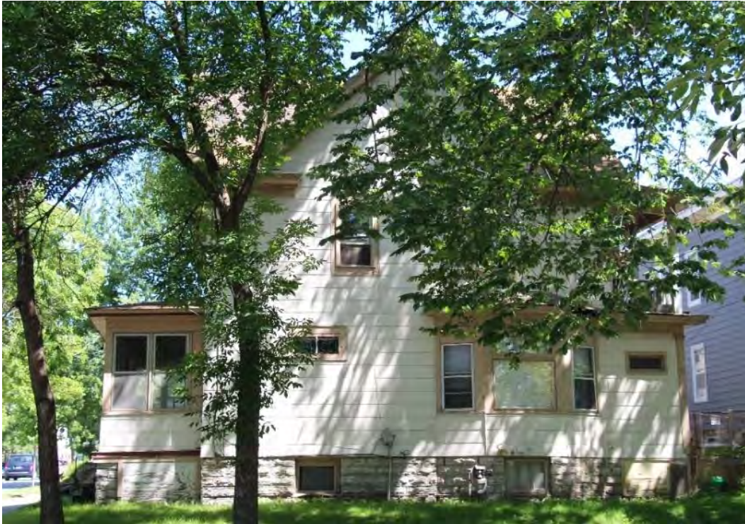
Side (south) elevation, view facing north.
