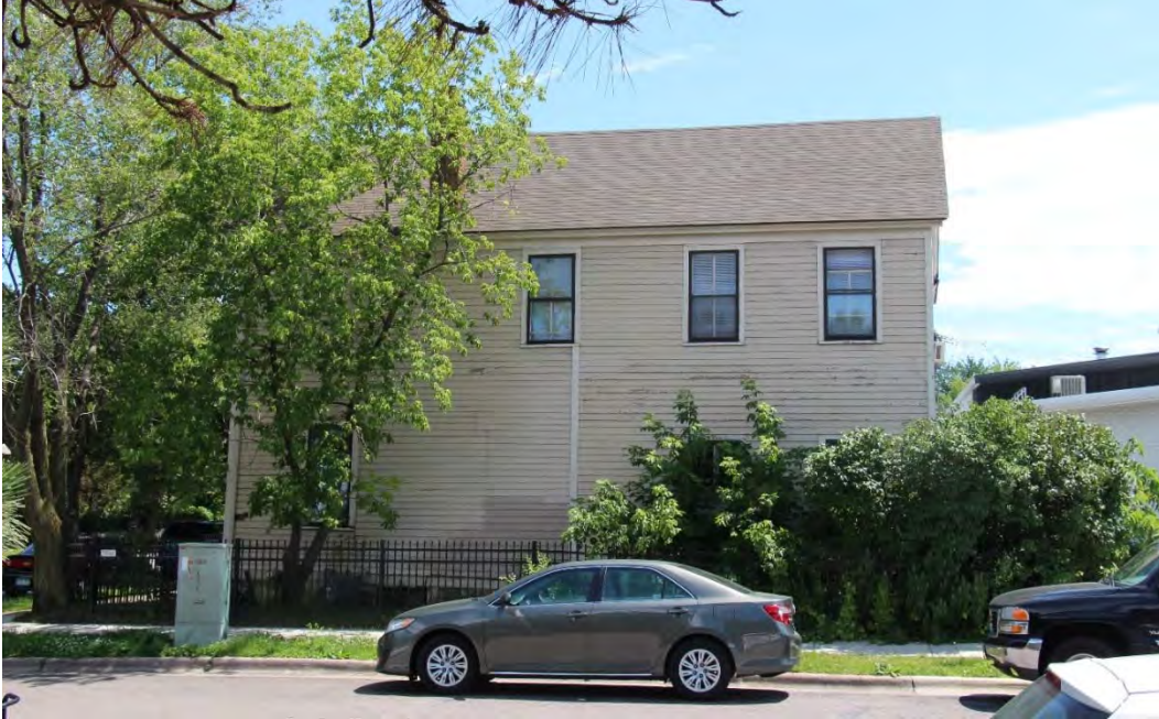
Side (north) elevation, view facing south.
