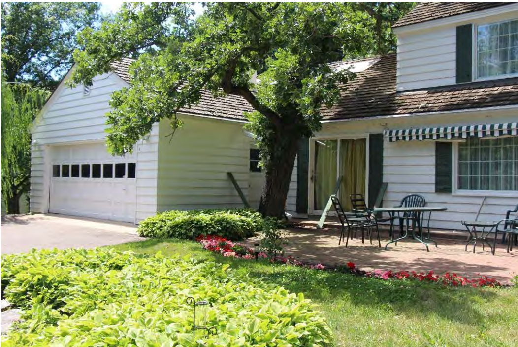
Figure 149. c. 1950 two-car garage attached to the side (south) elevation, view facing southwest.
