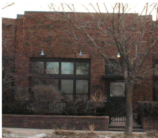
Figure 33. Detail of central bay featuring bank of windows and main entrance.
