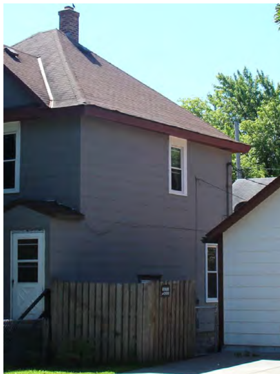
Figure 91. Back (west) elevation, view facing southeast.
