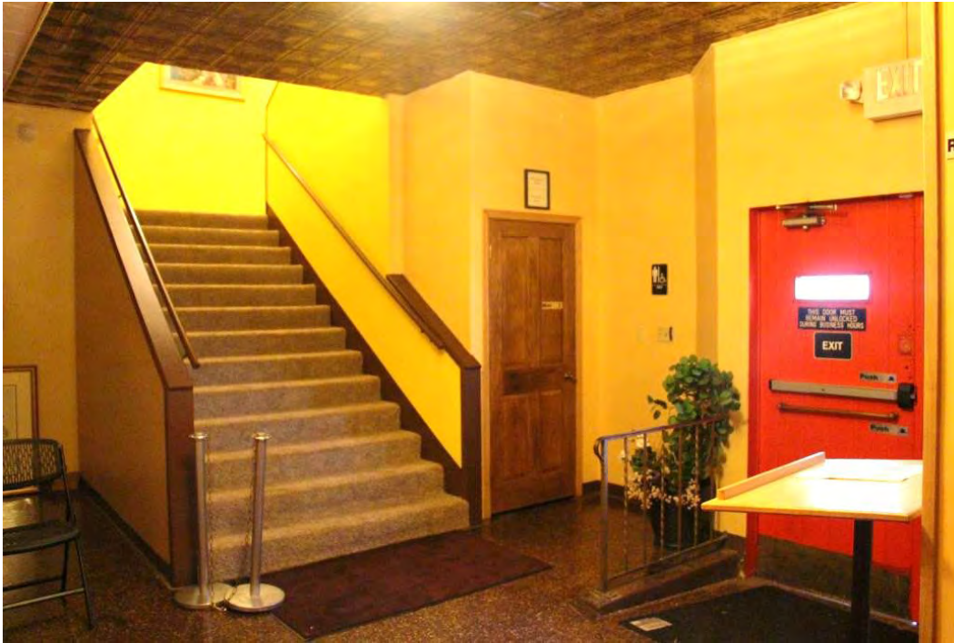
Figure 123. Entry vestibule with the original, but likely modified, staircase.
