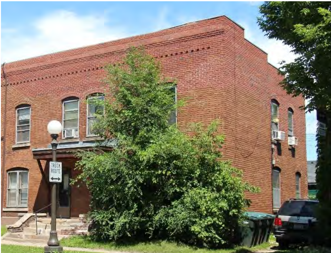
Figure 26. Side (south) elevation visible from Smith Avenue North, view facing northeast.
