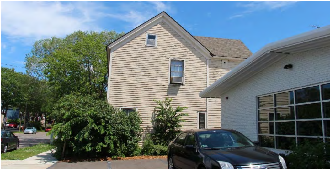
Side (west) elevation, view facing east.
