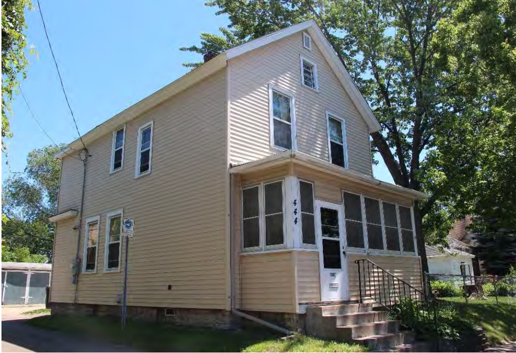
Side (north) elevation and front (west) facade, view facing southeast.
