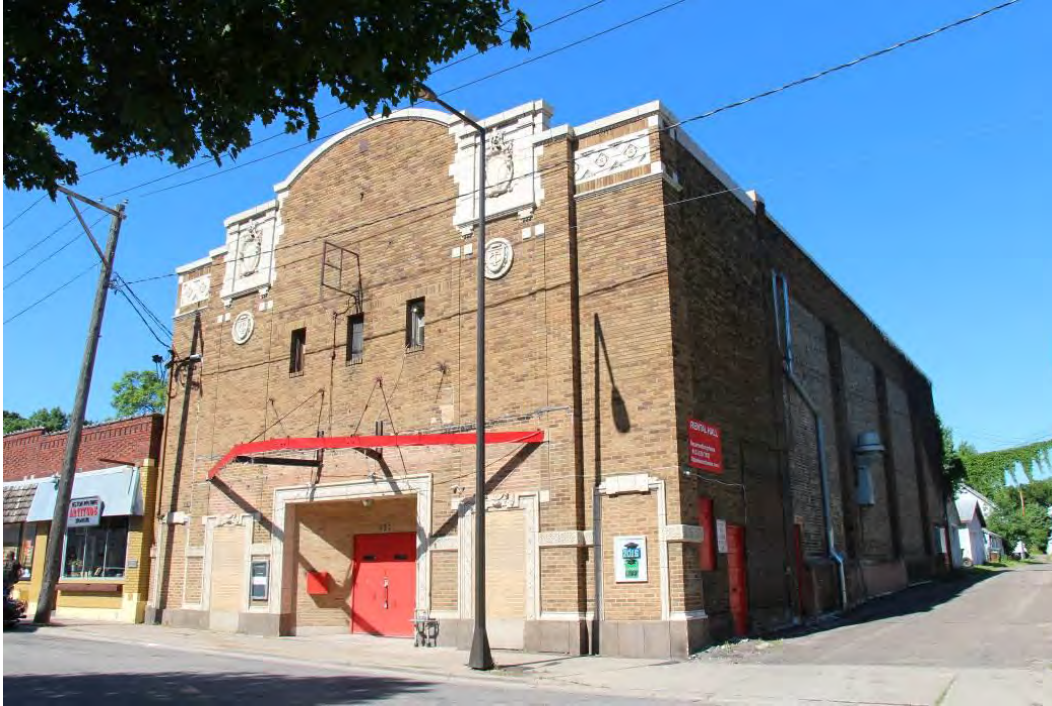
Figure 108. Front (east) facade and side (north) elevation of the Mohawk Theater.
