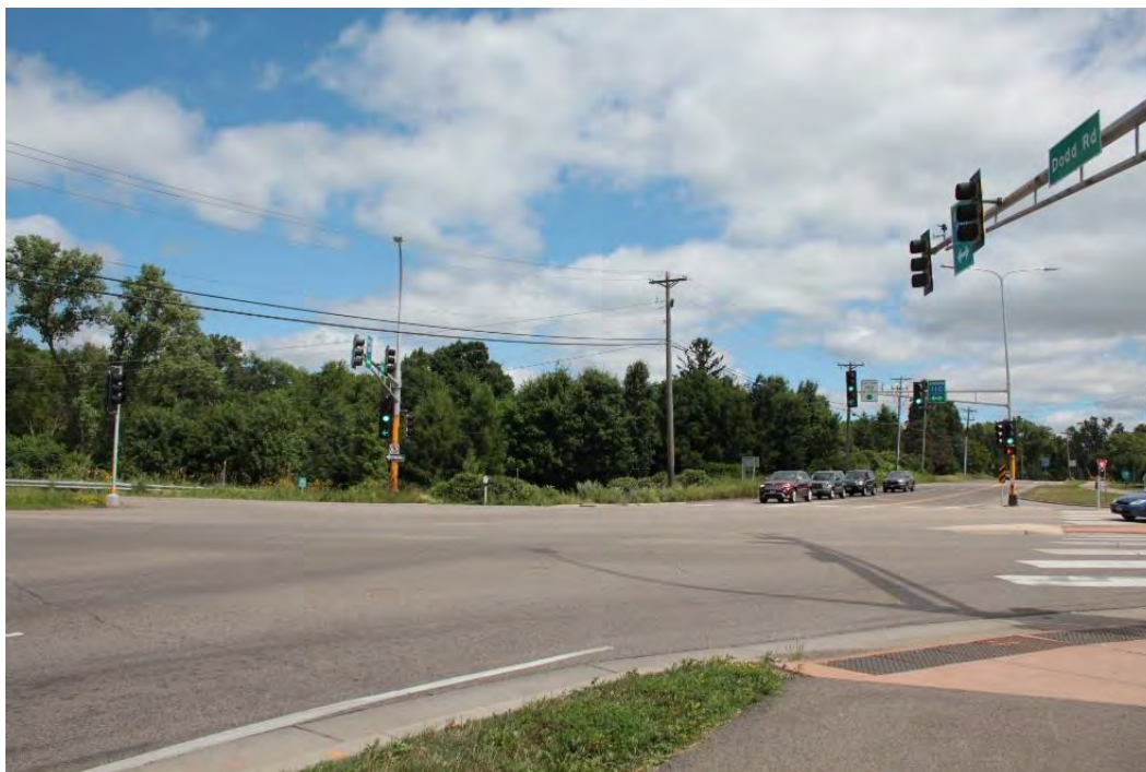
Figure 220. Dodd Road at TH 110 in Mendota Heights, view facing northwest.
