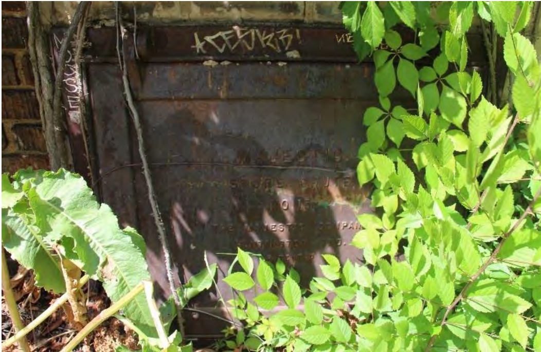
Figure 36. Detail of coal chute on the side (south) elevation.
