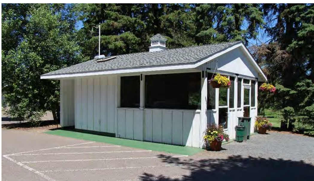
Figure 190. c.1990 rest house, view facing northwest.
