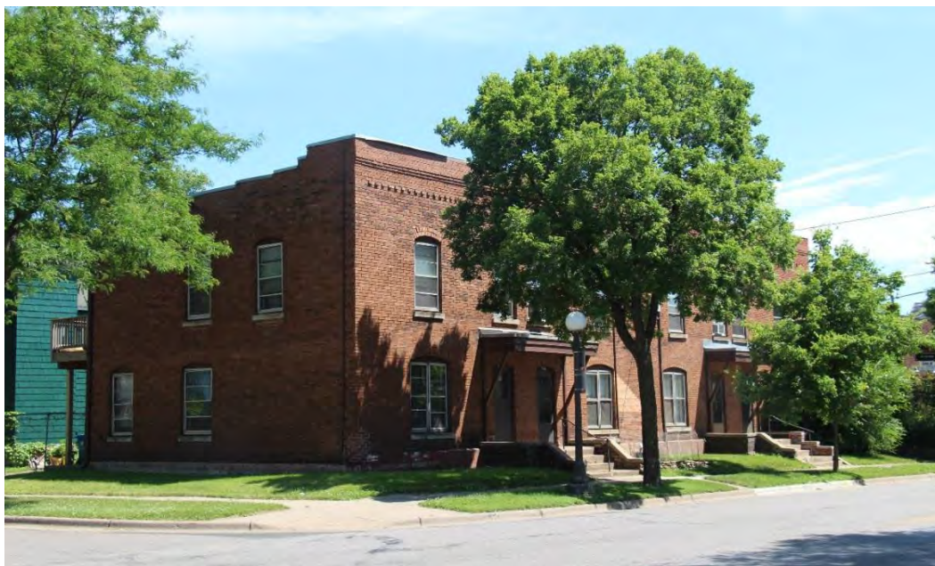
Figure 22. Front (west) facade and side (north) elevation of the Johnson Building, view facing southeast.
