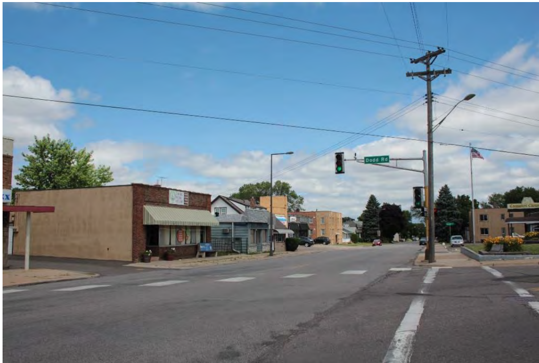
Figure 215. TH 149, intersection of Smith Avenue South and Dodd Road, view facing north.
