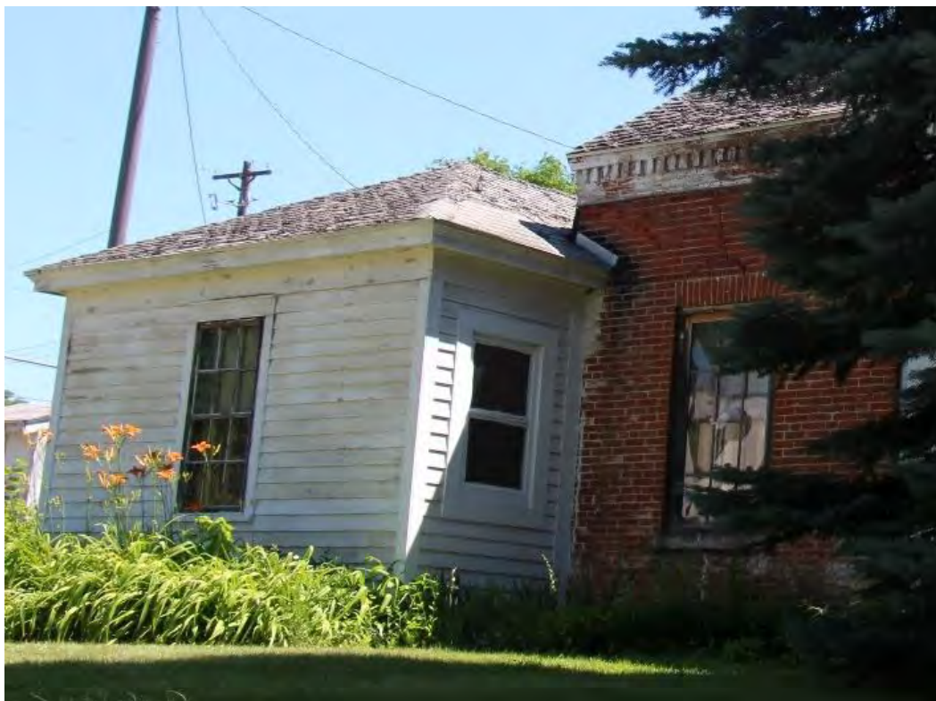
Figure 70. Addition on north elevation, view facing northeast.
