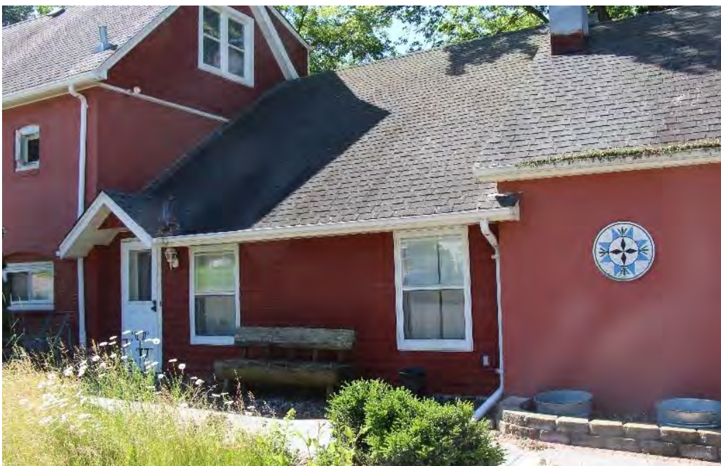
Figure 203. North elevation addition, view facing northeast.
