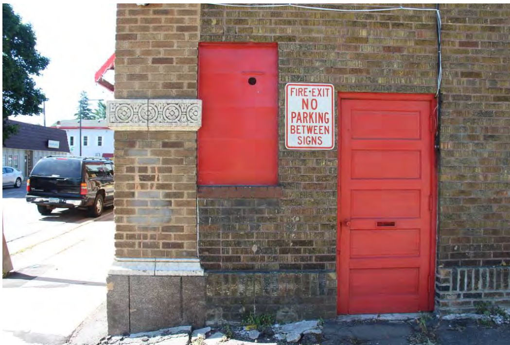
Figure 116. Detail of an original door and covered window on the side (north) elevation.
