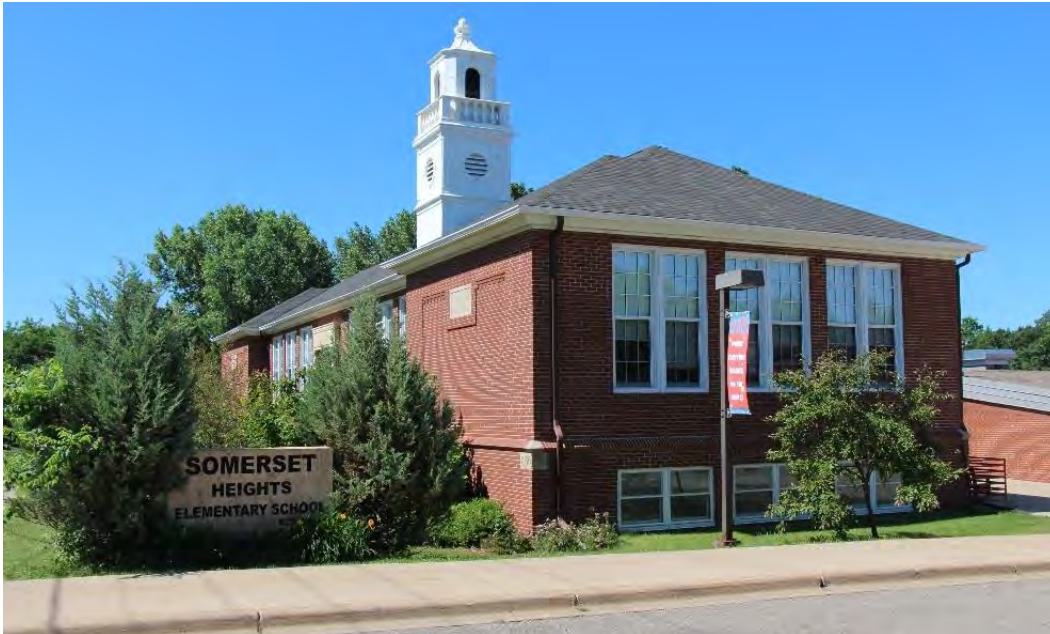
Figure 163. 1936 school building, facing southwest.
