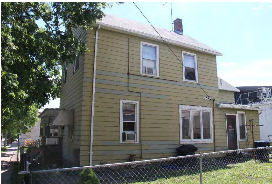
Figure 18. Side (north) elevation, view facing southwest.
