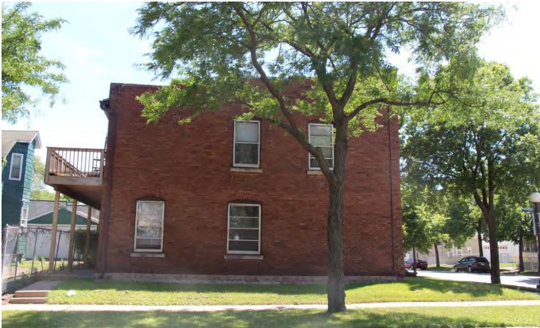
North elevation of the Johnson Building, view facing south.
