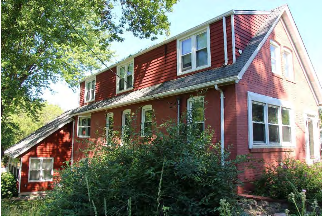
Figure 199. Side (south) elevation and dormer addition, view facing northwest.
