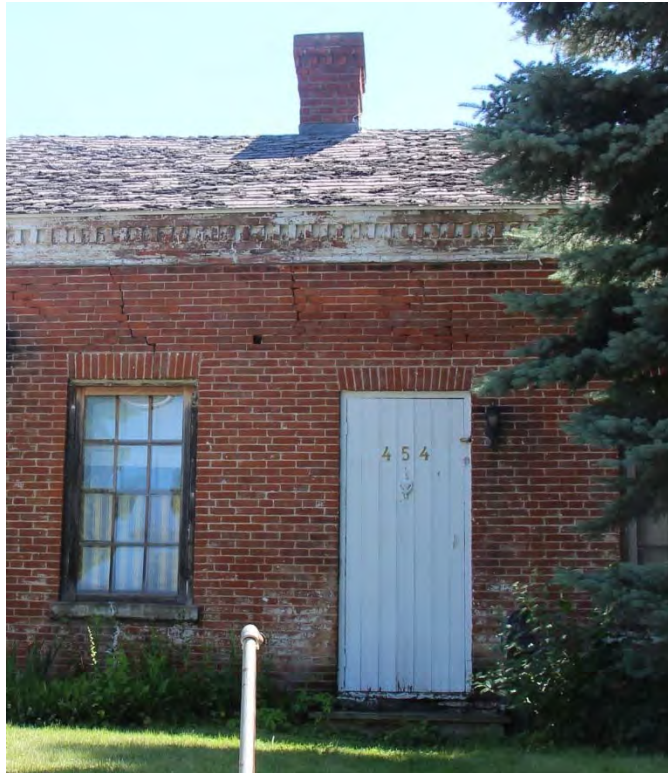
Detail of front (west) facade entrance. Note the dentil detail on the cornice.
