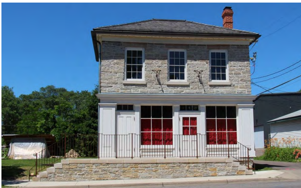
Figure 42. Front (east) facade, view facing west.
