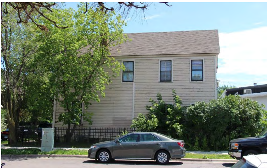
Figure 8. Side (north) elevation, view facing south.
