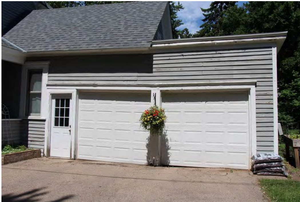
Figure 140. Garage addition at rear (southeast) elevation, view facing northeast.
