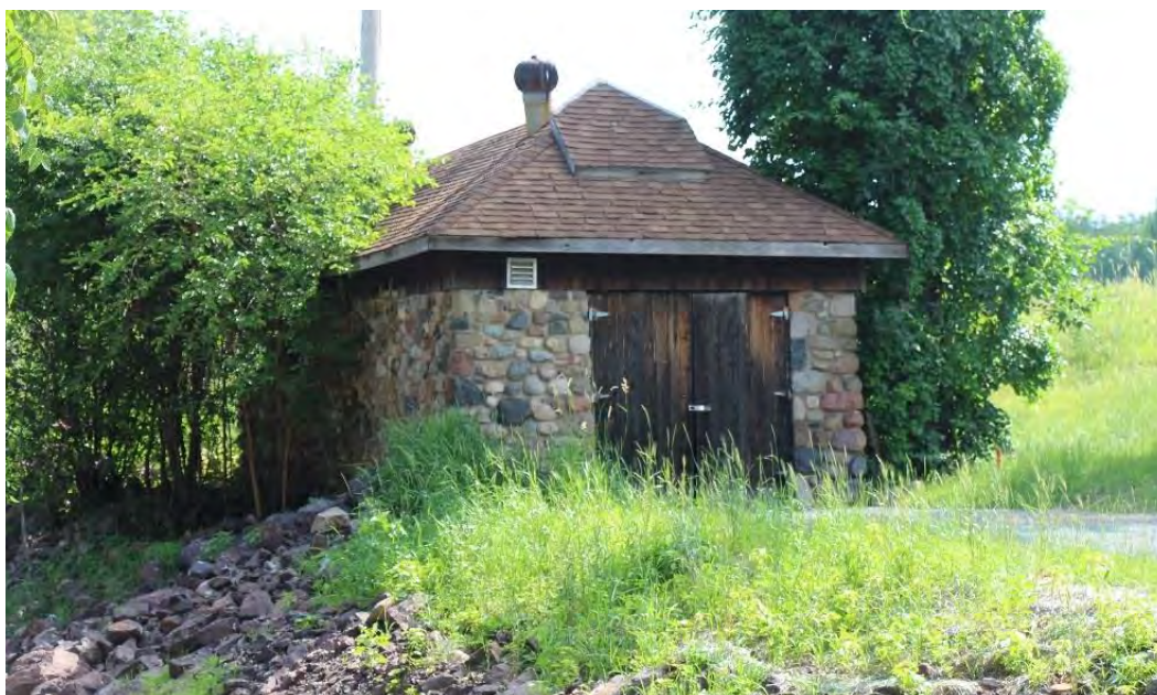
Figure 191. c.1945 pumphouse, view facing northeast.
