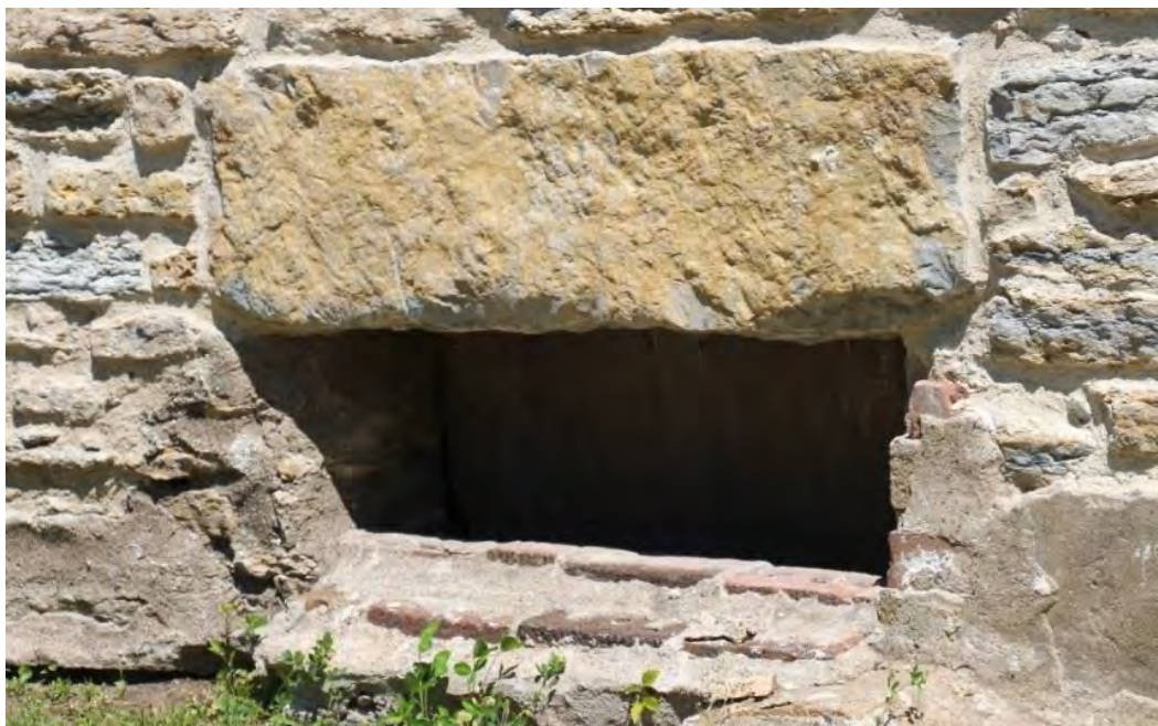
Figure 49. Detail of coal chute on side (south) elevation, view facing north. Note the opening is boarded up from the interior.
