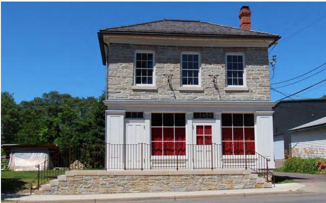
Front (east) facade, view facing west.
