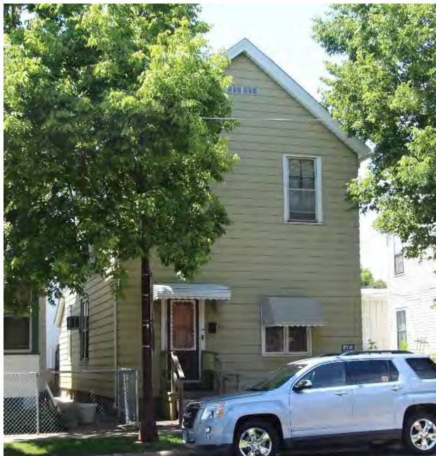
Figure 16. Front (east) facade and side (south) elevation, view facing northwest.
