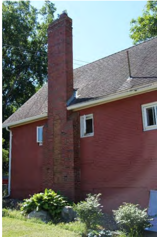
Figure 201. Side (north) elevation chimney, view facing northeast.
