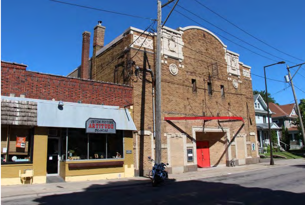
Figure 114. View of side (south) elevation and front (east) facade.
