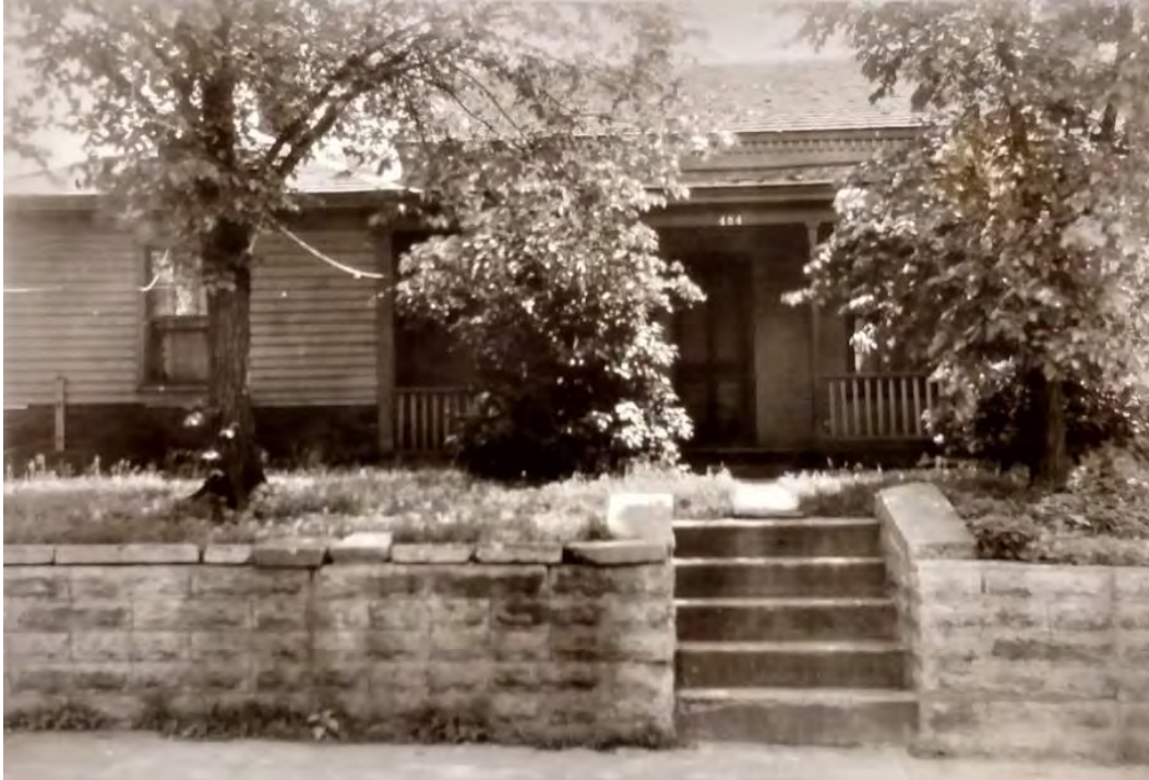
Figure 73. 1936 image of the pre-1900 porch on the front facade of the Adams House. 137
