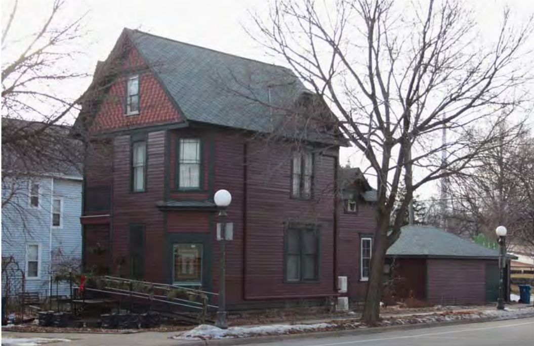
Front (north) facade and side (west) elevation, view facing southeast.
