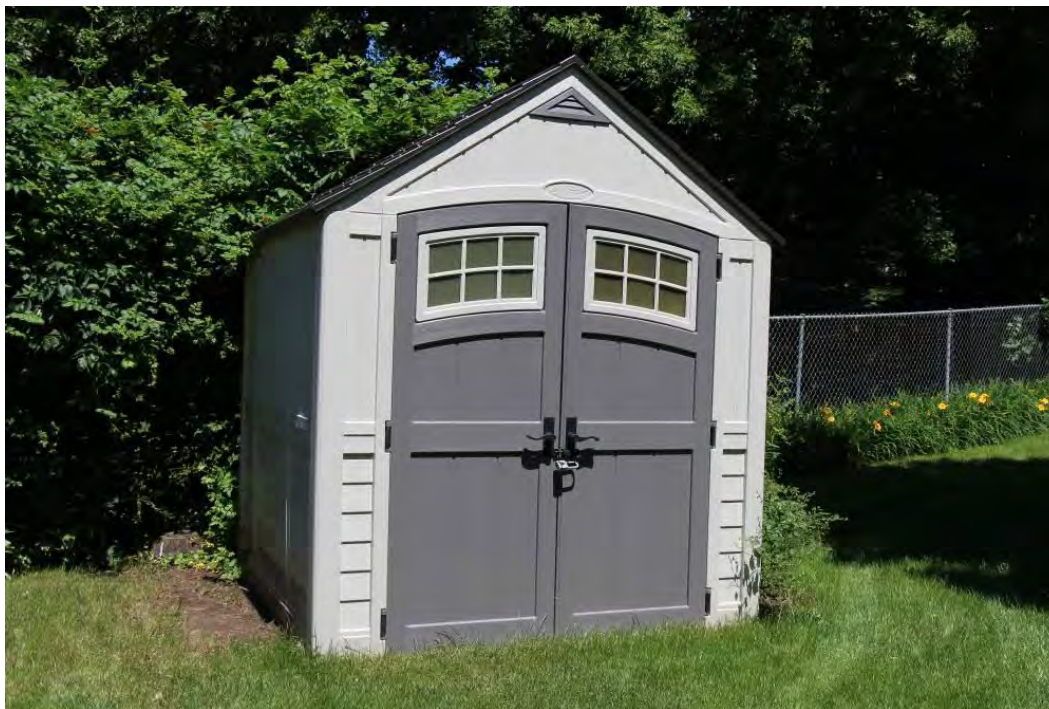
Figure 142. Modern shed, view facing northeast.
