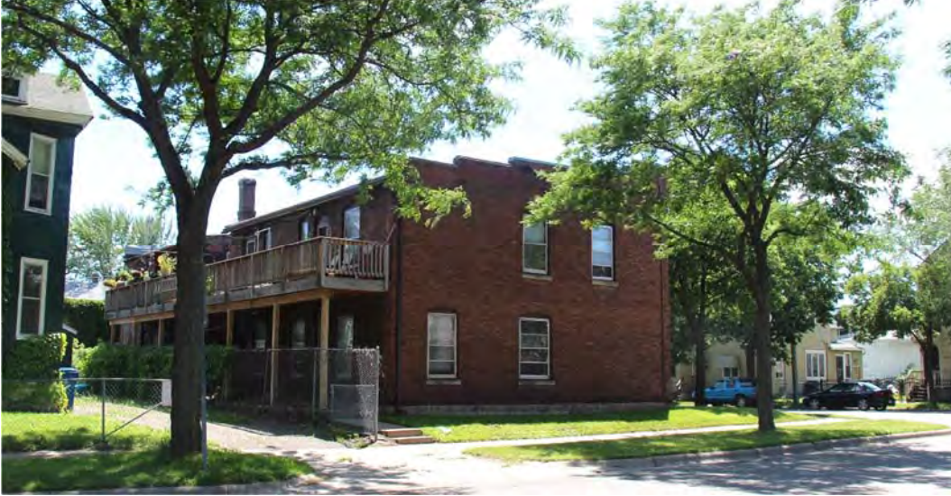
Rear (east) elevation of the Johnson Building, view facing southwest.
