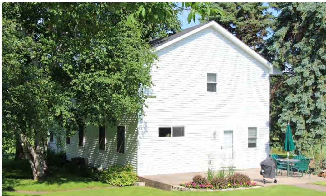
Figure 188. c.1880 building, view facing northwest.
