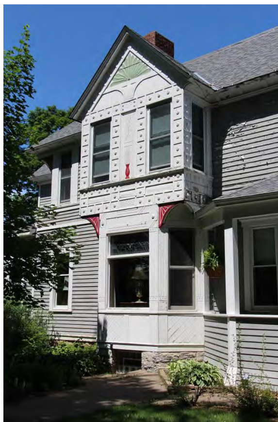
Figure 138. Detail of two-story bay window, view facing northwest.
