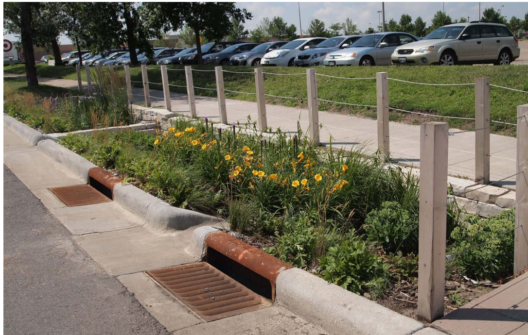
Figure 1.3 Green Infrastructure on the Green Line Source : Capitol Region Watershed District
