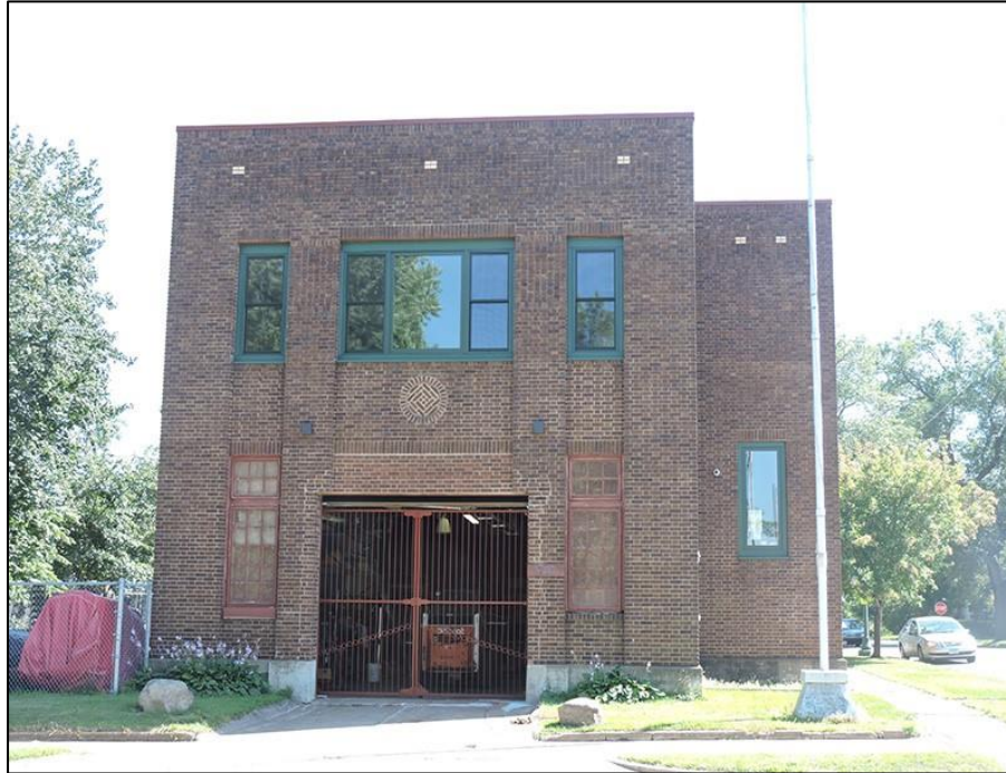
Figure 24. Engine House No. 24 at 1720 East Seventh Street, 2016
