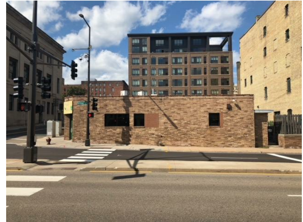
VIEW 3 - FACING NORTHWEST
