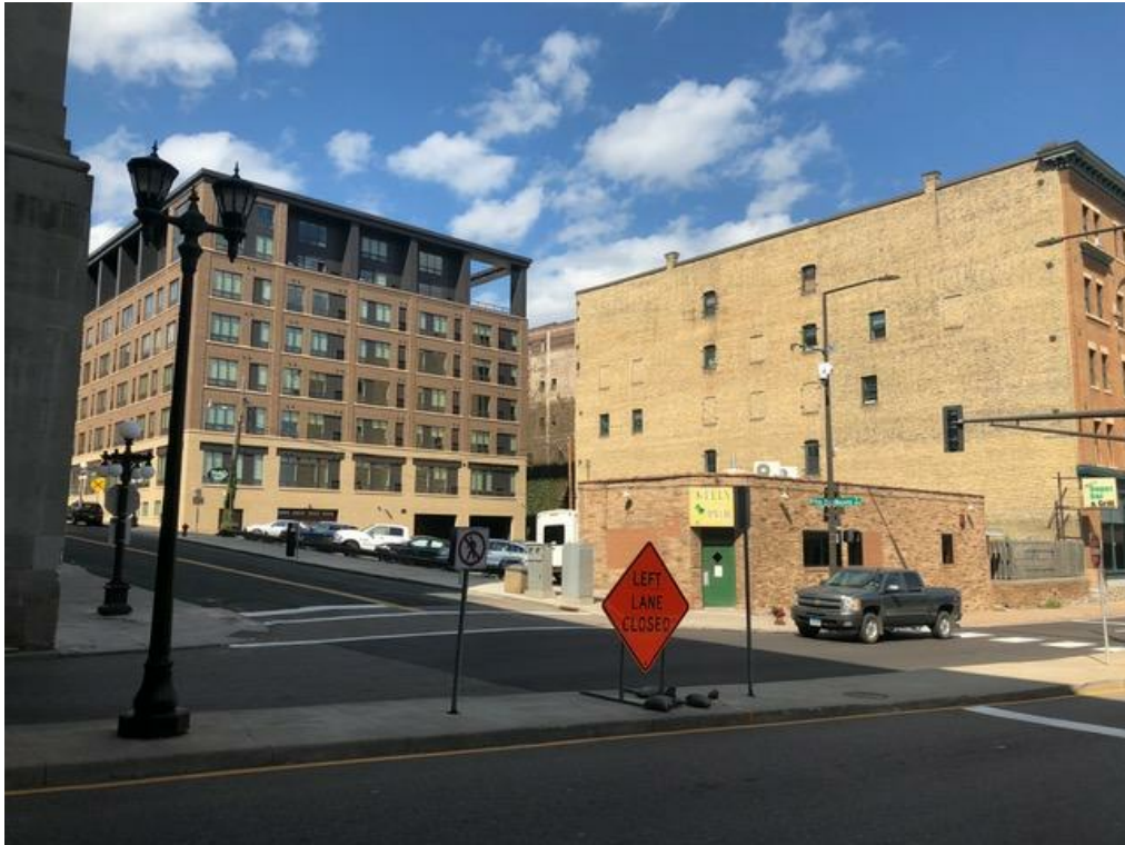
VIEW 1 - FACING NORTH
