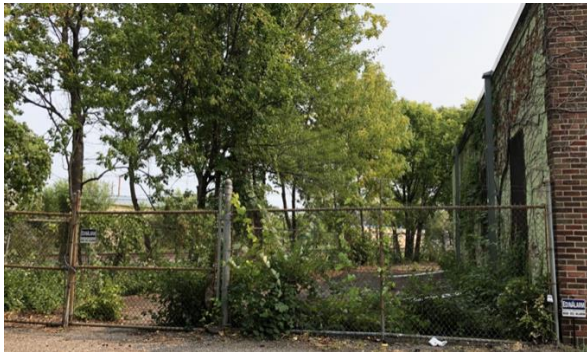
Rear of building at 1725 Carroll Avenue
