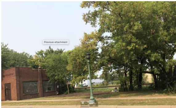
Eastern end of building at 1725 Carroll
