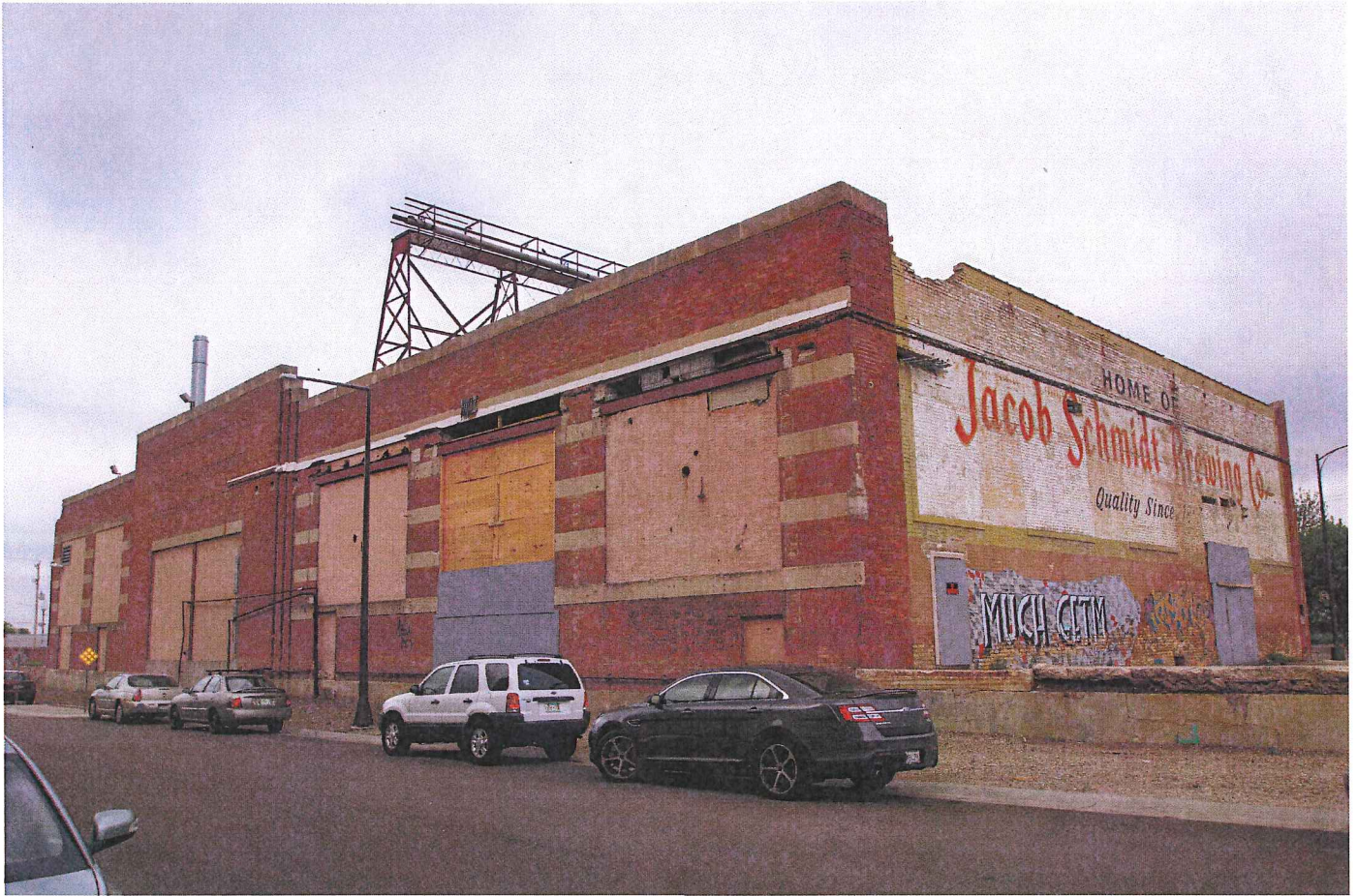
View from West 7th Street and Weber Street
