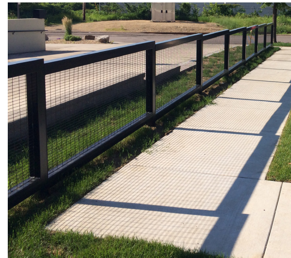
Parking Lot Fence
