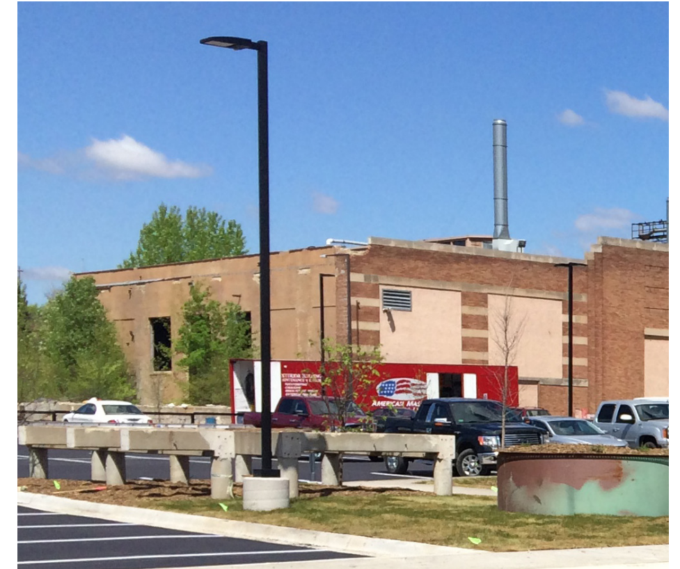
Parking Lot Light
